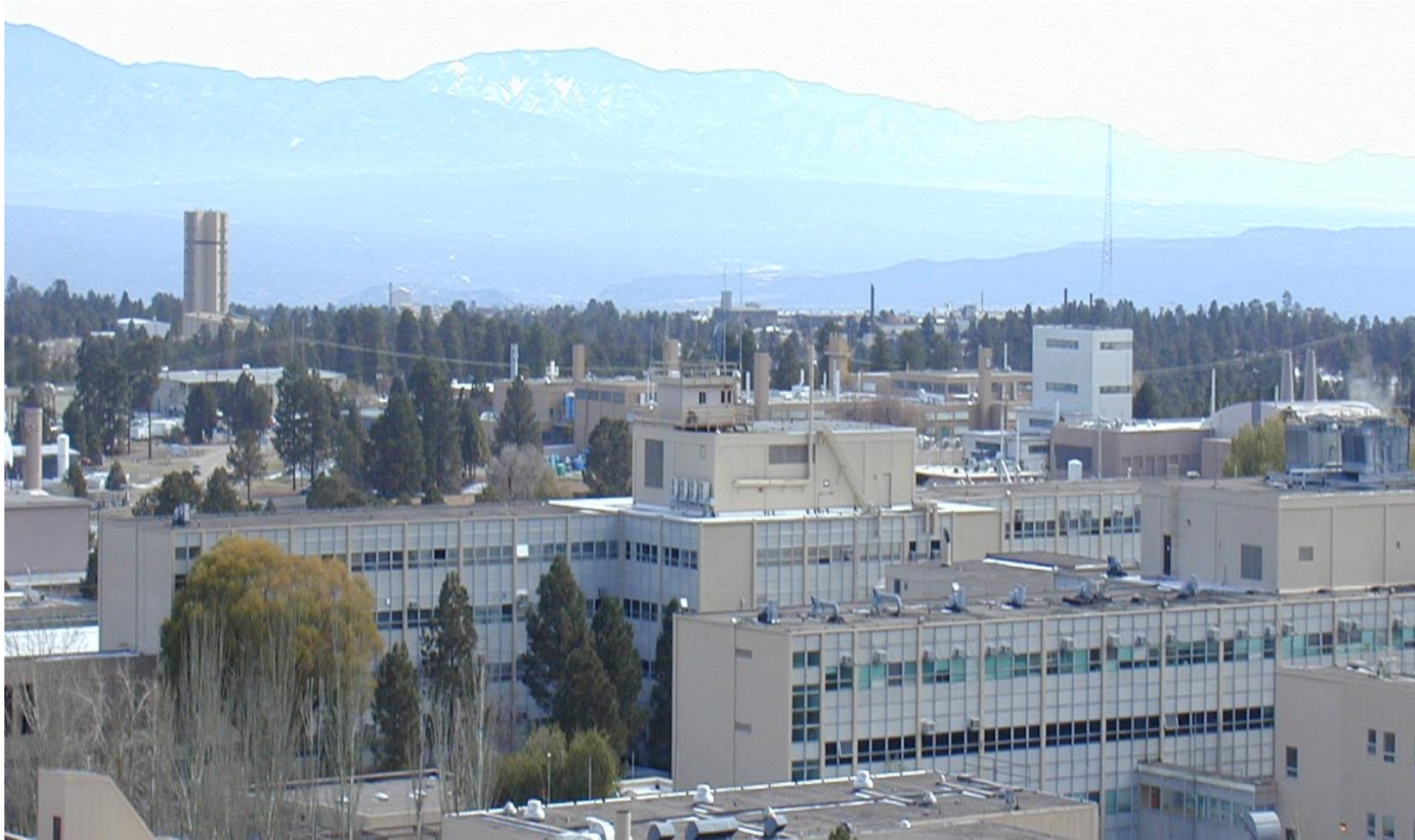
Figure 3a. Existing Administration Building 3-43 (looking mostly east).
