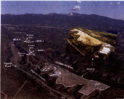
Technical Area 54 Material Disposal Area L Aerial
