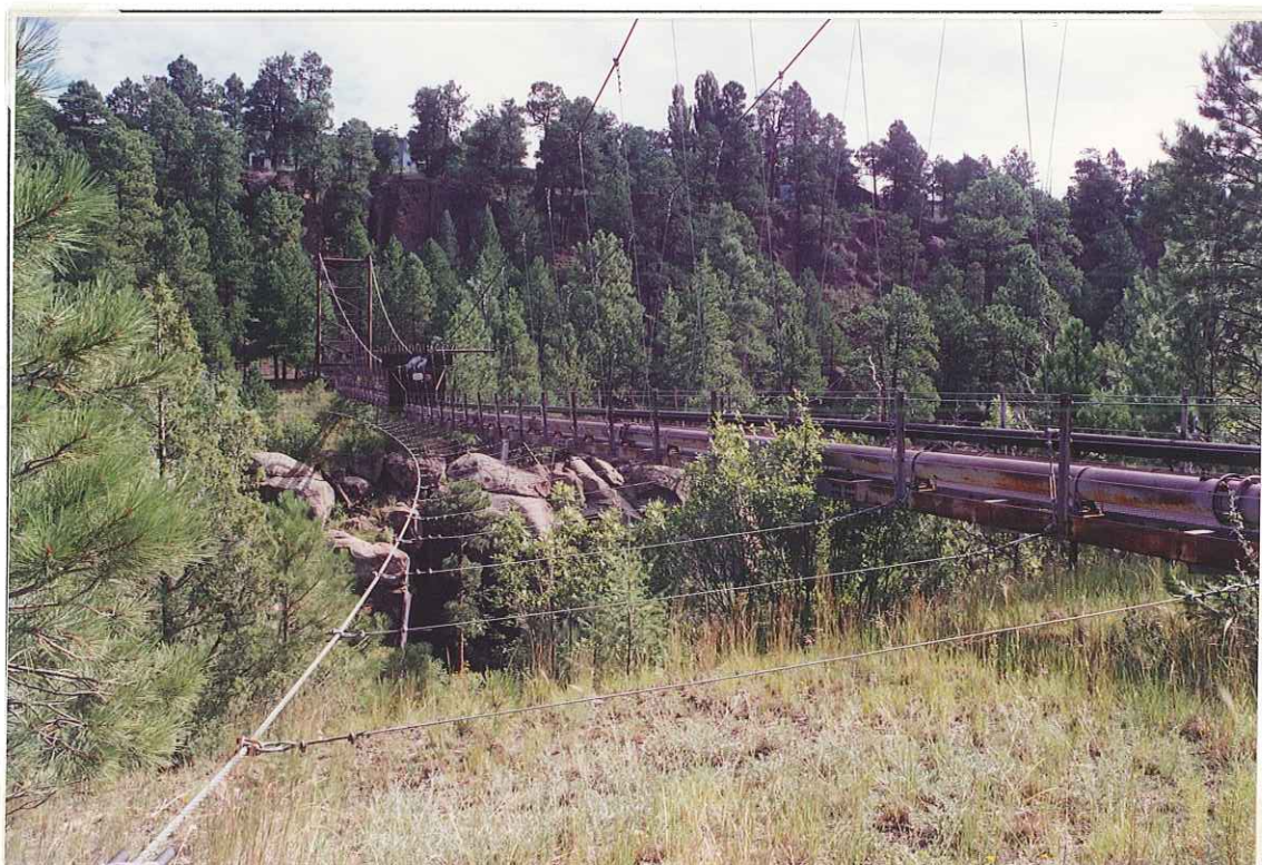
Little Peggy Sue Bridge, view from south end, dir. ~NNE
