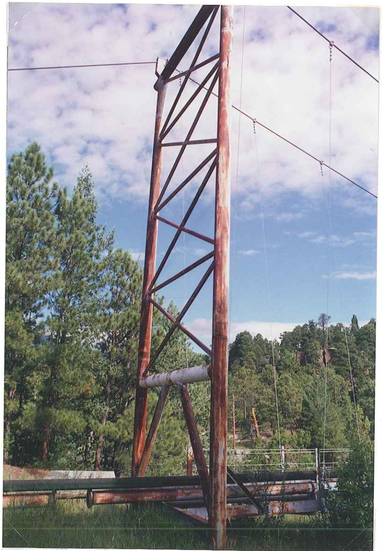
Little Peggy Sue Bridge, south tower, dir. ~W
