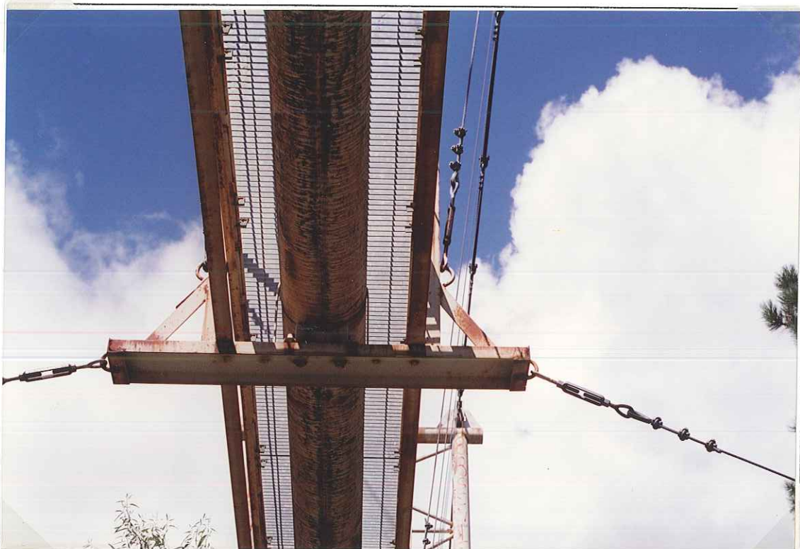
Peggy Sue Bridge (west end), view of pipeline, dir. ~W
