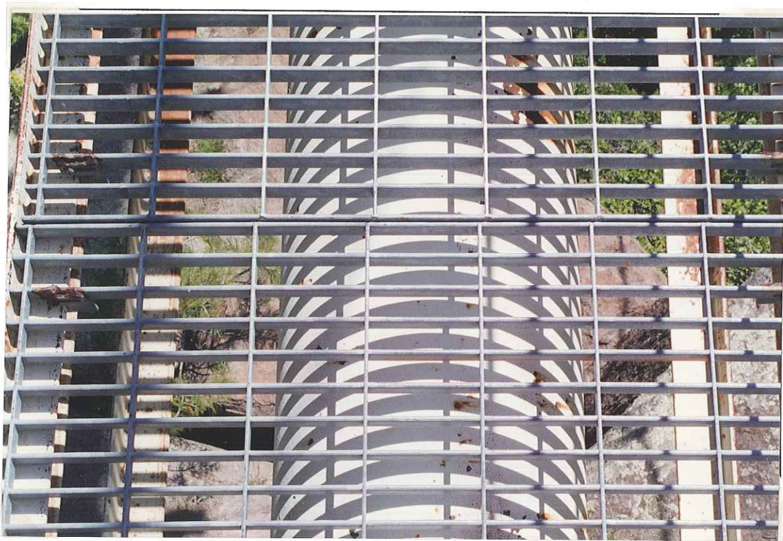
Peggy Sue Bridge, detail of decking and pipe, dir. ~down & east
