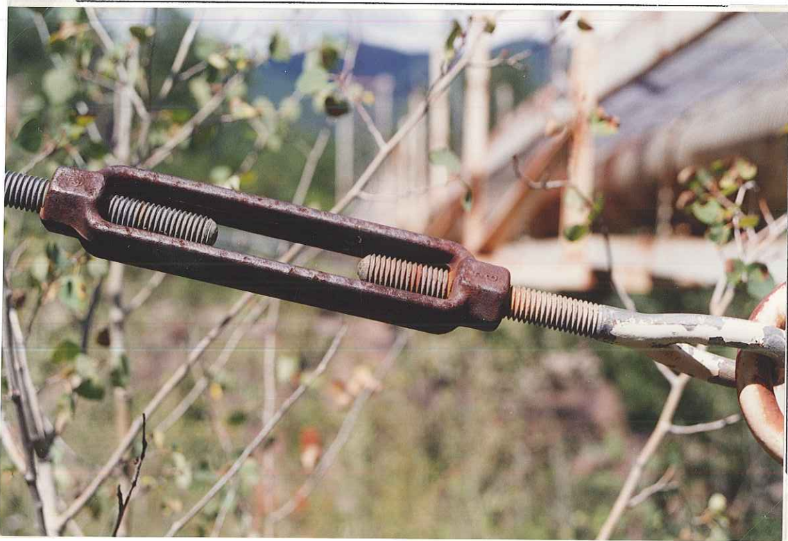
Peggy Sue Bridge (east end), cable connection detail, dir. ~W
