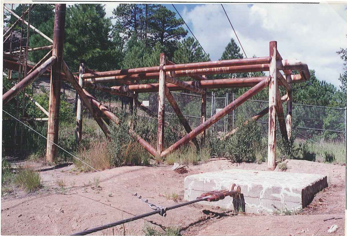
Peggy Sue Bridge (west end), gas piping, dir. ~W
