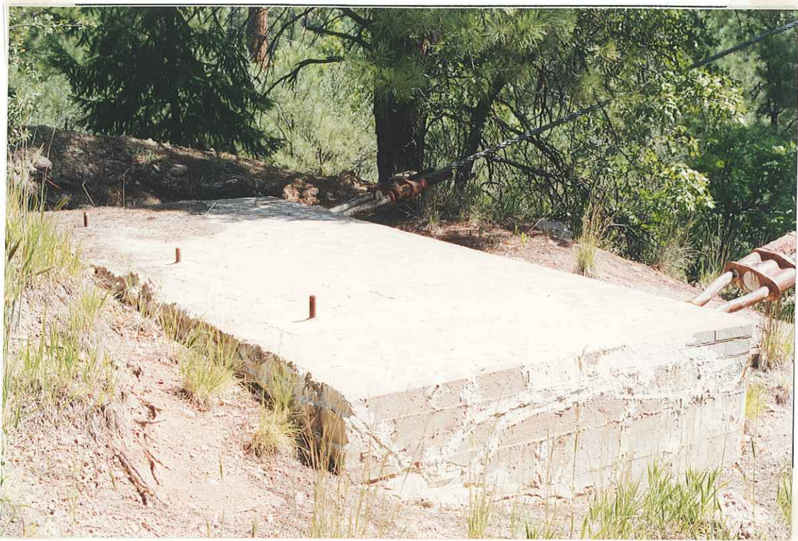
Peggy Sue Bridge (west end), western-most concrete anchor, dir. ~NNE
