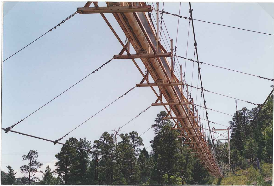
Peggy Sue Bridge (west end), view of underside, dir. ~E
