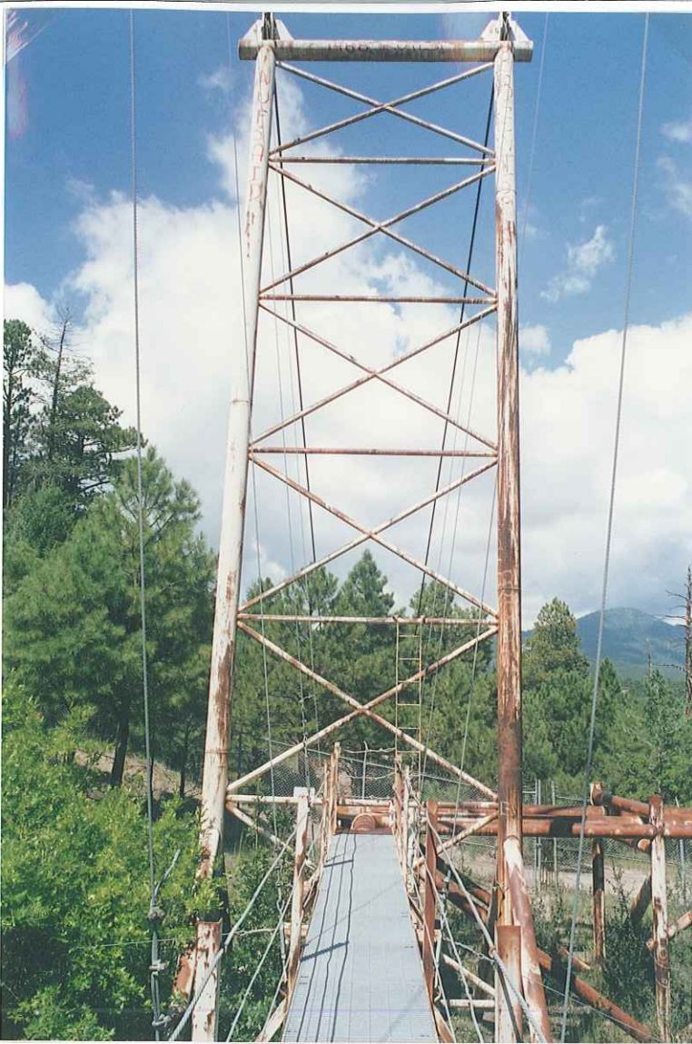
Peggy Sue Bridge, west tower, dir. ~W
