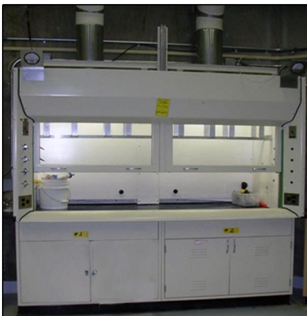
Figure 2.9-1. Example of a laboratory fume hood at LANL
