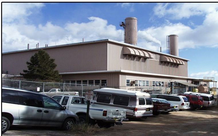
Figure 2.1-1. TA-3 power plant
