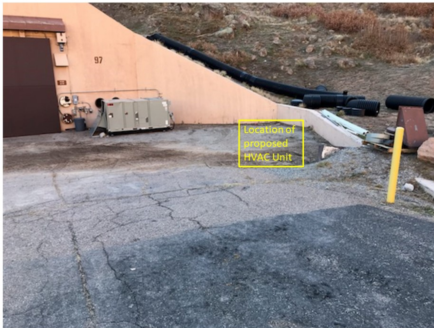
Photo 1. Proposed location of the HVAC unit on a paved area north of building 39-0097.
