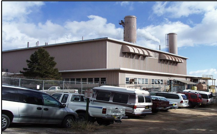
Figure 2.1-1. TA-3 power plant
