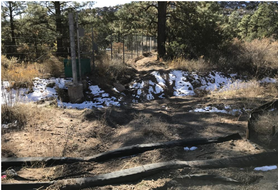
Photo 8. Approximate location of pre-fabricated bridge crossing Sandia Canyon, facing south.
