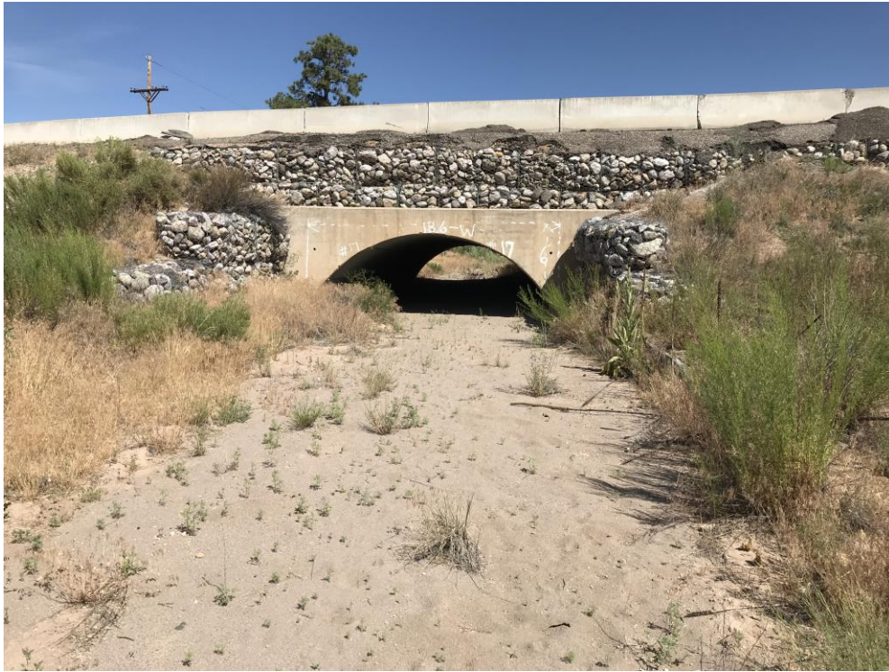
Photo 3. View of multi-plate arch culvert under East Jemez Road, facing north.
