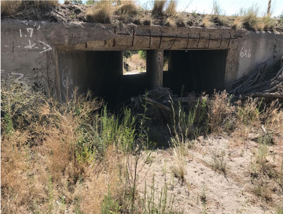
Photo 5. View of double box culvert under State Route 4, facing east.
