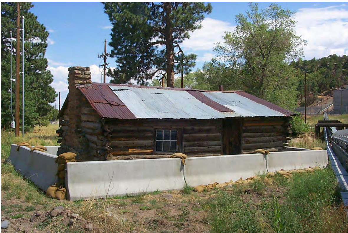
Figure 23.3 The Pond Cabin was enclosed to protect it from possible flash flooding after the Cerro Grande fire
