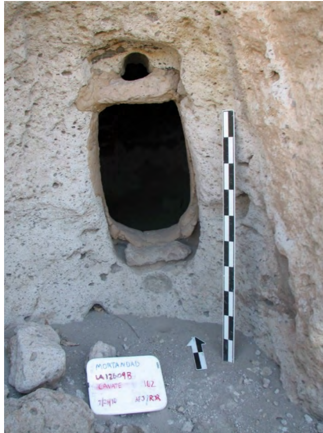
Figure 21.2 High-priority cavate; note intact lintel, ventilation hole, and plaster (2009)
