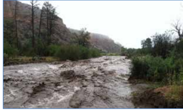
Figure 2-15 Flooding on Laboratory property
