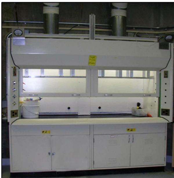
Figure 2.9-1. Example of a laboratory fume hood at LANL.
