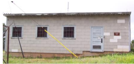
TA-14-6 (Shop and Darkroom Building)
