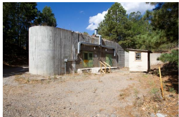
TA-8-2 (Shop and Storage Building, left) and TA-8-172 (Portable Guard Shack, right)
