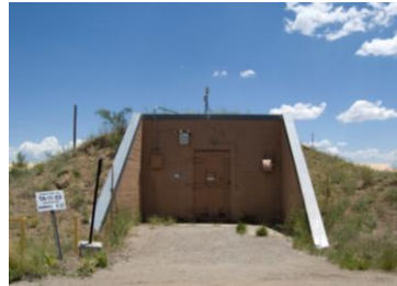
TA-11-1 (Control Building)
