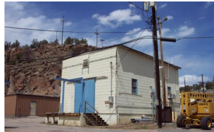
TA-18-1 (Slotin Building)
