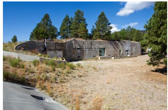
TA-8-1 (Laboratory and Shop Building, center) and TA-8-3 (Laboratory Building, left)
