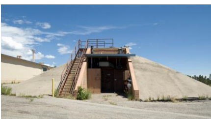
TA-11-3 (Cloud Chamber Building)
