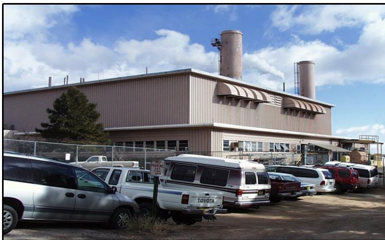
Figure 2.1-1. TA-3 power plant.
