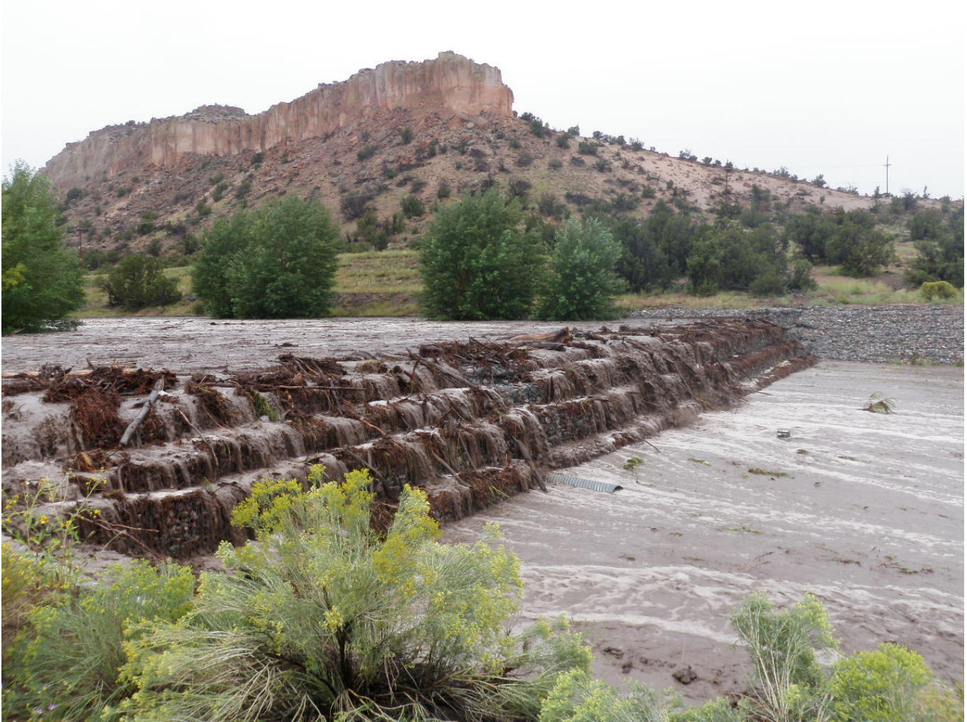
Los Alamos Canyon weir performing as designed to retain as much sediment as possible during a major storm event.
