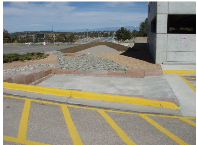
Storm water controls are a major part of the runoff management plan at Technical Area 03.
