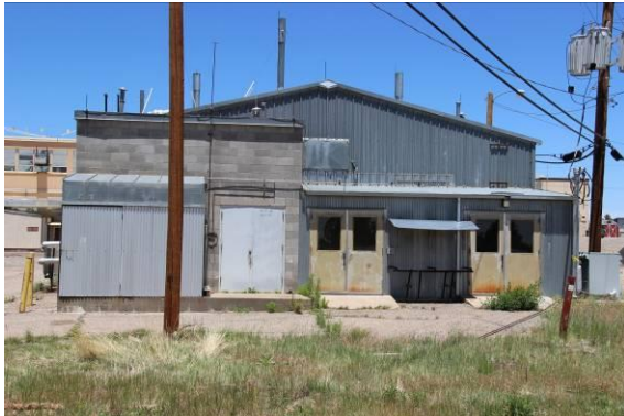
View of south side
