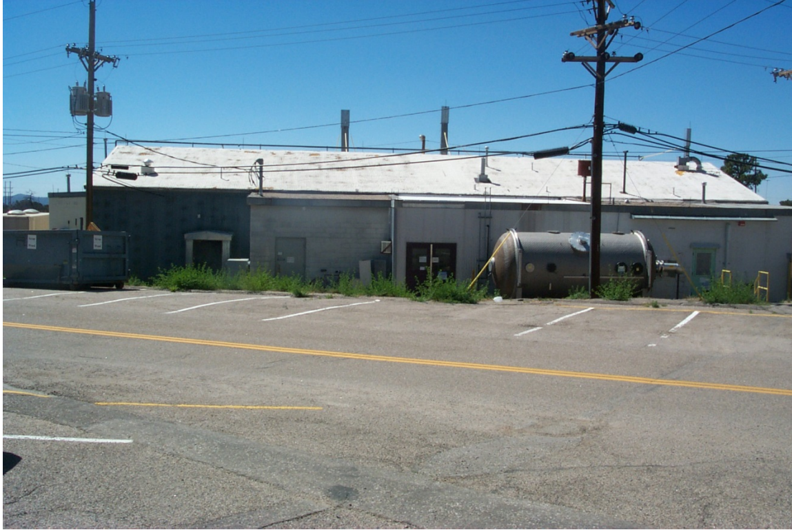
TA-46-41 Northwest side
