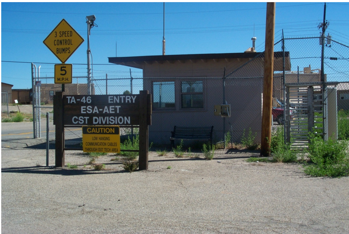
TA-46-2 Southwest side
