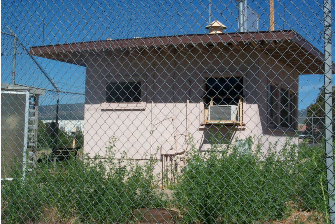
TA-46-2 Southeast side
