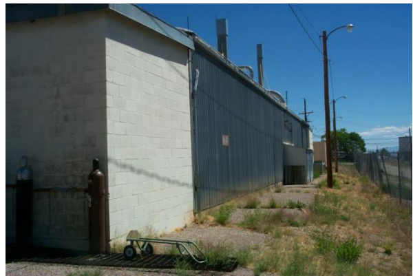
Oblique view of south side to the east
