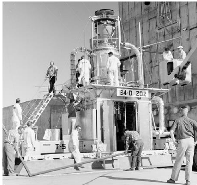
The Project Rover nuclear reactor (photo at left) was designed to power rockets. Compressed hydrogen in the spheres at the top flowed through the reactor core (center) and formed a jet as it exited the nozzle at the bottom (LANL 1983). The Laboratory's Kiwi B-4D reactor (photo at right) being readied for a "hot run" in May 1964 (LASL 1964).
