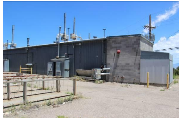
View of west and south sides
