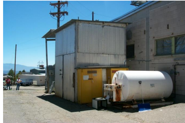
Oblique view of north and west sides
