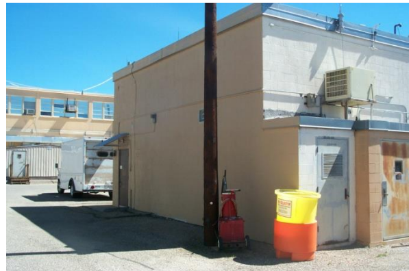
Oblique view of west side
