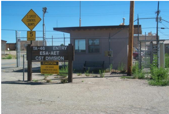
View of south side
