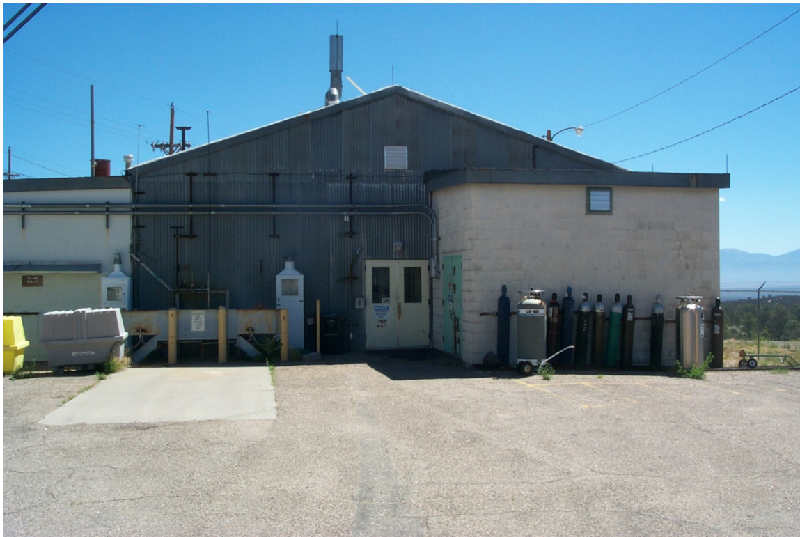
TA-46-41 Southwest side
