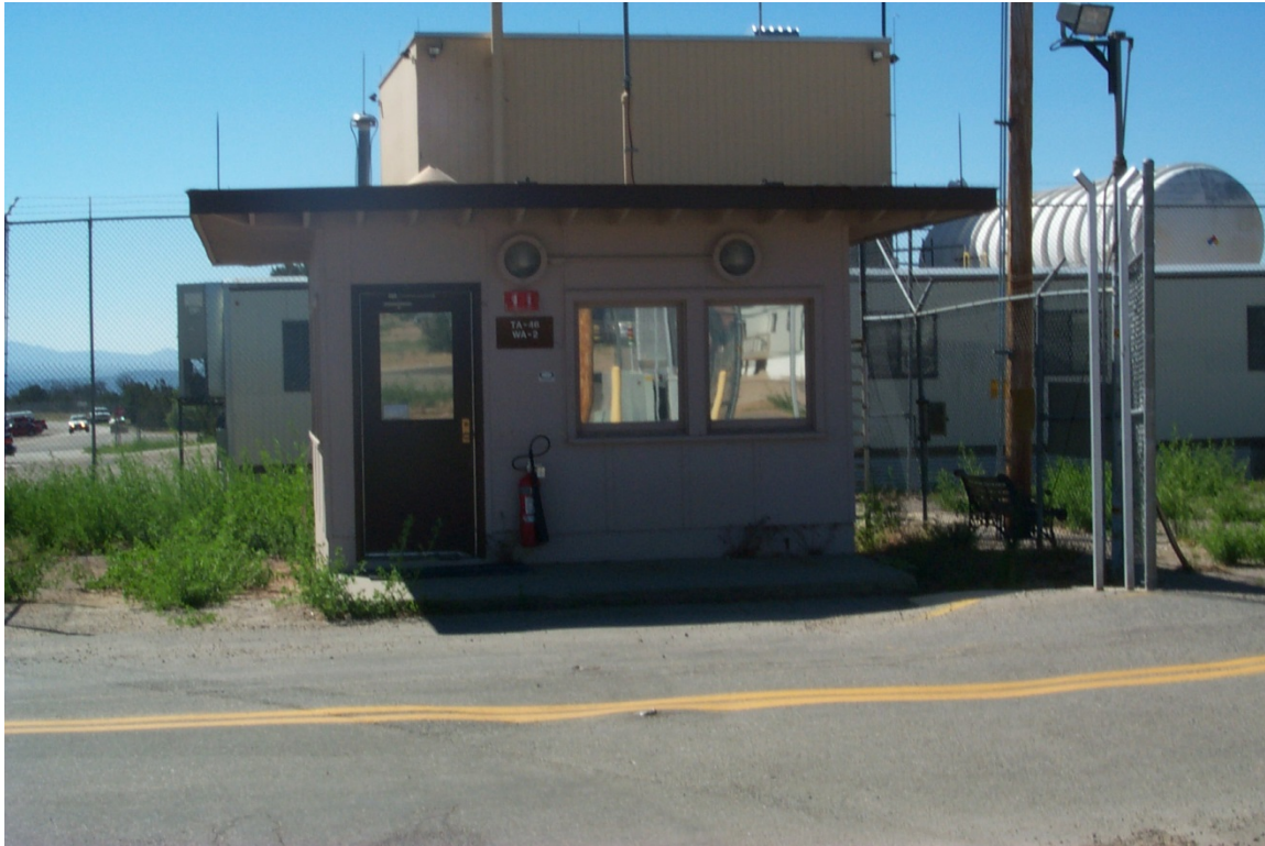
TA-46-2 Northwest Side
