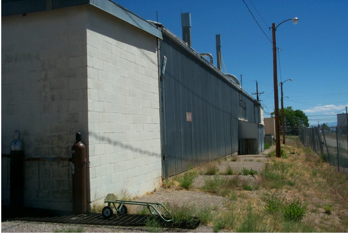
TA-46-41 Southeast side
