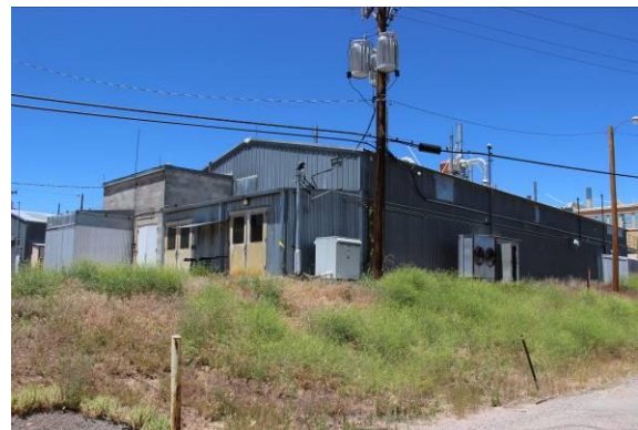
View of south and east side
