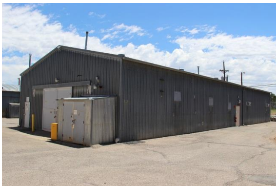
View of north and west side
