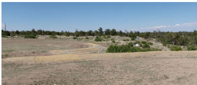
F-SMA-2, Earthen Berm, F00103010015 (photo ID 23503-5)
