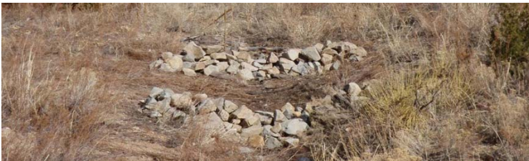
PT-SMA-1.7, Rock Check Dam, I00306010010 (photo ID 12975-1r)
