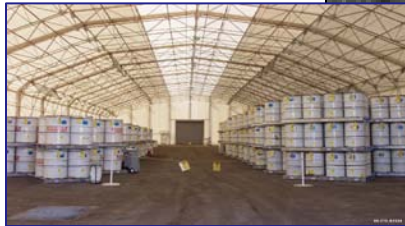
Storage (Area G)
