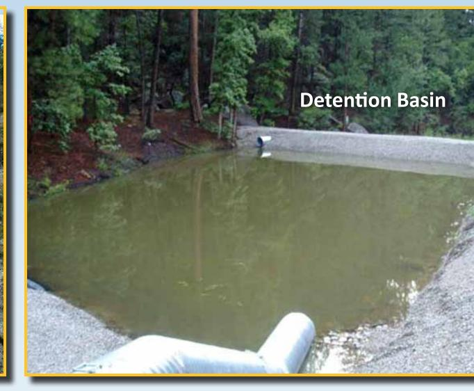
Detention basins manage storm water runoff by temporarily storing water after a storm which limits downstream erosion and controls some pollutants such as suspended solids.
