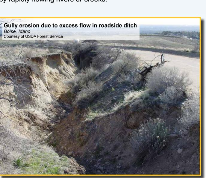
that it cuts a well defined channel. These channels can be as small as one centimeter wide or as large as several meters.
