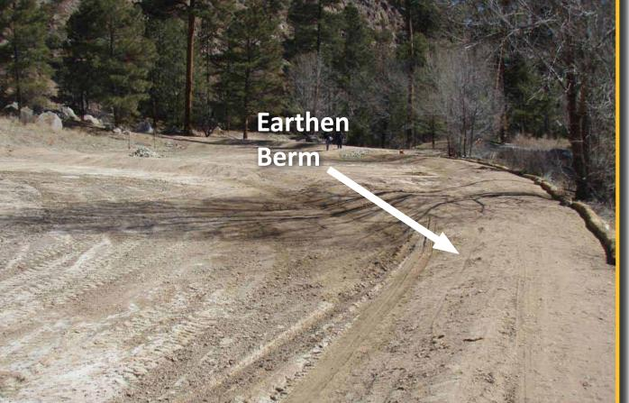
Earthen berms capture sediment, intercept flow, and manage runoff.
