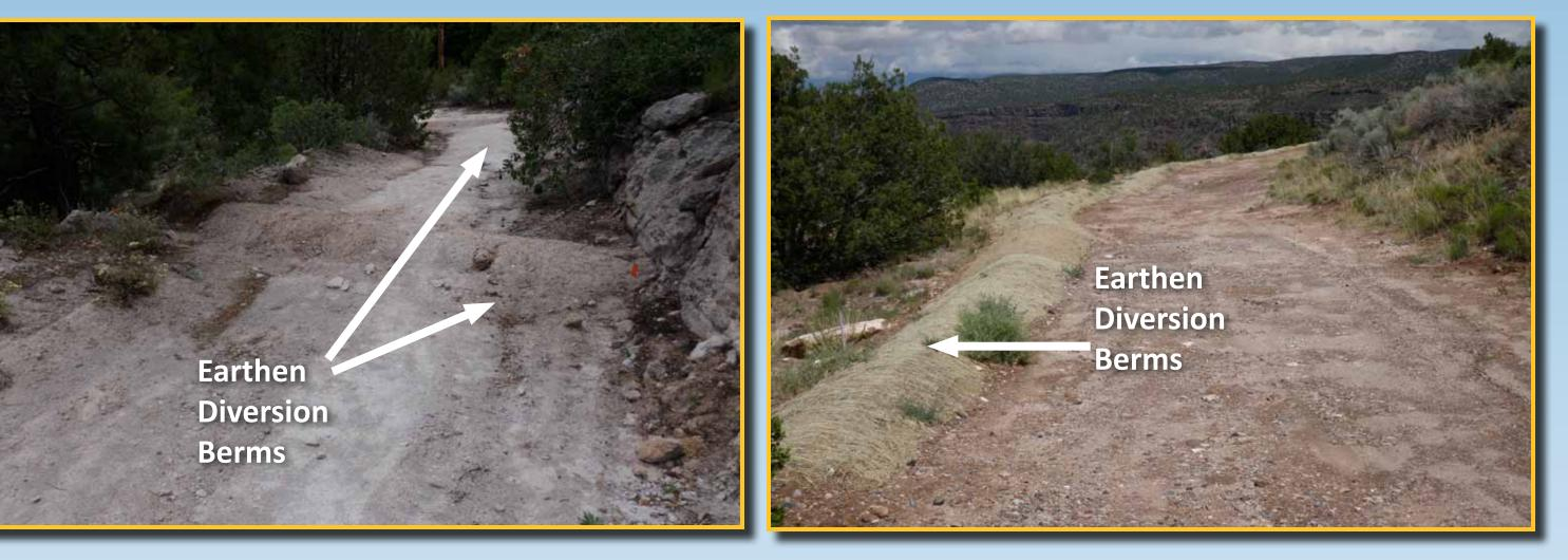
Earthen diversion berms can reduce or control run-on generated from decommissioned roads.
