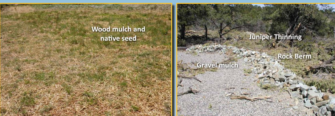
Wood mulch is an engineered erosion control material used to prevent wind erosion, rill formation, and promote revegetation.
