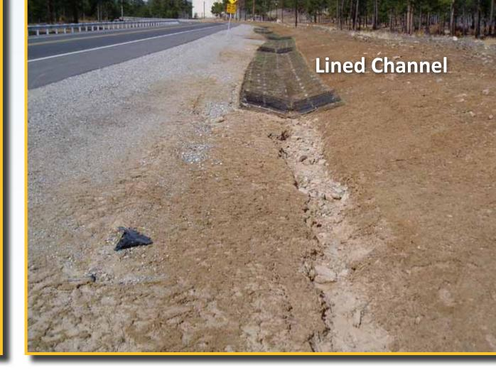
Silt fence failure due to improper maintenance BMP should extend length of eroded channel
