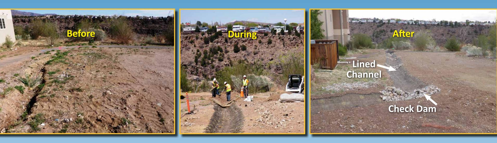
Lined channels can convey run-on across a site while minimizing the potential for erosion.
