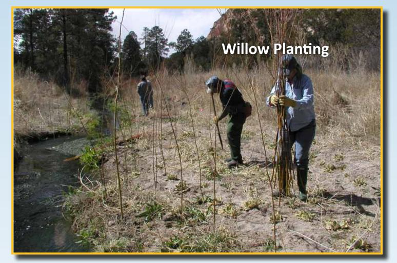
Willow planting is a bioengineering erosion control practice which provides mechanical streambank stabilization.
