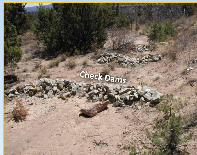
Rock check dams reduce the velocity of concentrated storn water flows and are an effective aid in trapping sediment particles by virtue of the ability to pond runoff.
