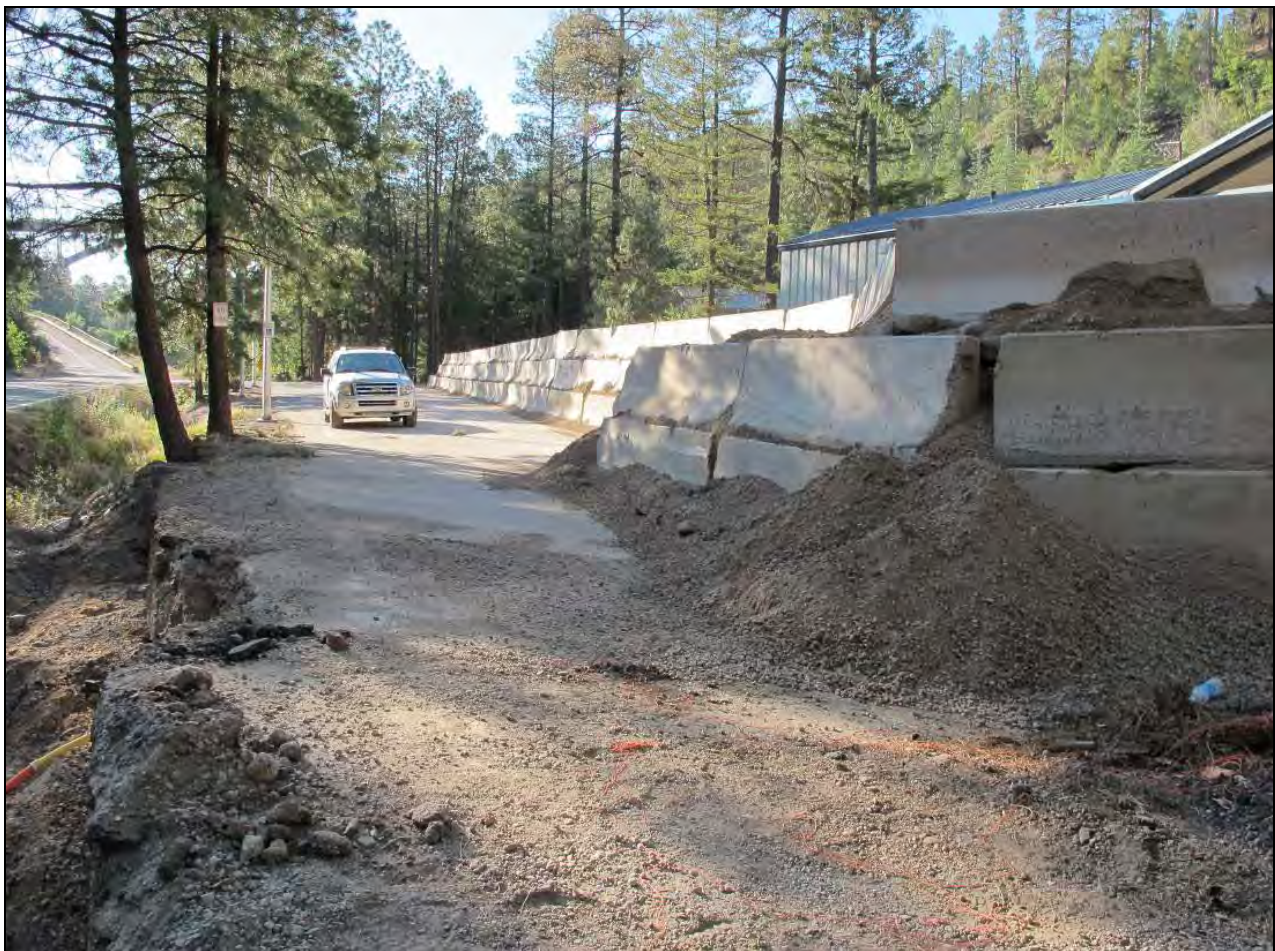
Photograph 14. Armoring at the Los Alamos County Ice Rink.
