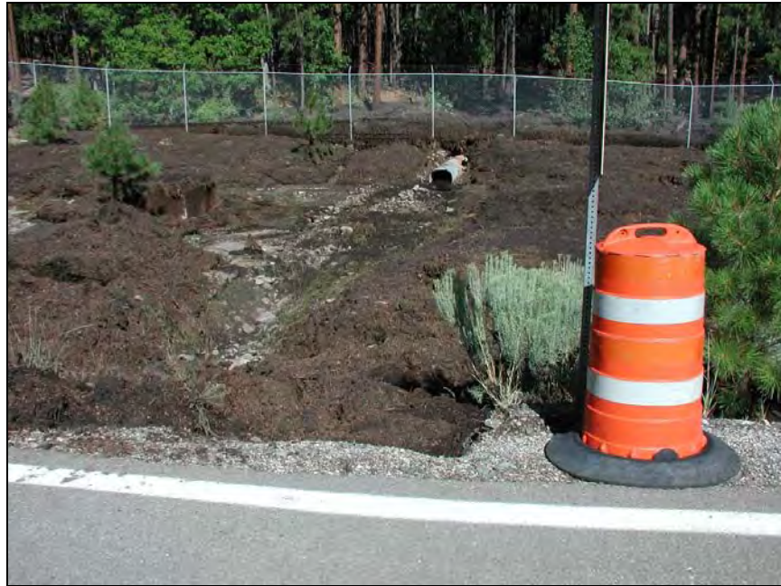
Photograph 39. Cleaned out culvert along Anchor Ranch Road.
