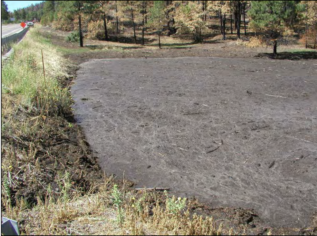
Photograph 37. Ponding of ash and debris along NM 501.
