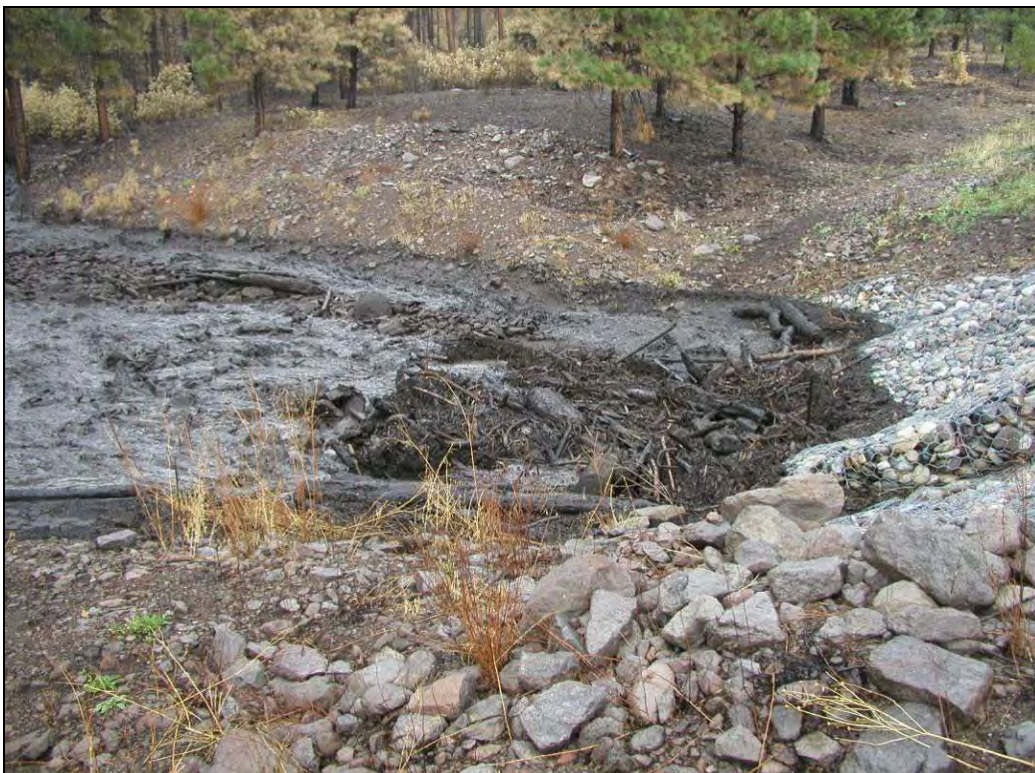
Photograph 38. Ash accumulation at Water Canyon crossing and NM 501.
