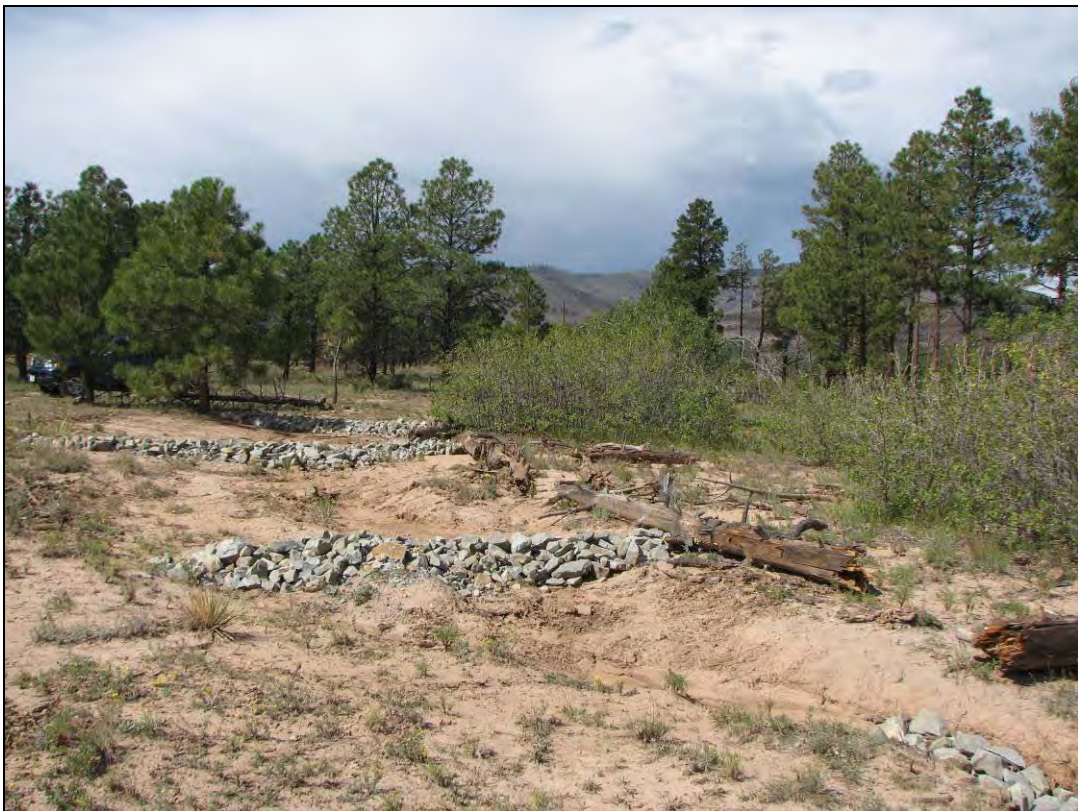
Figure 12. New rock erosion-control measures, LA 21334 (2011).
