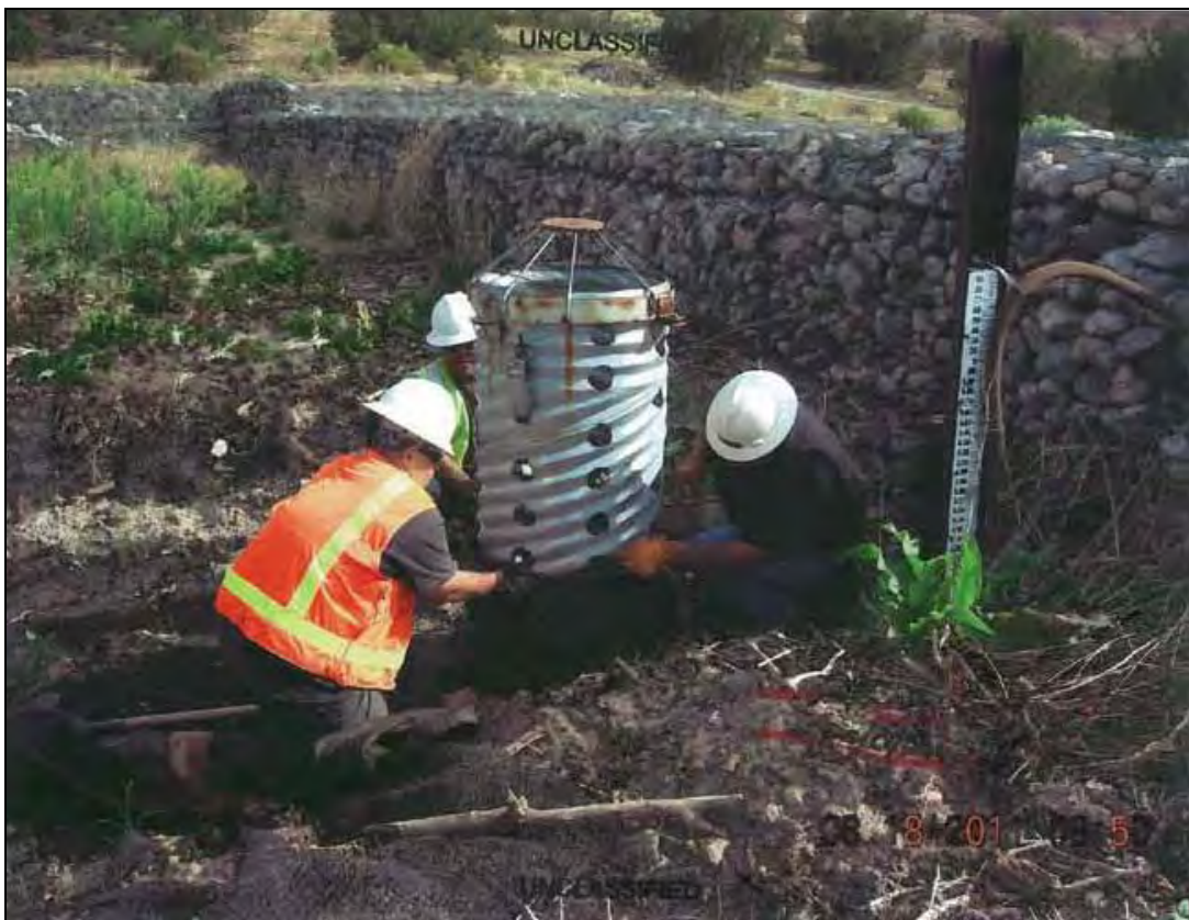
Photograph 9. Crews expose discharge standpipe and wrap it with filter fabric.
