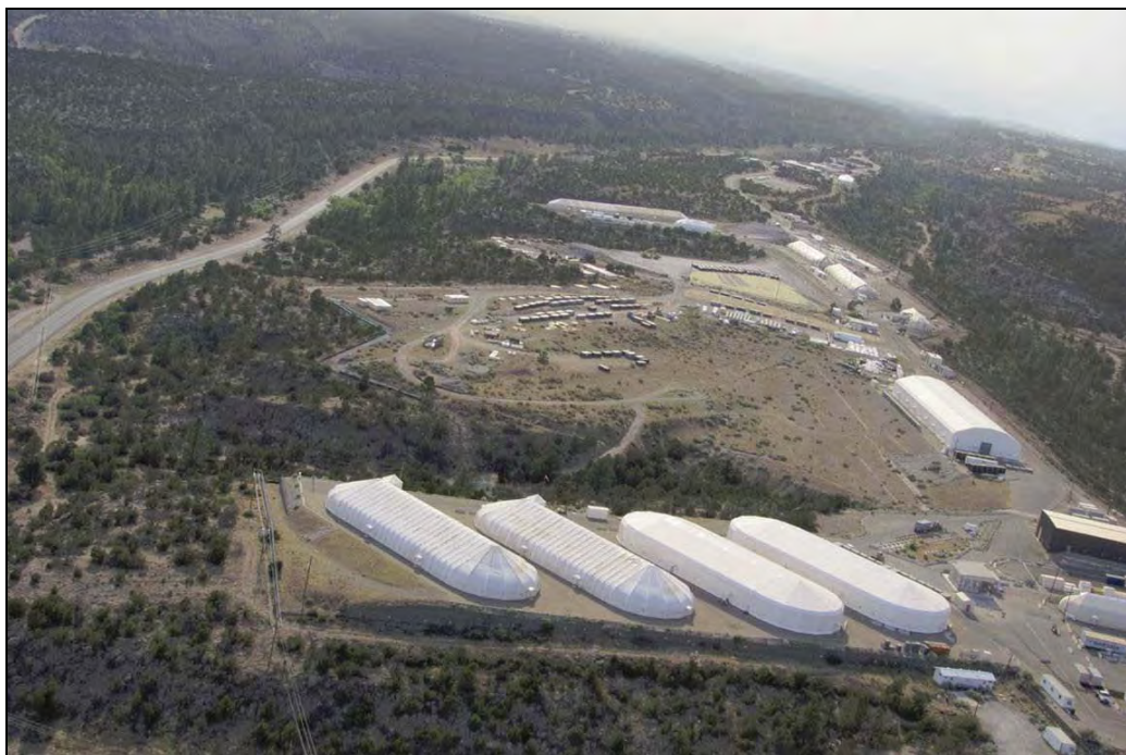
Photograph 18. Aerial view of TA-54, Area G, on June 29, 2011.
