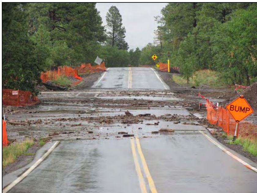
Photograph 40. Post-Las Conchas fire flooding impacts a road at LANL.
