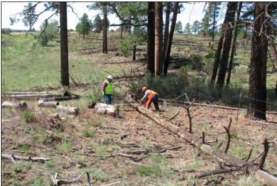
Figure 2. LA 89727, snag removal, facing south (FY 2011).
