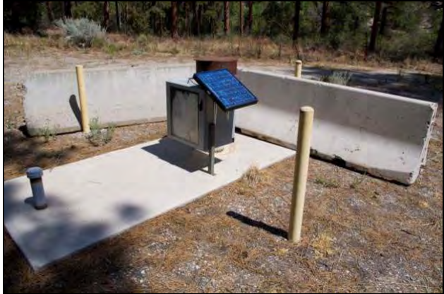
Photographs 12 and 13. Armoring at groundwater wellhead (left) and armoring of a sediment collection system (right).
