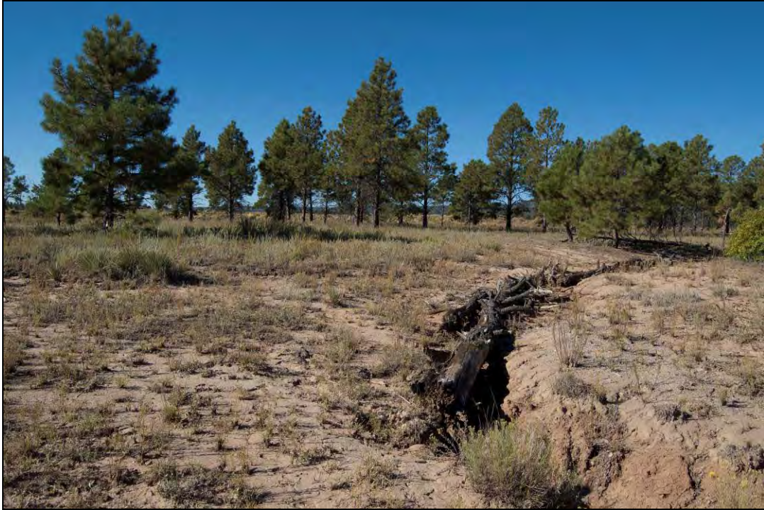
Figure 11. Detail of erosion channel, Montoya Homestead, LA 21334 (2010).
