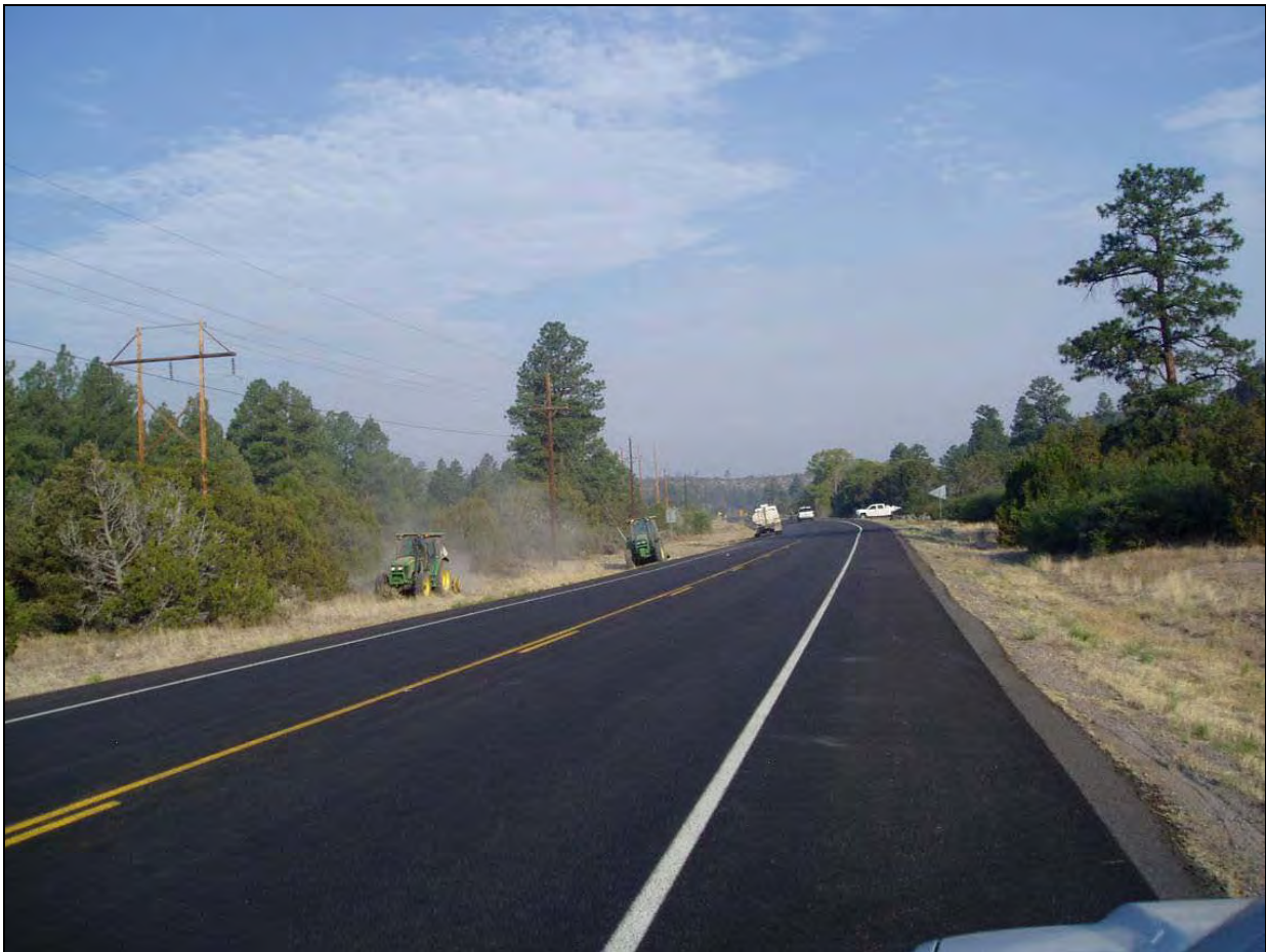
Photograph 15. Mowers work to create firebreaks along Pajarito Road.
