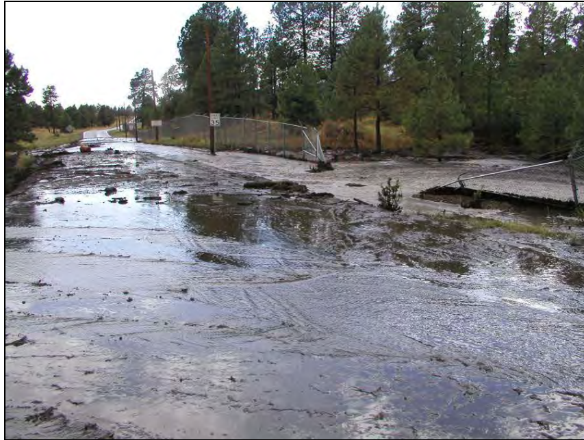
Photograph 41. Post-fire flooding at Anchor Ranch Road.
