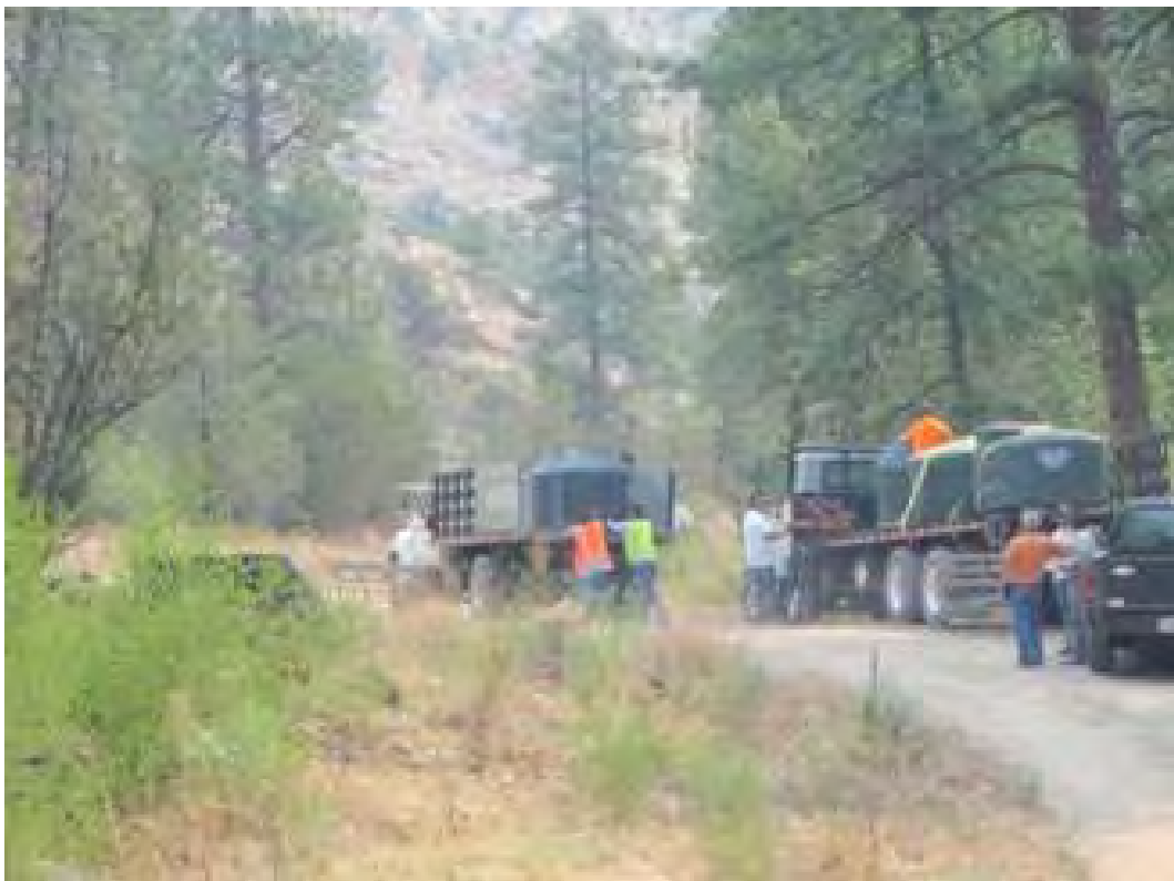
Photograph 10. Crews remove sediments and waste from canyon.
