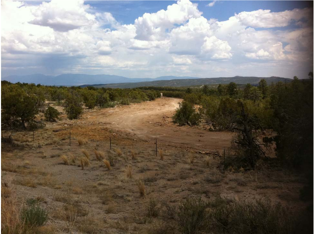
Figure 1. Example of new fire breaks in LANL Canyons.
