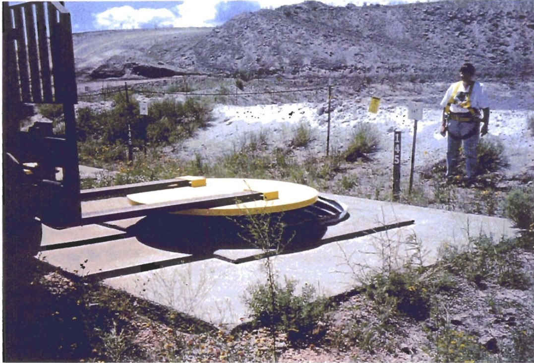
Figure 6. Operational Cap Removed for Inspection, Storage Shaft 145
