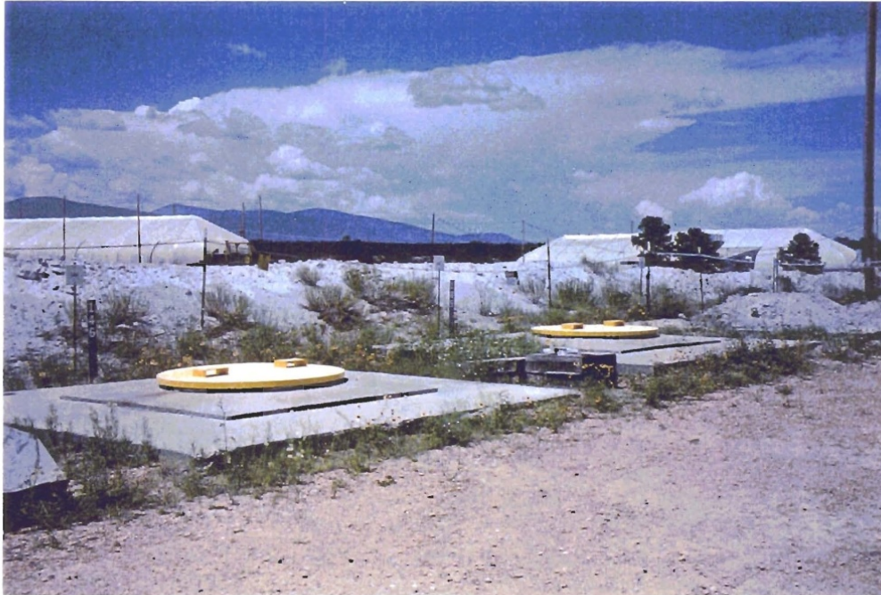
Figure 3. Storage Shafts 145 and 146
