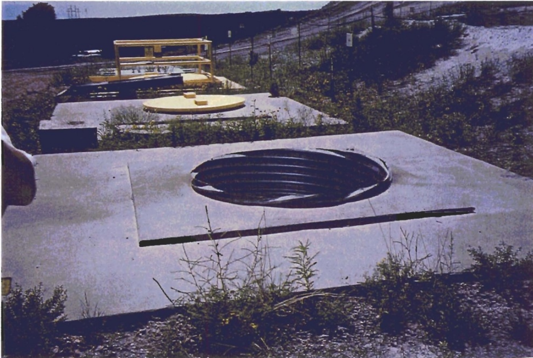
Figure 8. Surface View with Operational Cap Removed, Storage Shaft 145
