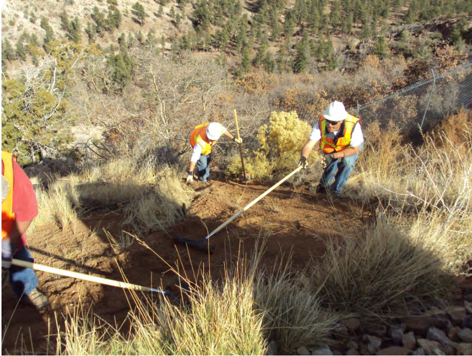
AREA T-FILLING RILL WITH FILL MATERIAL
