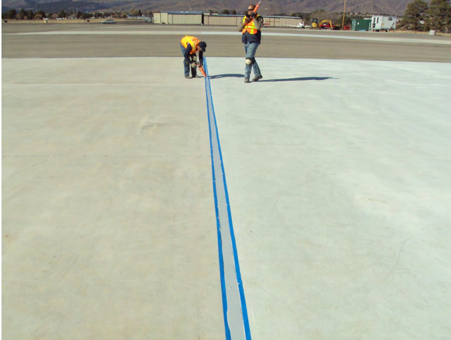
HANGAR PADS-FILLING CRACKS
