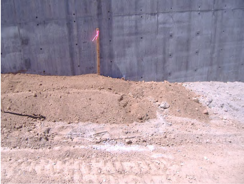
AREA 5 –USING CONSTRUCTION STAKING TO DETERMINE REQUIRED GRADE
