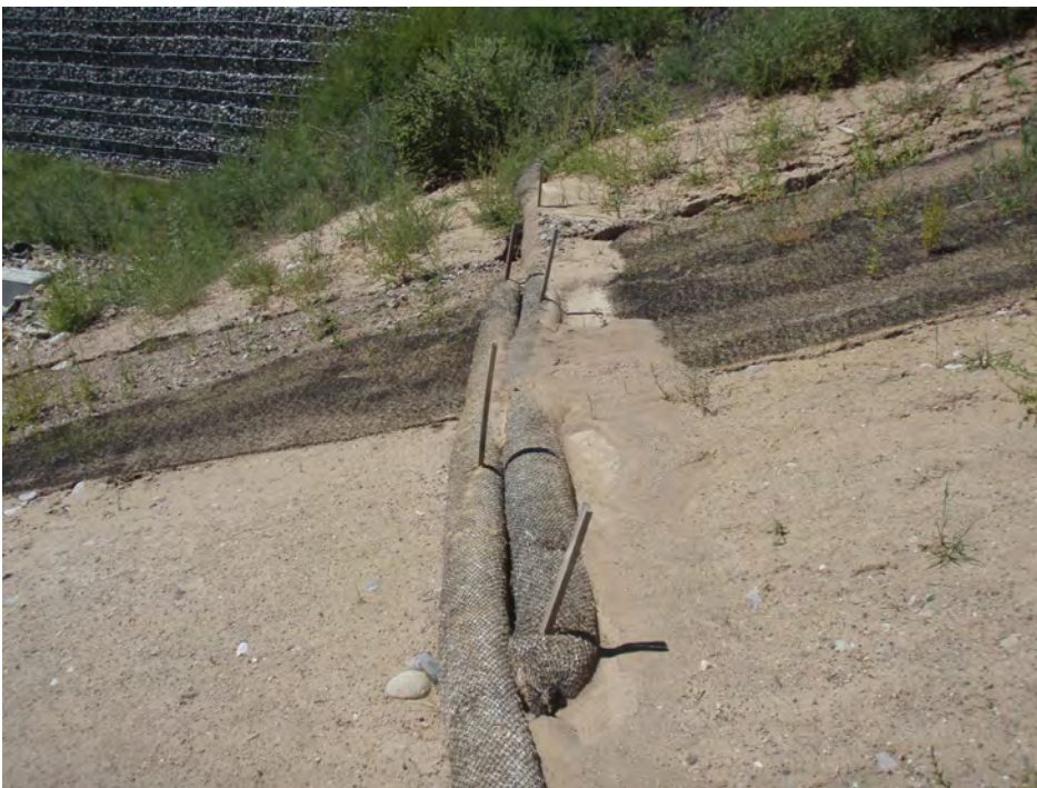
Figure 13 Sediment accumulation behind wattles in the wattle area
