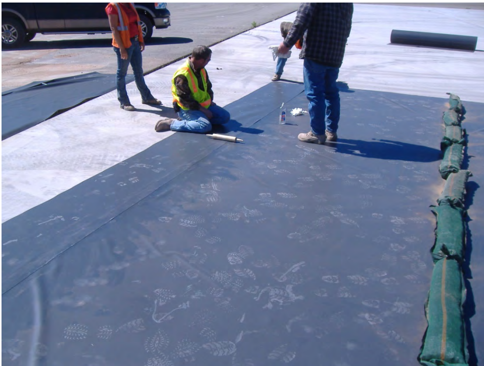
GEOMEMBRANE –SEAMING GEOMEMBRANE FOR USE UNDER POROUS DETENTION AREAS
