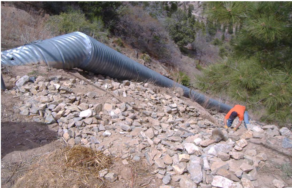
AREA C-FILLING RILL WITH RIP RAP AND TOPSOIL FILL MATERIAL
