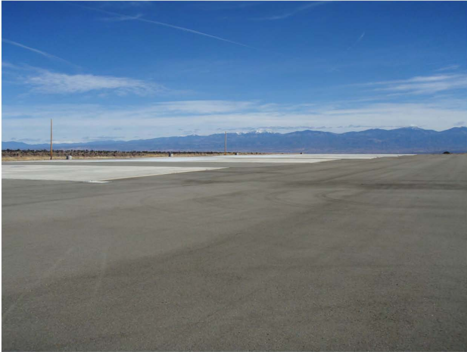
Figure 3 Looking northeast across the MatCon pavement and concrete hangar pads
