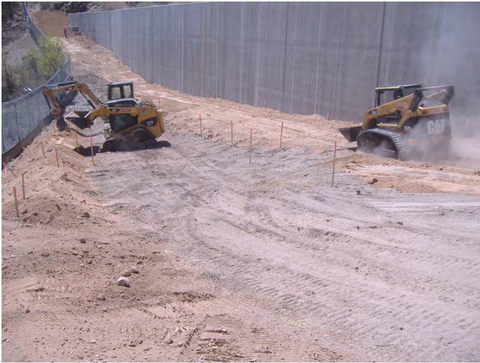
AREAS S –CONSTRUCTING POROUS DETENTION AREAS
