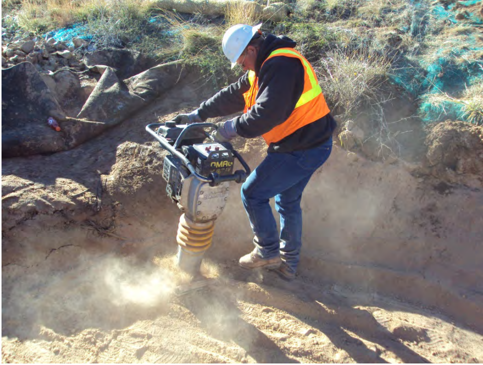
AREA L-COMPACTION OF INFILTRATION MATERIAL
