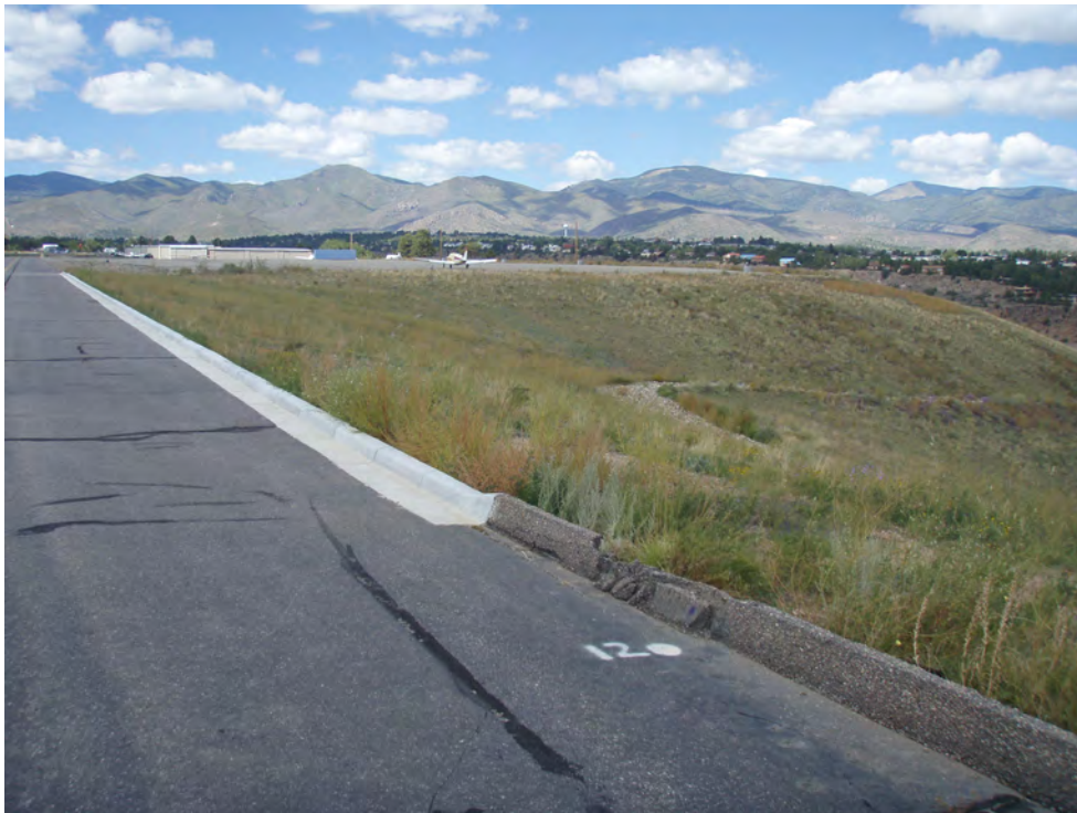
Figure 11 Curb installed in 2009 to control run-on to vegetative cap
