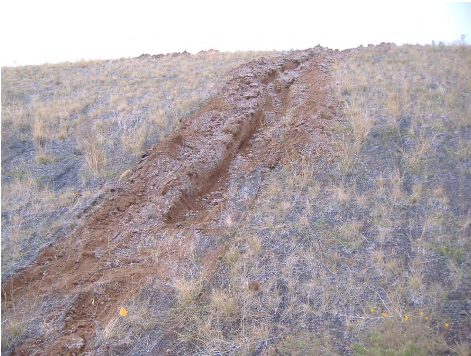
AREA I-TRM CUT AND REMOVED AND RILL PARTIALLY EXCAVATED
