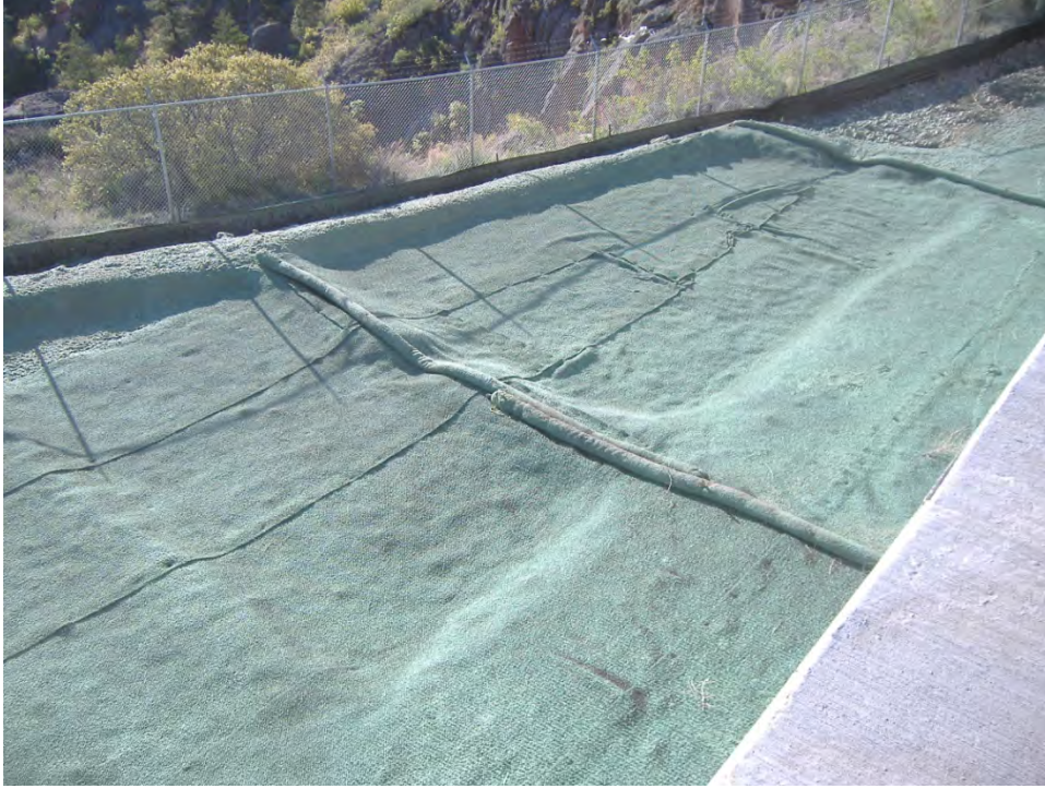
AREA S –GREEN ARMOR SYSTEM INSTALLED
