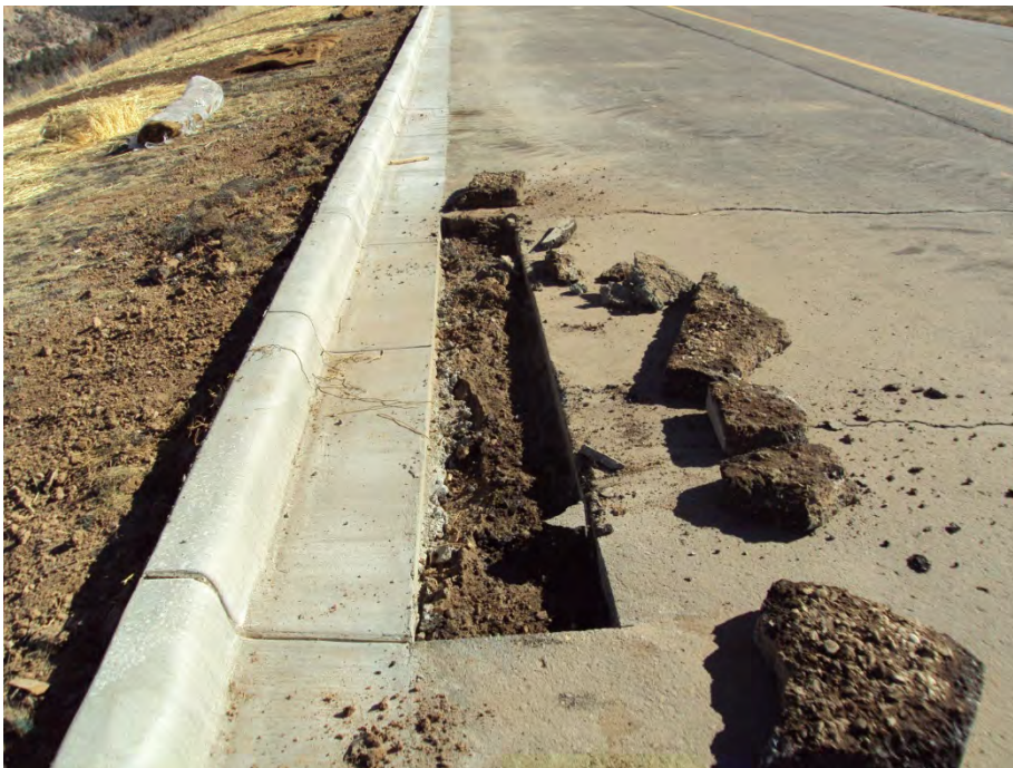
CONCRETE CURB AND GUTTER-PRIOR TO BITUMINOUS PATCH
