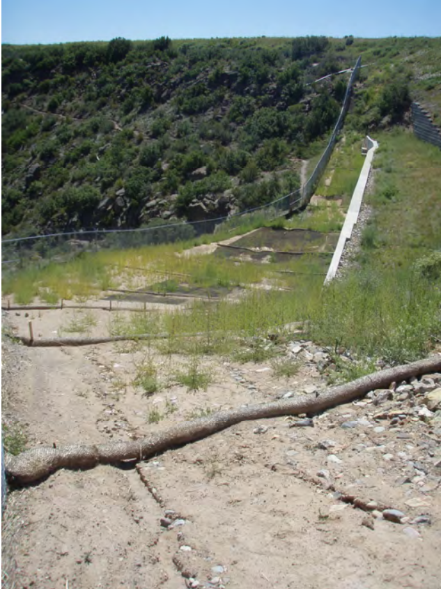
Figure 12 Rilling in wattle area
