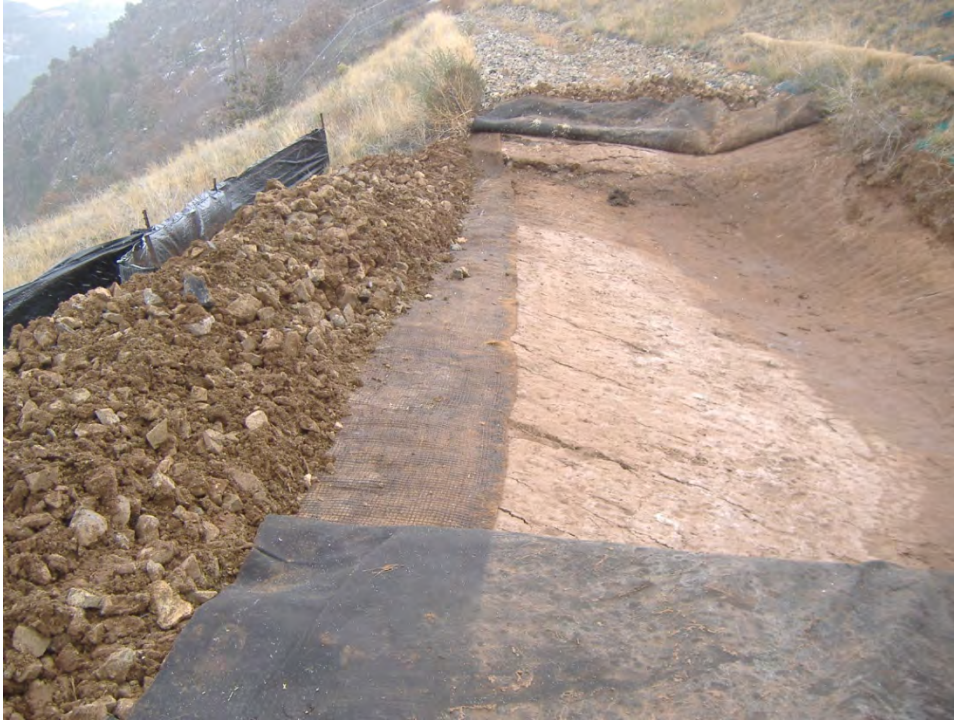
AREA L-SUBGRADE PRIOR TO SCARIFICATION AND PLACEMENT OF INFILTRATION MATERIAL
