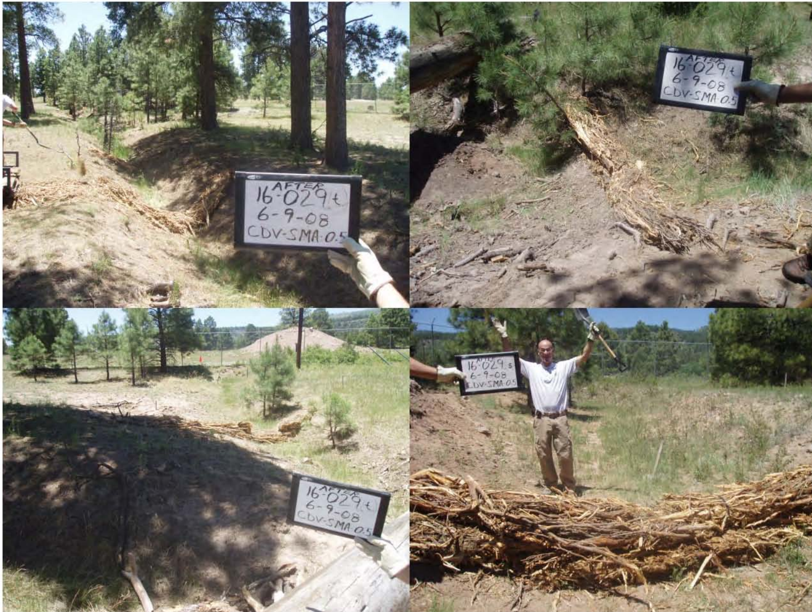
Figure 2 Drainages into the 90s Line Pond after BMP installation, June 2008
