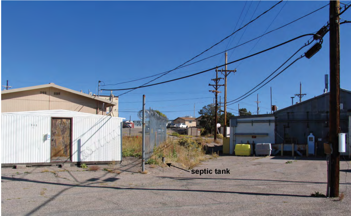
Figure B-10.0-1 Location of septic tank and overhead utilities at SWMU 46-003(a)
