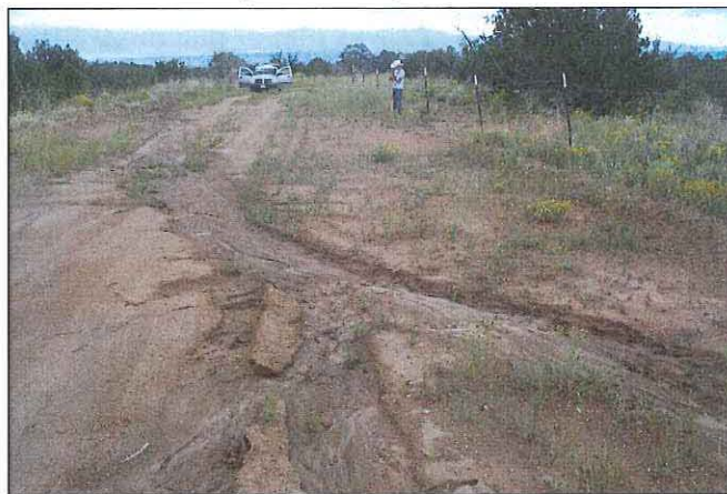
Figure 9. L. Maestas stands in the vicinity of the roomblock exposed in Firebreak 5 at LA 4697, erosion in the foreground is within a few meters of the roomblock (view east).
