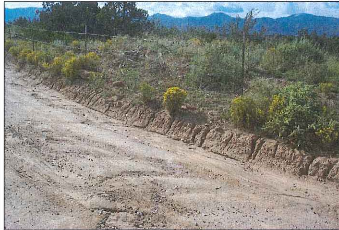
Figure 4. Eroded cut, roomblock mound is behind the center fence section (view west).
