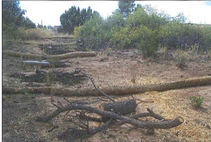
Figure 12. FY 2010 treatment (wattles and slash) at LA 89779 (view southwest).
