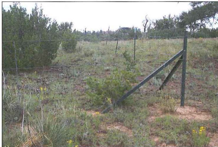
Figure 13. Sagging fence wire at LA 30642 (view southwest).
