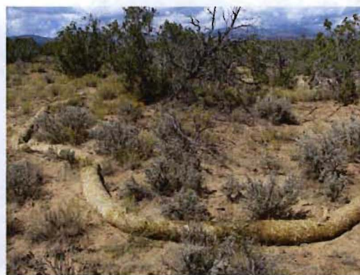
Figure 2. Wattle installation at a site in TA-70. Figure 3. Wattle installation at a site in TA-70.
