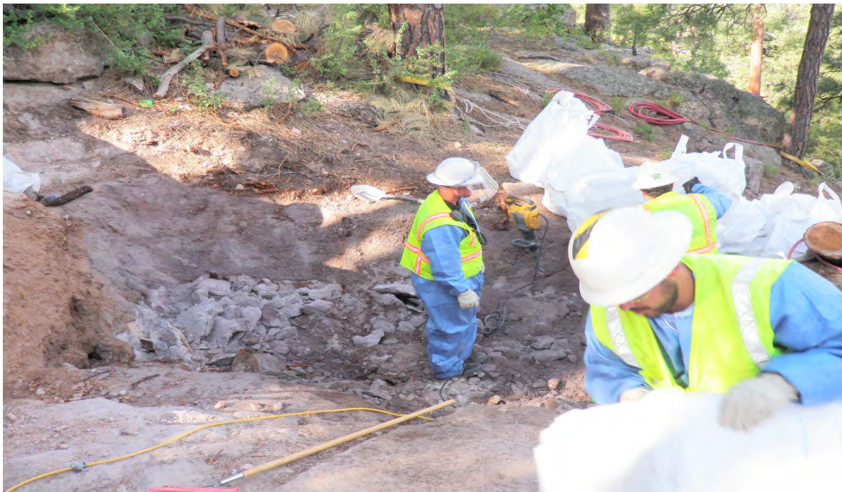
Excavation and packaging of contaminated media within the SWMU-01-001(f) outfall area
