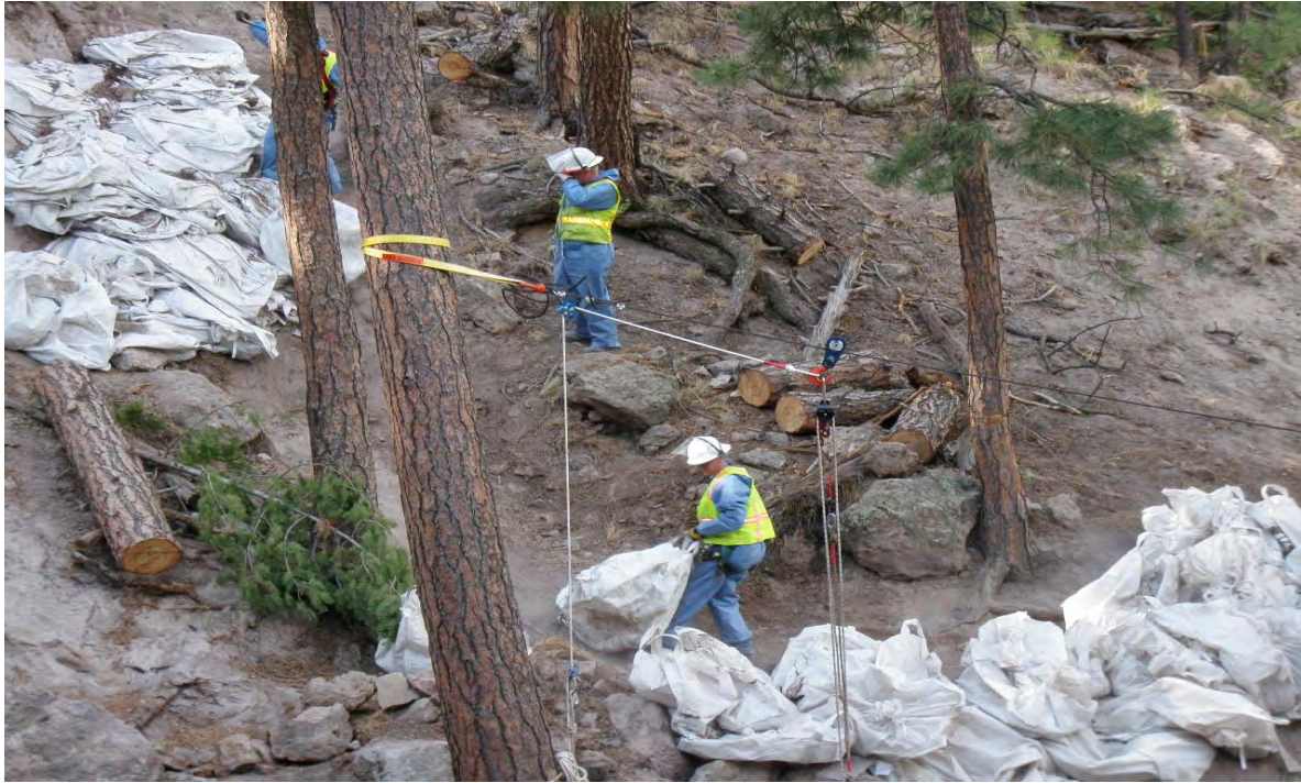
Packaging of contaminated media from the drainage below the SWMU 01-001(f) outfall
