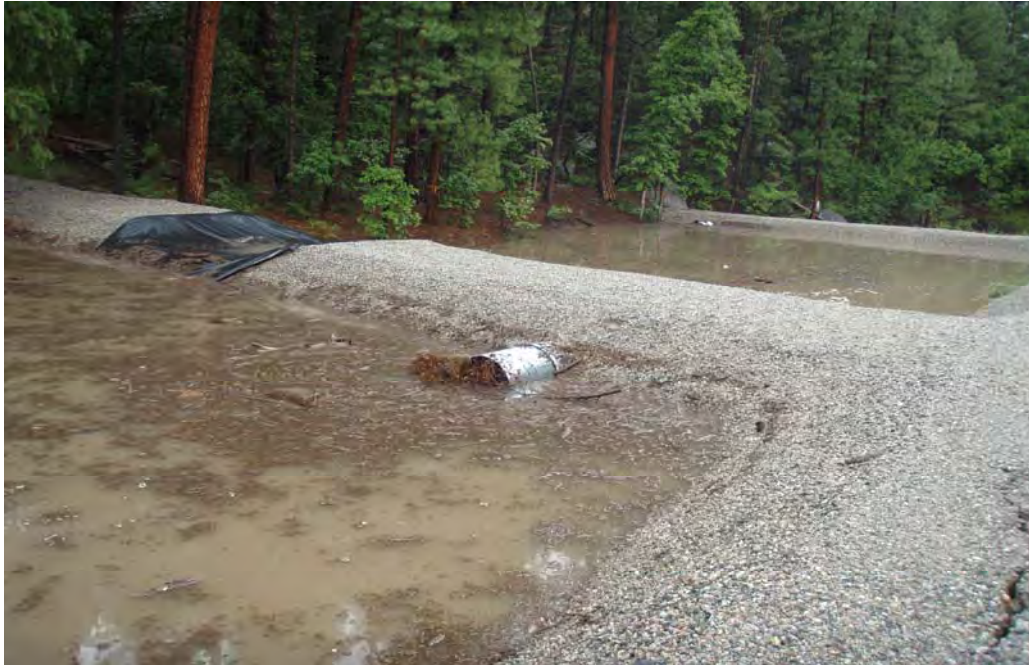
Upper and lower retention basins following significant precipitation events on August 15 and 16, 2010
