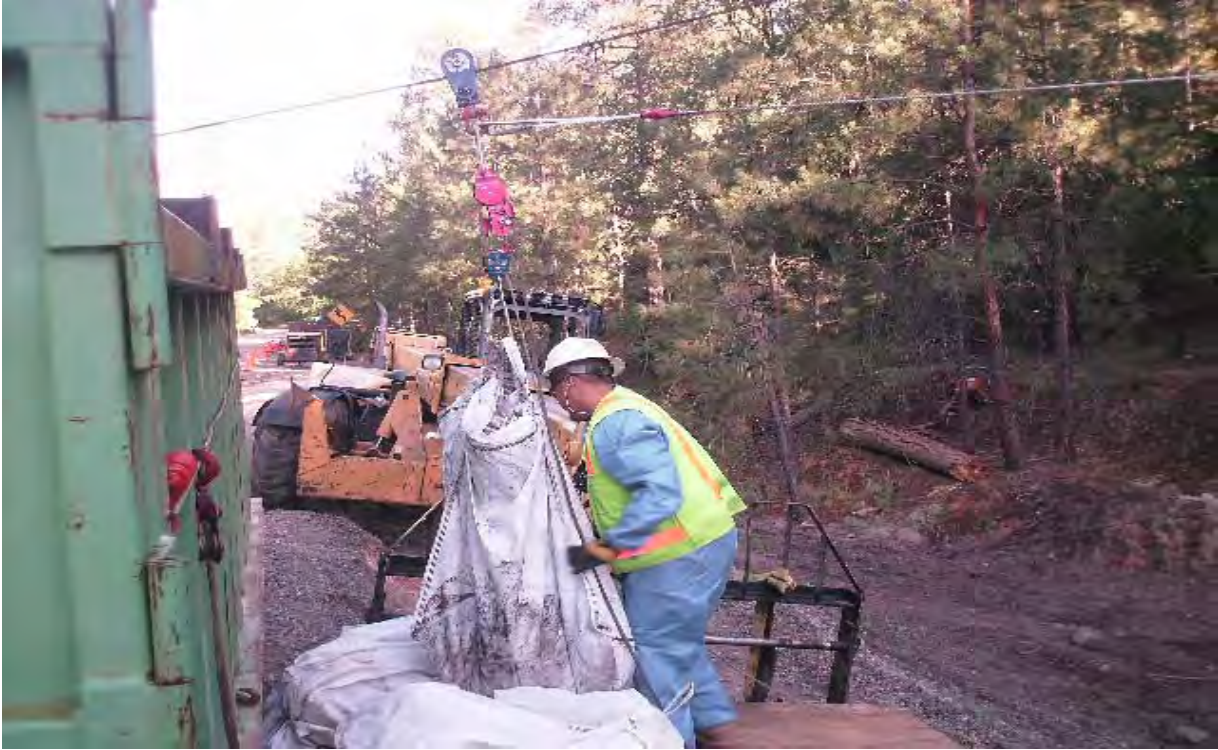
Unloading waste bags from zip line in Los Alamos Canyon
