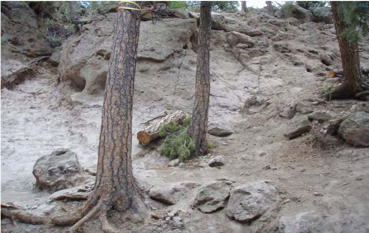
Excavated Area 3 in the drainage below the SWMU 01-001(f) outfall following supplemental removal of contaminated media
