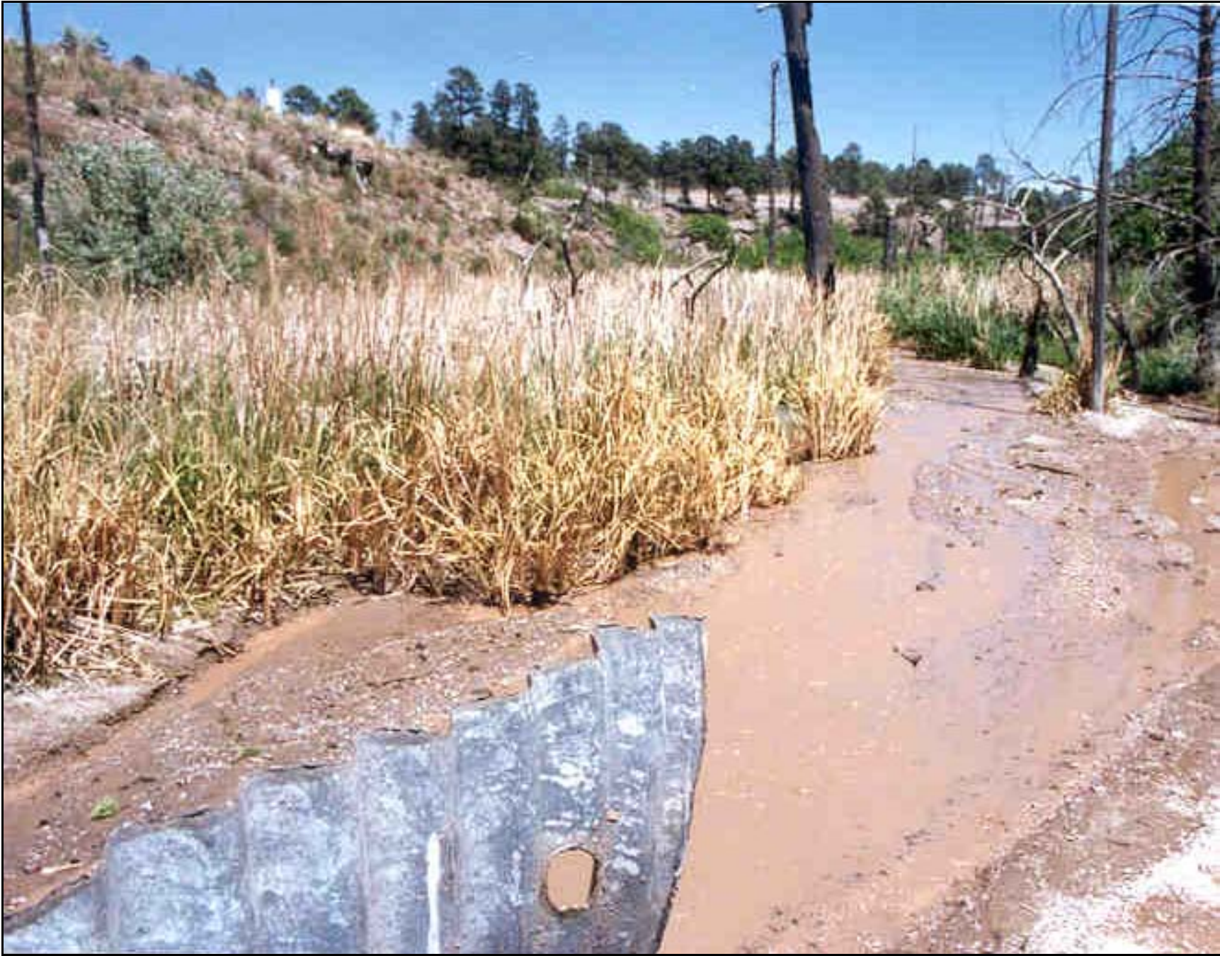
(Photo A) 1990 – Looking east from the outfall
