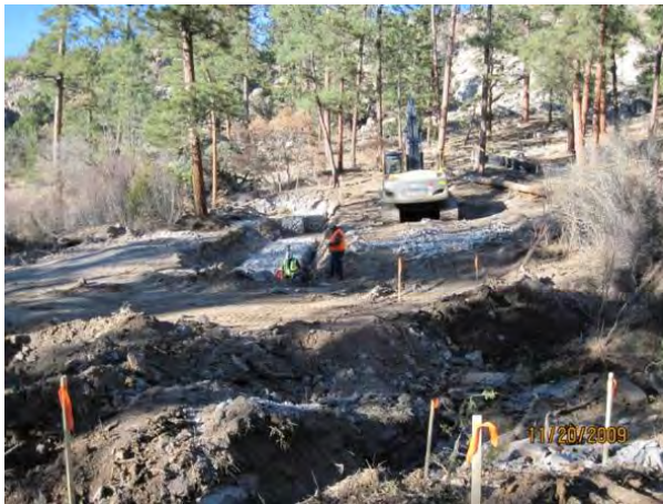
Photo 1 Structure construction, looking north
