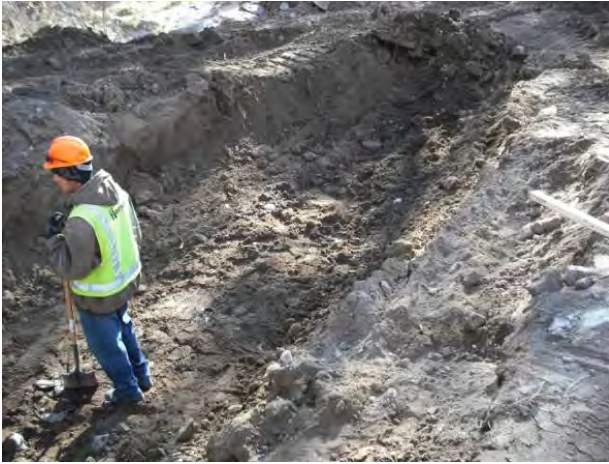
Photo 5 Excavated north half of structure
