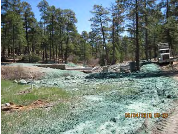
Photo 1 DP Canyon hydroseeding
