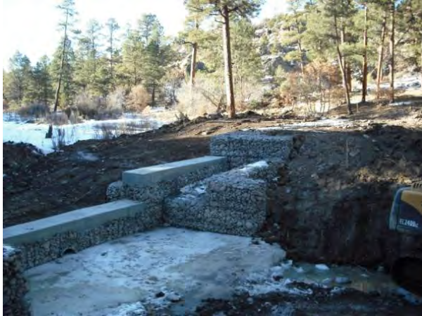
Photo 5 Downstream, facing side of structure, ice-filled stilling basin, looking northwest
