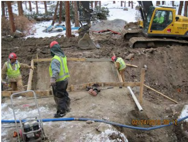
Photo 1 Forming flume for concrete placement
