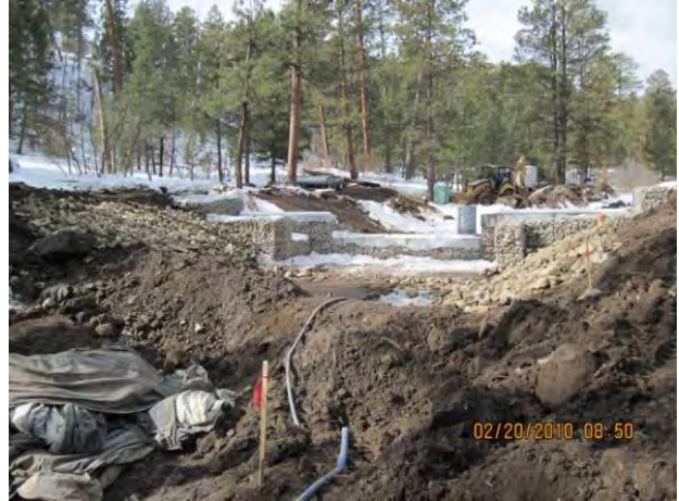
Photo 6 Looking upstream at downstream, facing side of structure from flume location
