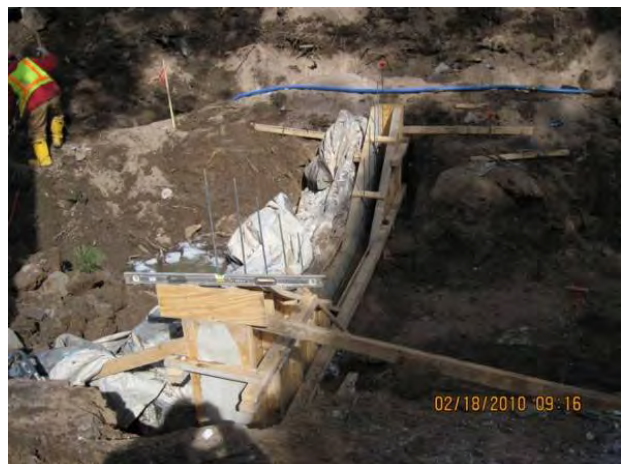
Photo 10 West headwall form, prior to concrete placement
