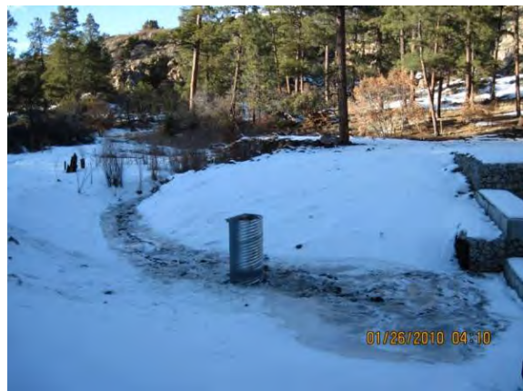
Photo 2 Riser pipe looking northwest
