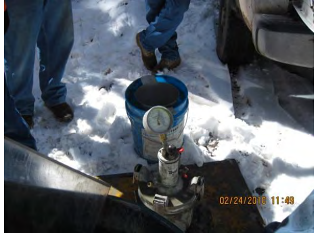
Photo 8 Concrete test of flume
