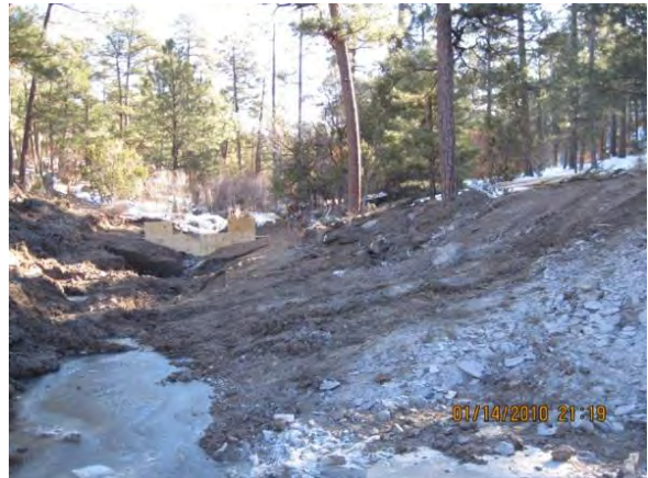
Photo 6 Flume headwall forms, looking downstream from structure
