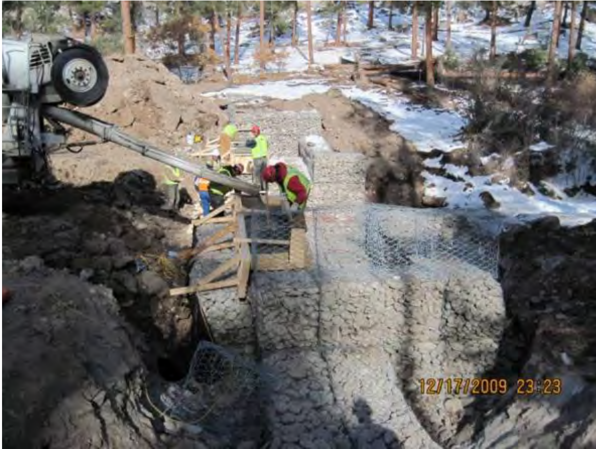
Figure 2.1-3 Concrete cap placement
