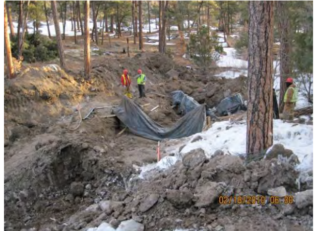
Photo 4 Newly placed flume headwalls covered with concrete blankets to cure
