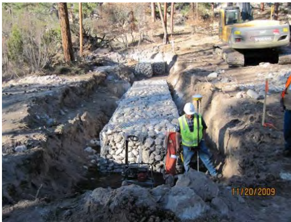
Photo 3 Structure subgrade gabion baskets, looking north
