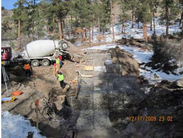
Photo 1 Placing concrete cap on low-flow and overflow weir
