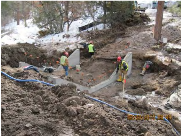
Photo 3 Preparing flume subgrade, concrete headwalls complete
