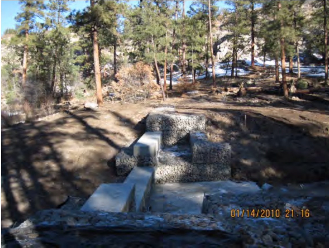
Figure 2.1-1 DP grade-control structure (looking north)
