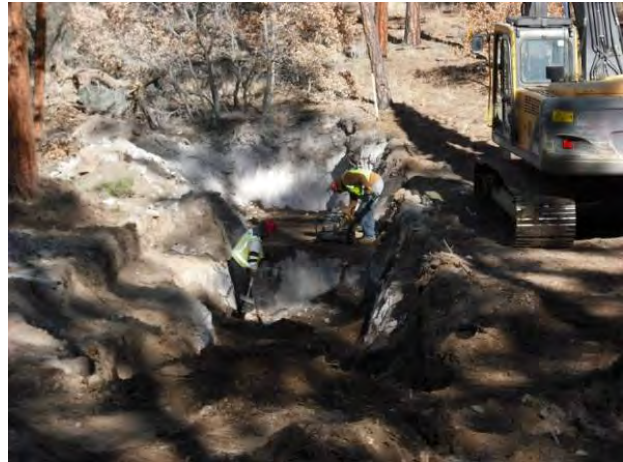
Photo 4 Structure subgrade compaction, north half, looking north
