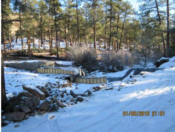
Photo 1 Looking downstream at structure, concrete blankets covering concrete cap
