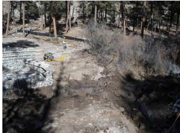
Photo 8 Stilling basin excavation, looking northeast
