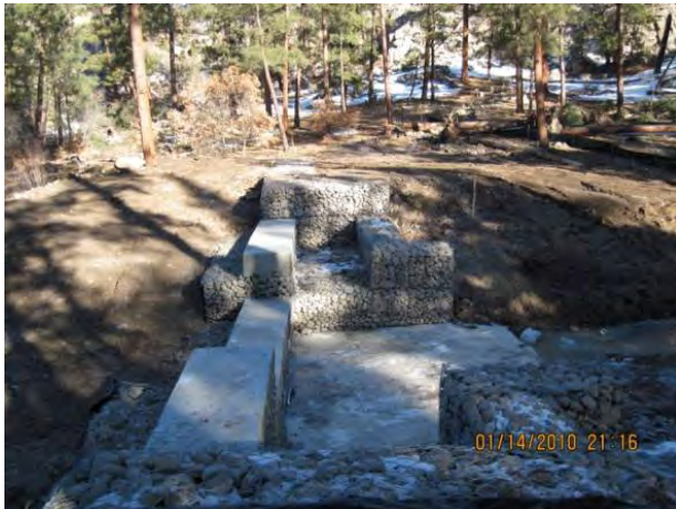
Photo 1 Structure, looking north
