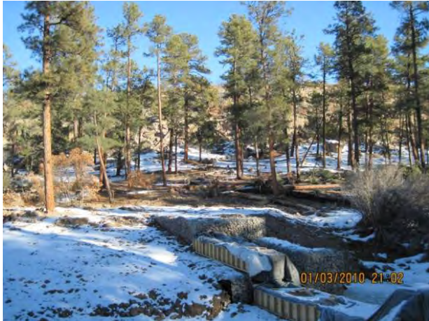
Photo 3 Looking northeast at structure, concrete blankets covering concrete cap
