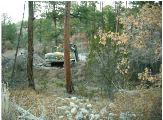
Photo 4 Excavation for structure
