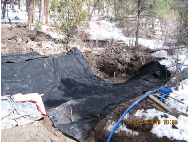
Photo 1 Flume concrete covered with concrete blankets to cure, looking northeast
