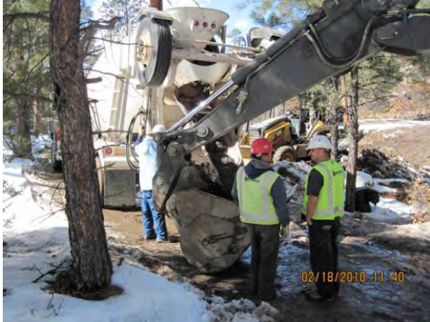
Photo 11 Concrete for headwall placement
