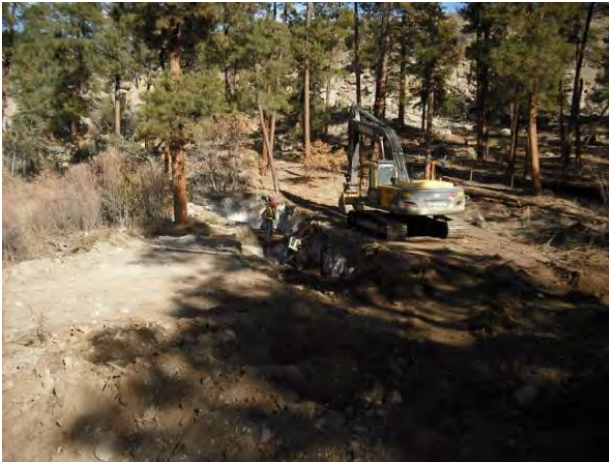
Photo 3 North half of structure subgrade compaction, looking north
