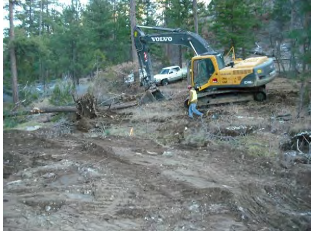
Photo 2 Excavation for structure, looking northwest
