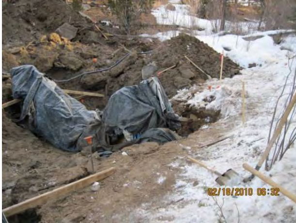
Photo 1 Newly placed concrete headwall covered with blanket to cure
