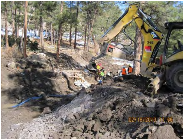
Photo 17 Placing headwall concrete
