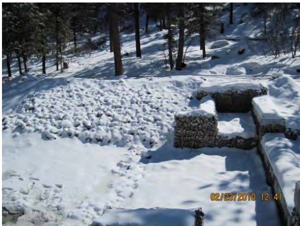
Photo 1 Grade control structure, looking south
