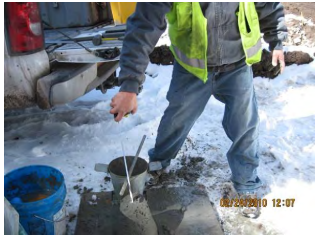
Photo 10 Slump Test for flume concrete placement
