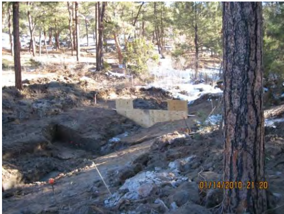
Photo 5 Forms for flume headwall concrete placement, looking northeast from access road
