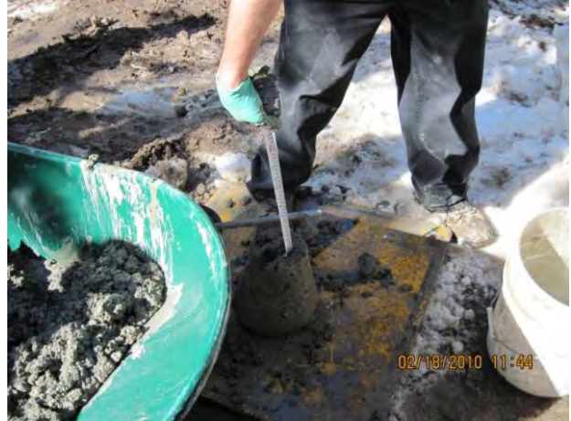
Photo 12 Headwall concrete slump test
