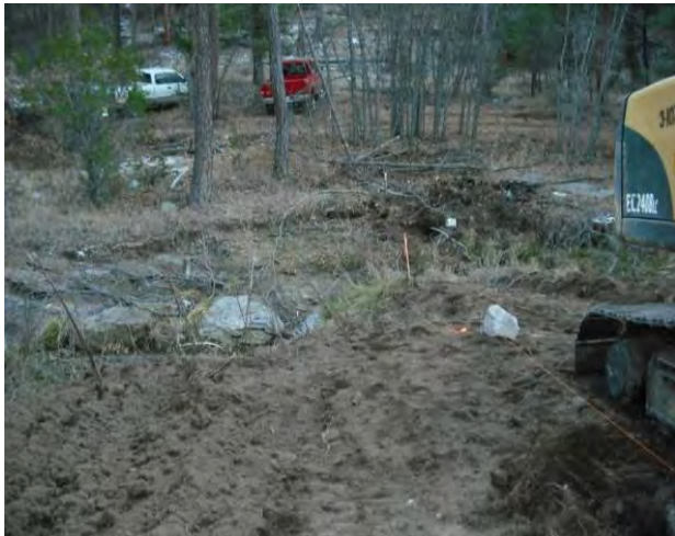
Photo 3 Clearing for structure, looking south
