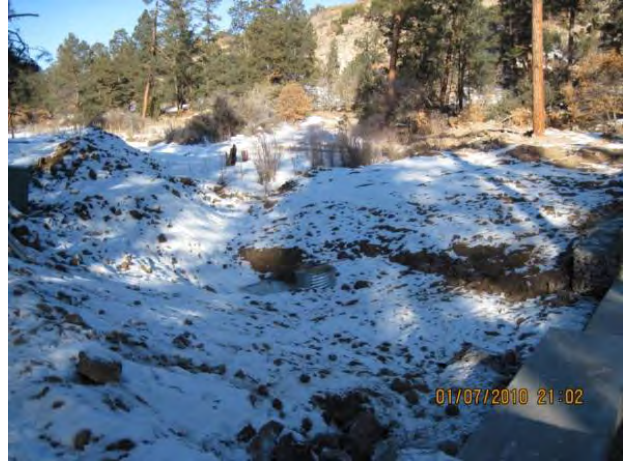
Photo 2 Riser pipe, before extension
