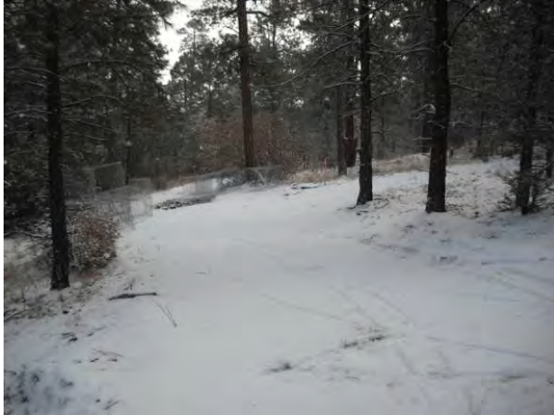
Photo 1 Gabion assembly area, looking east
