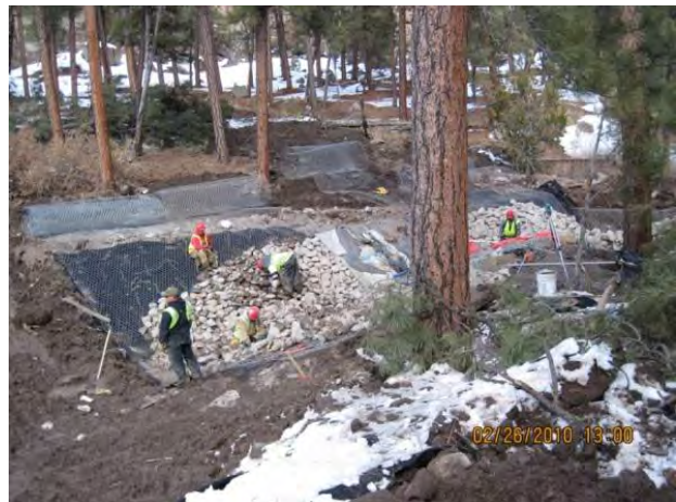
Photo 2 Installation of Class A rip rap on upstream and downstream sides of flume
