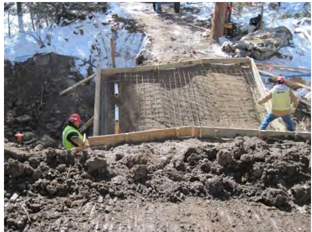
Photo 4 Wire mesh reinforcement installed in flume form prior to concrete placement
