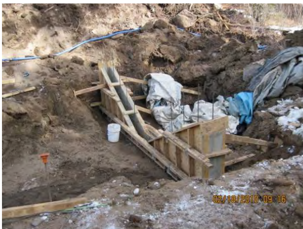
Photo 9 East headwall form, prior to concrete placement
