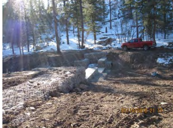
Photo 4 Completed structure, looking south
