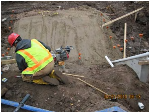
Photo 3 Compaction of flume subgrade
