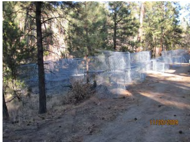
Photo 2 Gabion basket assembly area
