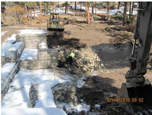
Photo 1 Class B rip rap installation, on north slope, downgradient of structure
