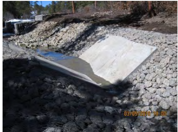
Photo 2 Completed flume, looking west/northwest
