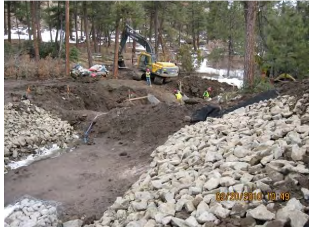
Photo 8 Looking northeast from access road at flume subgrade preparation
