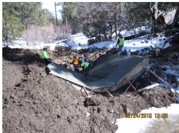
Photo 12 Flume concrete placement and finishing
