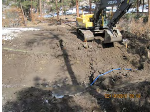
Photo 6 Preparing north slope, downstream of structure, for rip rap installation
