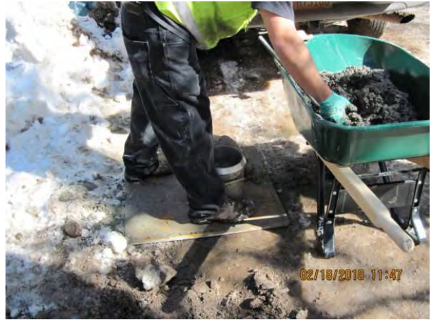
Photo 14 Setting up for concrete test
