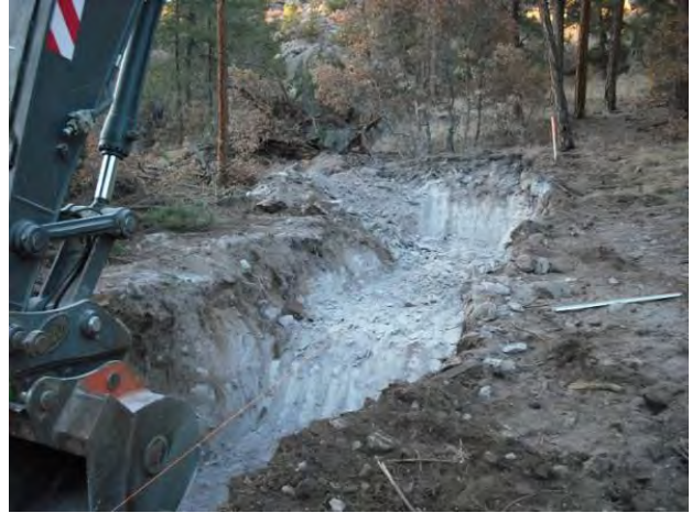
Photo 6 Structure excavation, looking northwest
