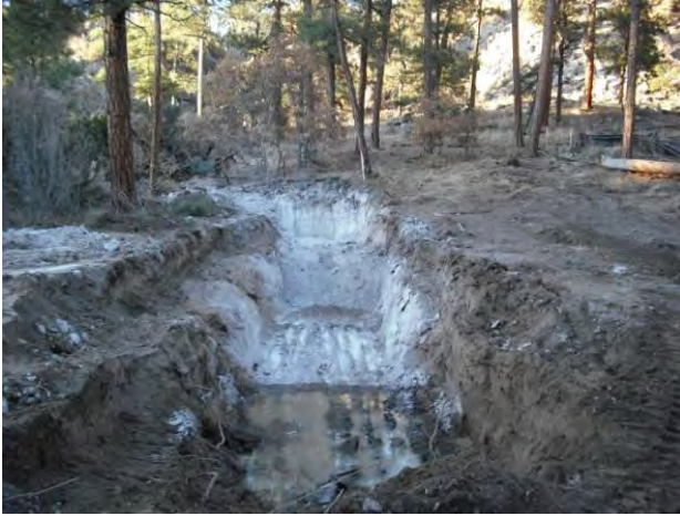
Photo 5 Structure excavation, looking north
