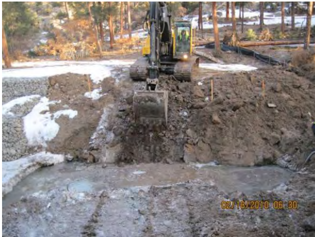
Photo 7 Preparing north slope, downstream of structure, for rip rap installation
