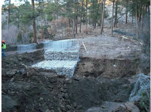
Photo 2 Structure, looking north; subgrade and above grade gabion baskets
