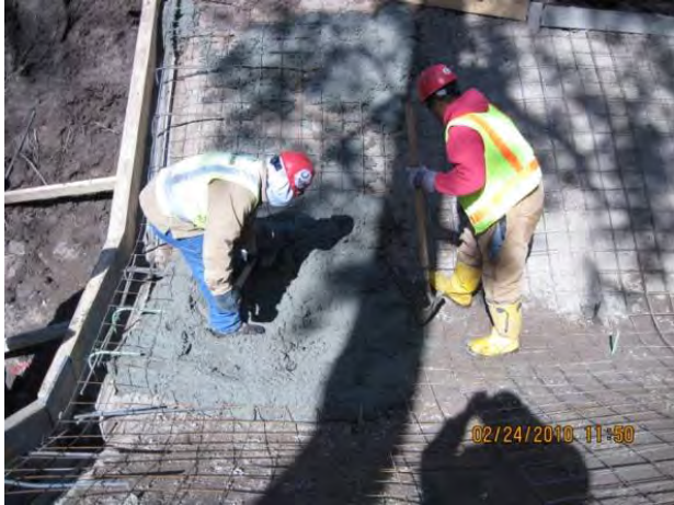
Photo 7 Flume concrete placement
