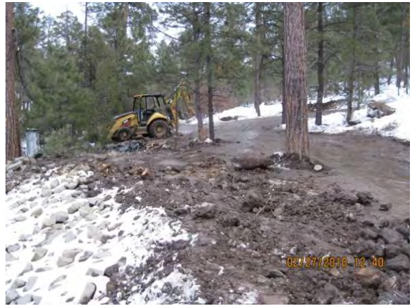
Photo 4 Looking east, towards Stream Gage stilling well and access road
