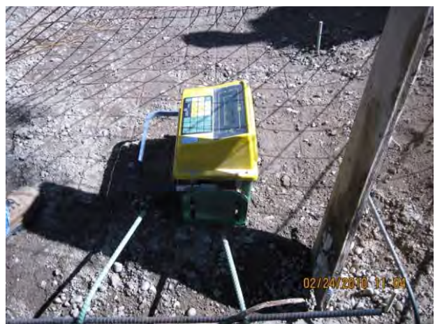
Photo 6 Measuring flume subgrade temperature prior to concrete placement
