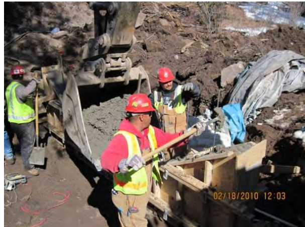
Photo 18 Placing headwall concrete
