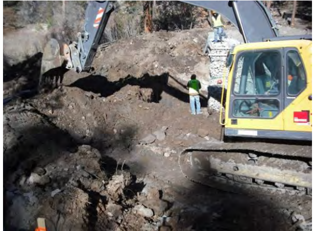
Photo 4 Structure construction, looking north/northwest
