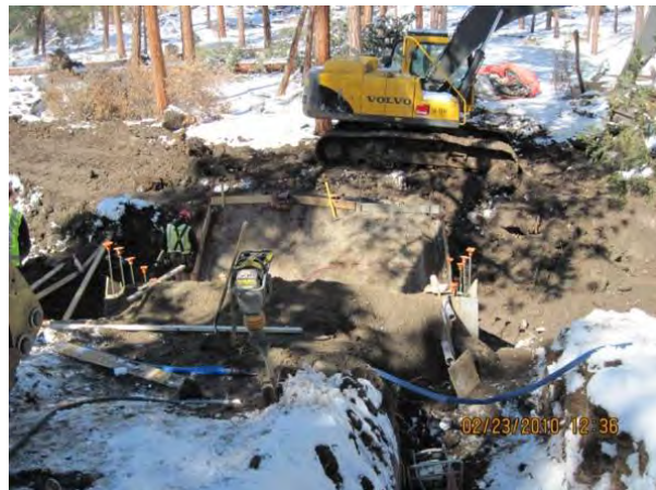
Photo 2 Work on flume subgrade
