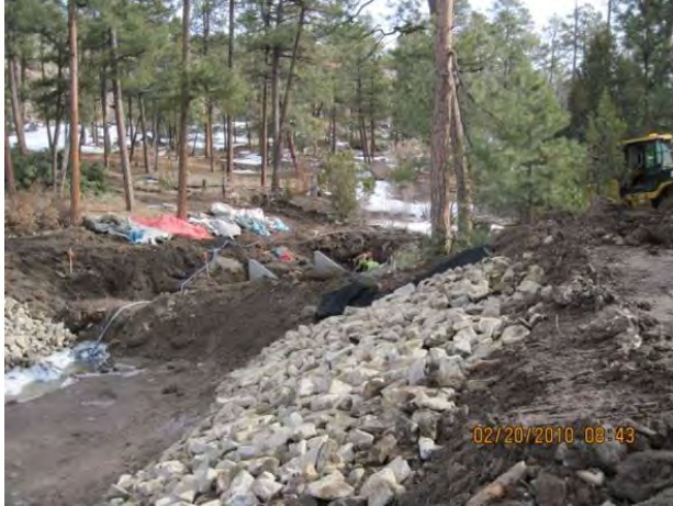
Photo 1 Class B rip rap on south slope, downgradient of structure
