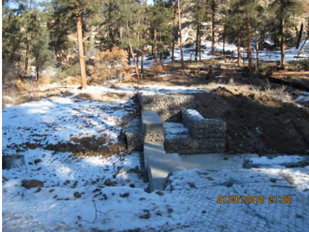
Photo 1 Looking north, at structure and concrete cap
