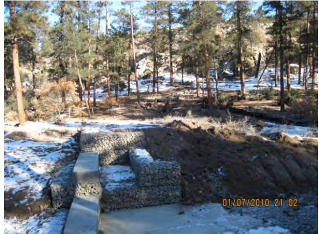
Photo 4 Structure, looking north; concrete cap on low-flow and overflow weir crests
