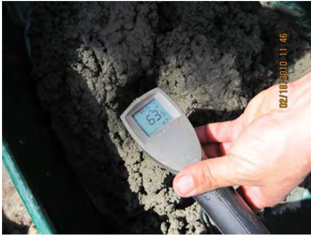
Photo 13 Monitoring headwall concrete temperature
