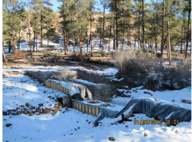
Photo 2 Looking northeast at structure, concrete blankets covering concrete cap
