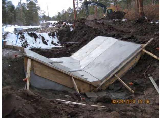
Photo 14 Finished flume concrete
