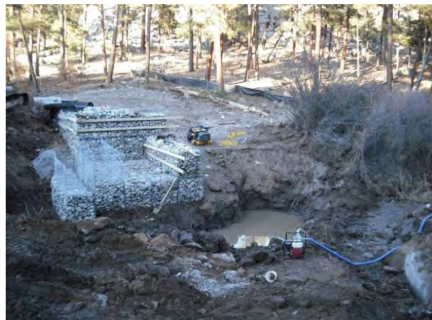
Photo 10 Structure construction, north half, pumping groundwater from stilling basin excavation
