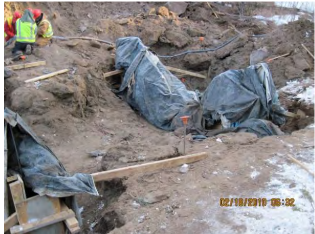
Photo 8 Concrete blankets cover newly placed concrete headwalls
