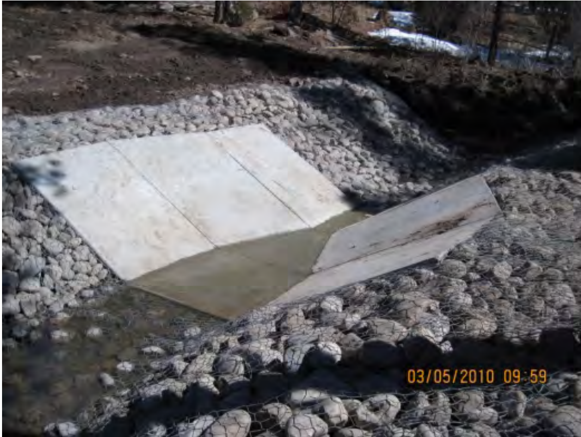
Figure 2.1-5 E039.1 supercritical-flow flume/stream gage
