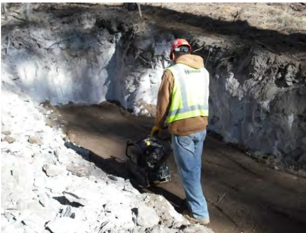
Photo 7 Subgrade compaction, north half
