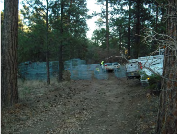
Photo 1 Gabion basket assembly area
