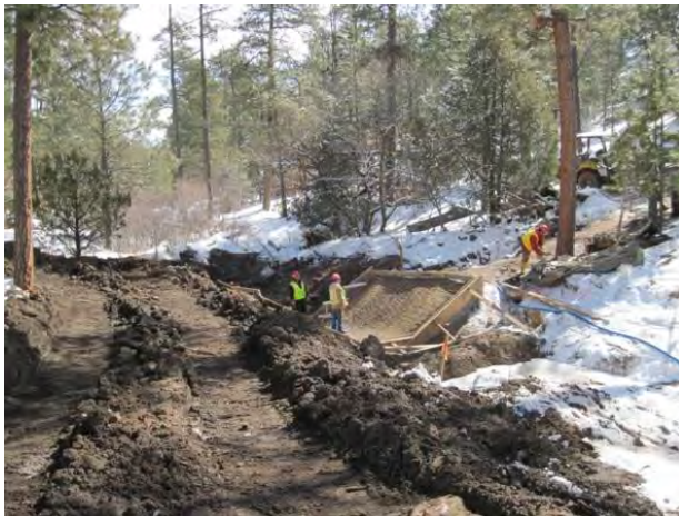
Photo 3 Wire mesh reinforcement installed in flume form prior to concrete placement
