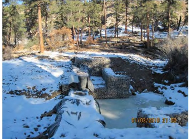
Photo 4 Looking north at structure, ice covers stilling basin
