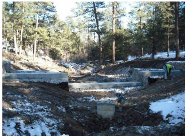
Photo 4 Looking at upstream side of structure, flume location in background
