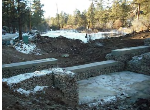
Photo 6 Downstream, facing side of structure, ice-filled stilling basin, looking west
