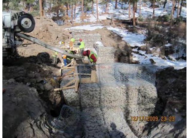
Photo 2 Placing concrete cap on low-flow and overflow weir
