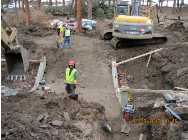
Photo 7 Preparing flume subgrade
