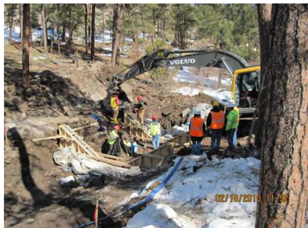
Photo 16 Placing headwall concrete
