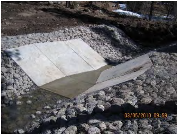
Photo 1 Completed flume, looking east/northeast
