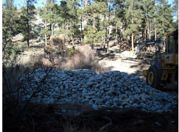
Photo 2 Gabion stone stockpile
