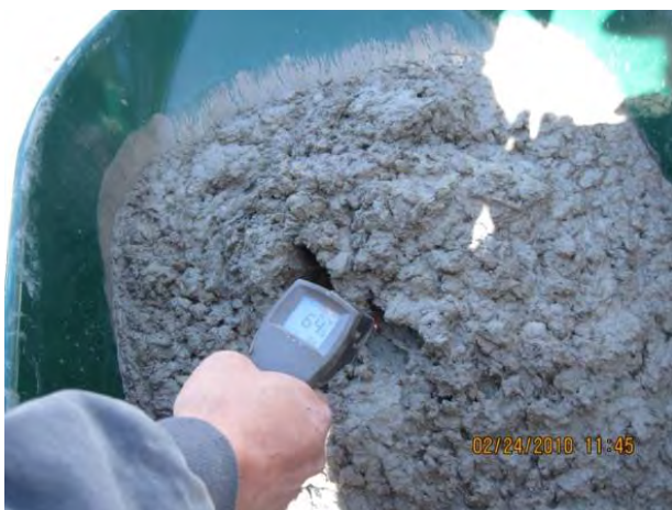
Photo 5 Measuring concrete temperature for flume concrete placement
