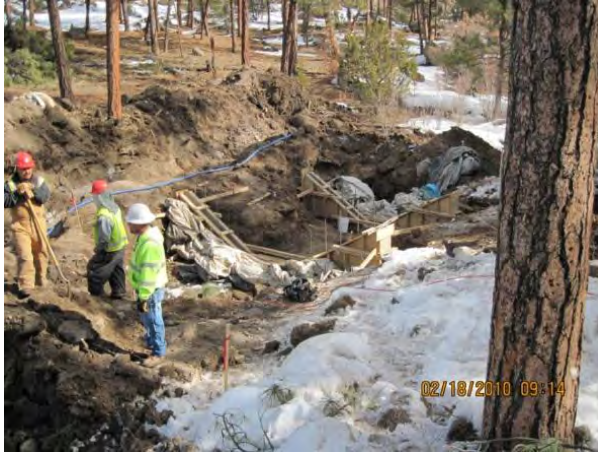
Photo 5 Flume headwall forms prior to placing concrete
