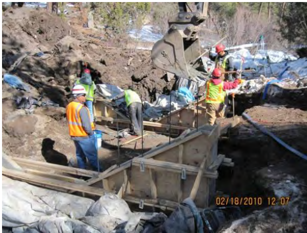
Photo 19 Placing headwall concrete
