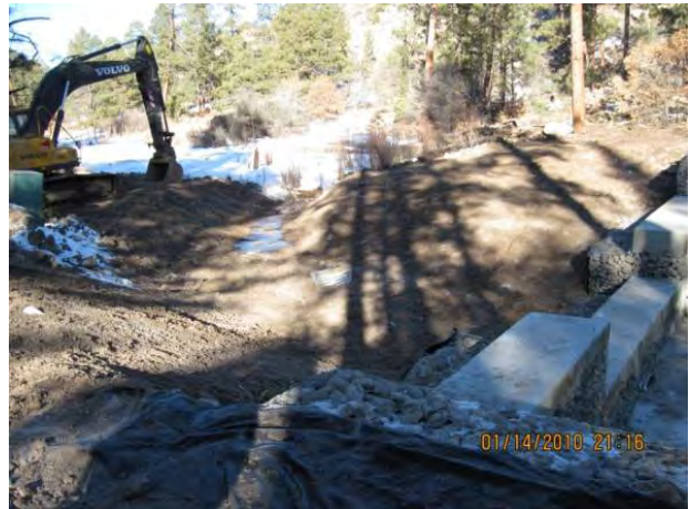
Photo 2 Upstream approach to structure
