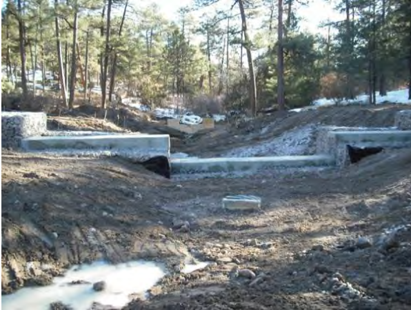
Photo 1 Upstream face of structure, riser pipe before extension
