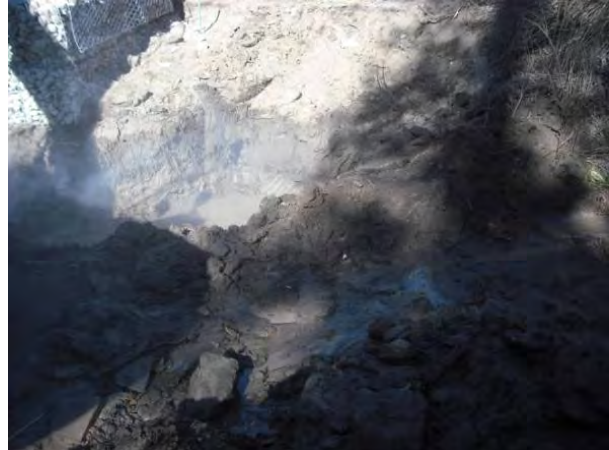
Photo 6 High water mark within stilling basin excavation area
