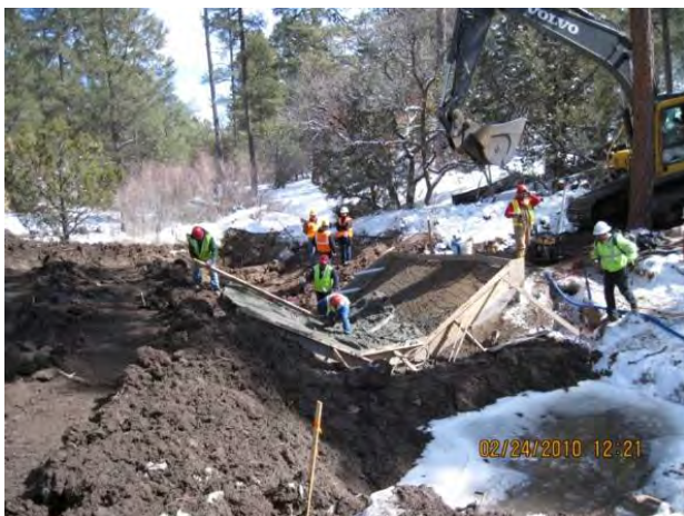
Photo 11 Flume concrete placement and finishing
