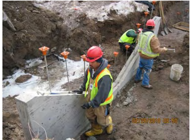
Photo 4 Concrete headwall
