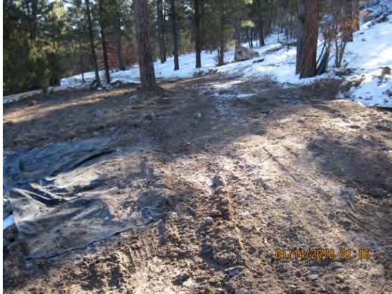
Photo 3 Access road crossing southern confinement wall gabion baskets, looking east
