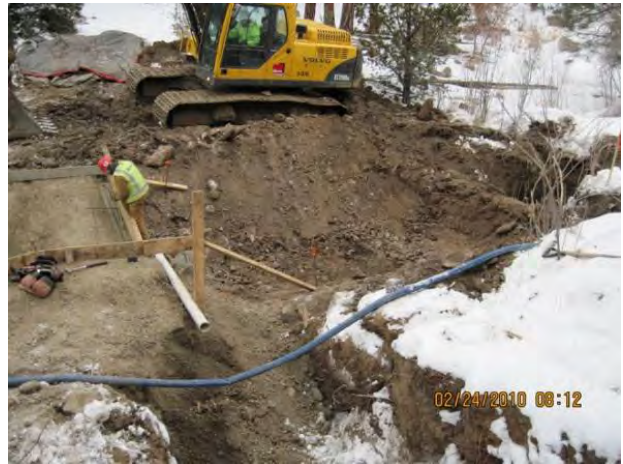
Photo 2 Forming flume for concrete placement
