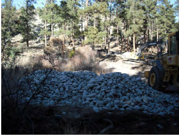
Photo 1 Gabion stone stockpile area
