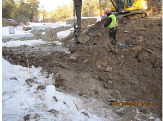
Photo 2 Excavation for Class B rip rap installation upstream of flume
