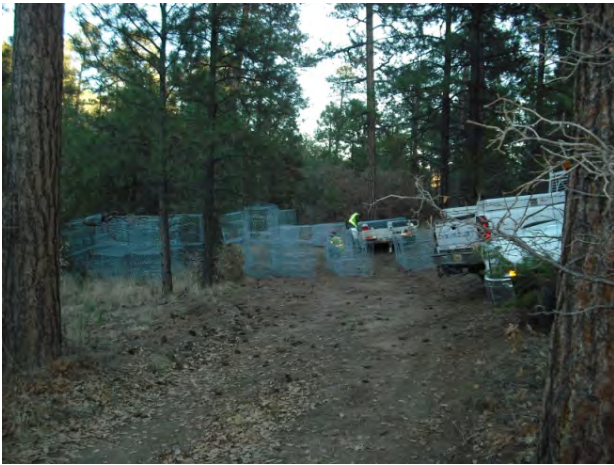
Photo 1 Gabion basket assembly area
