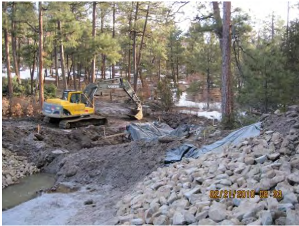
Photo 1 Flume subgrade covered with concrete blanket to keep warm and dry
