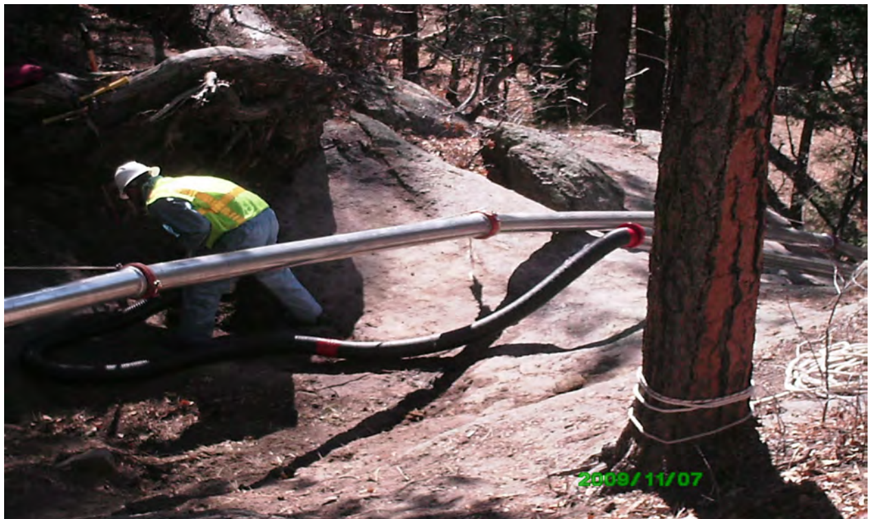
Crews vacuuming contaminated sediment from drainage
