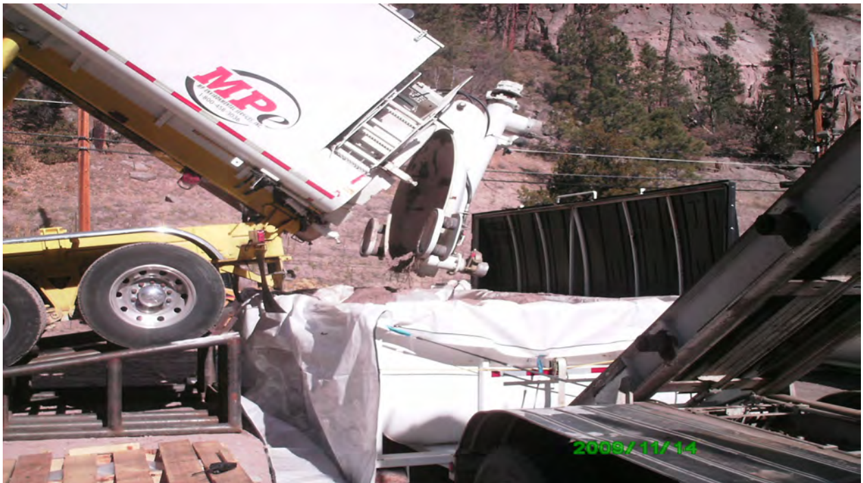
Vacuum truck emptying sediment into rolloff bin
