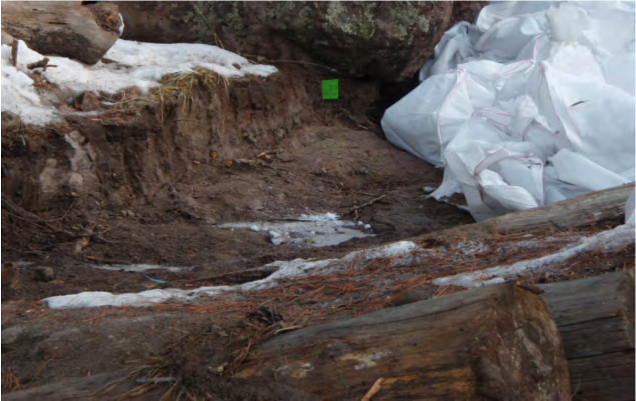
Confirmation sampling location within drainage and bags of excavated rock
