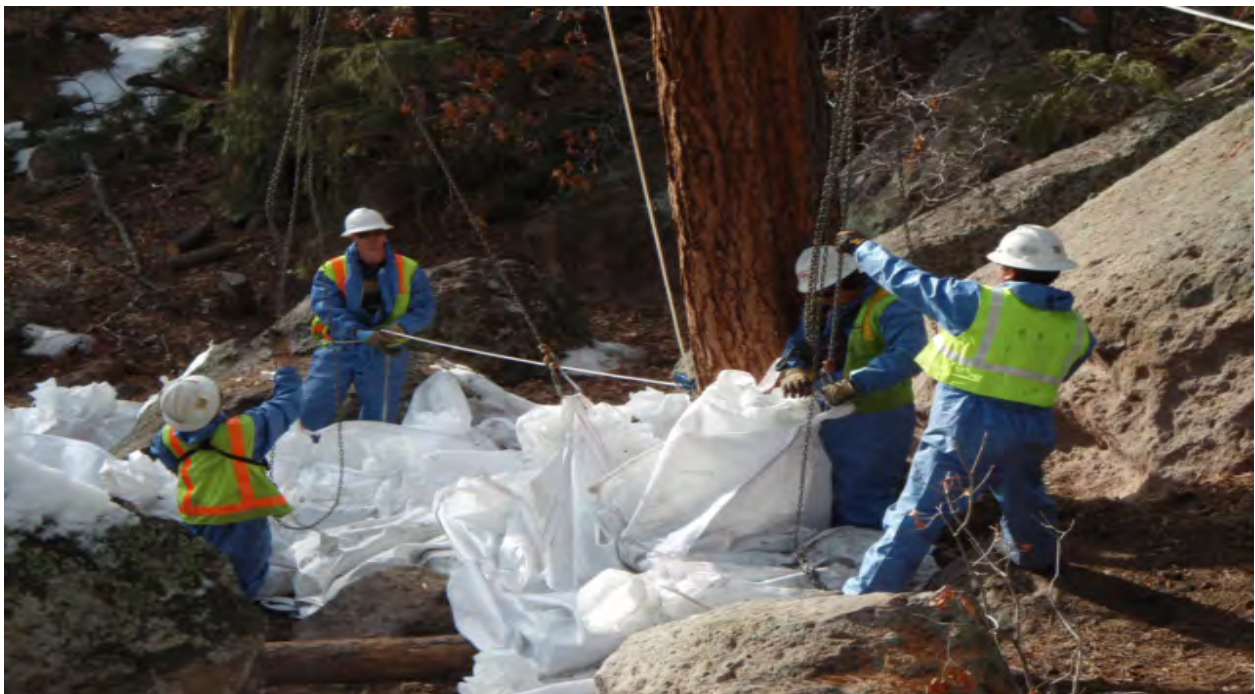
Crews loading bags of excavated rock onto slip line within drainage
