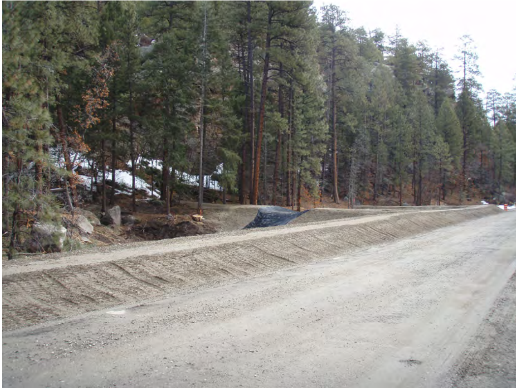
March 2010, looking downcanyon at retention pond berms
