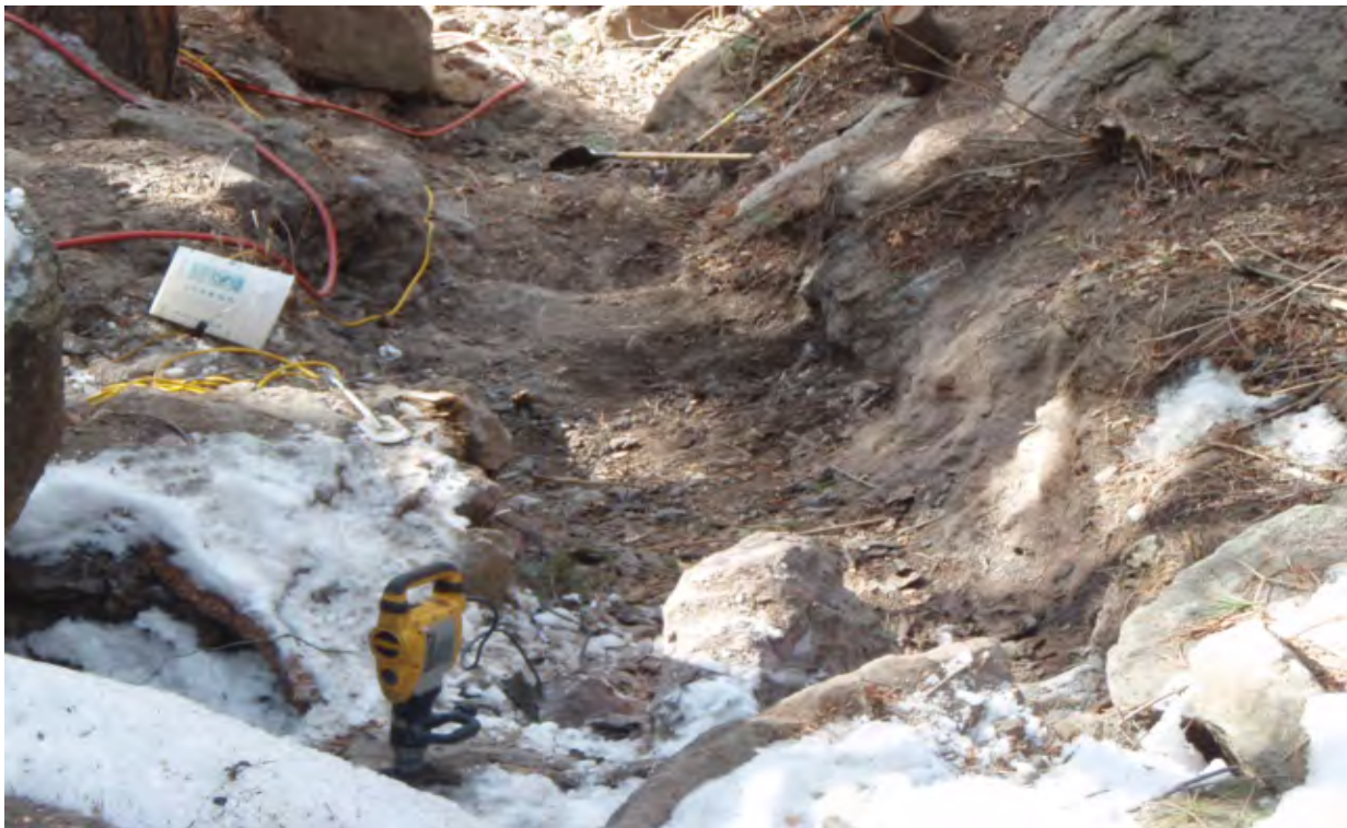
View of drainage during rock removal activities
