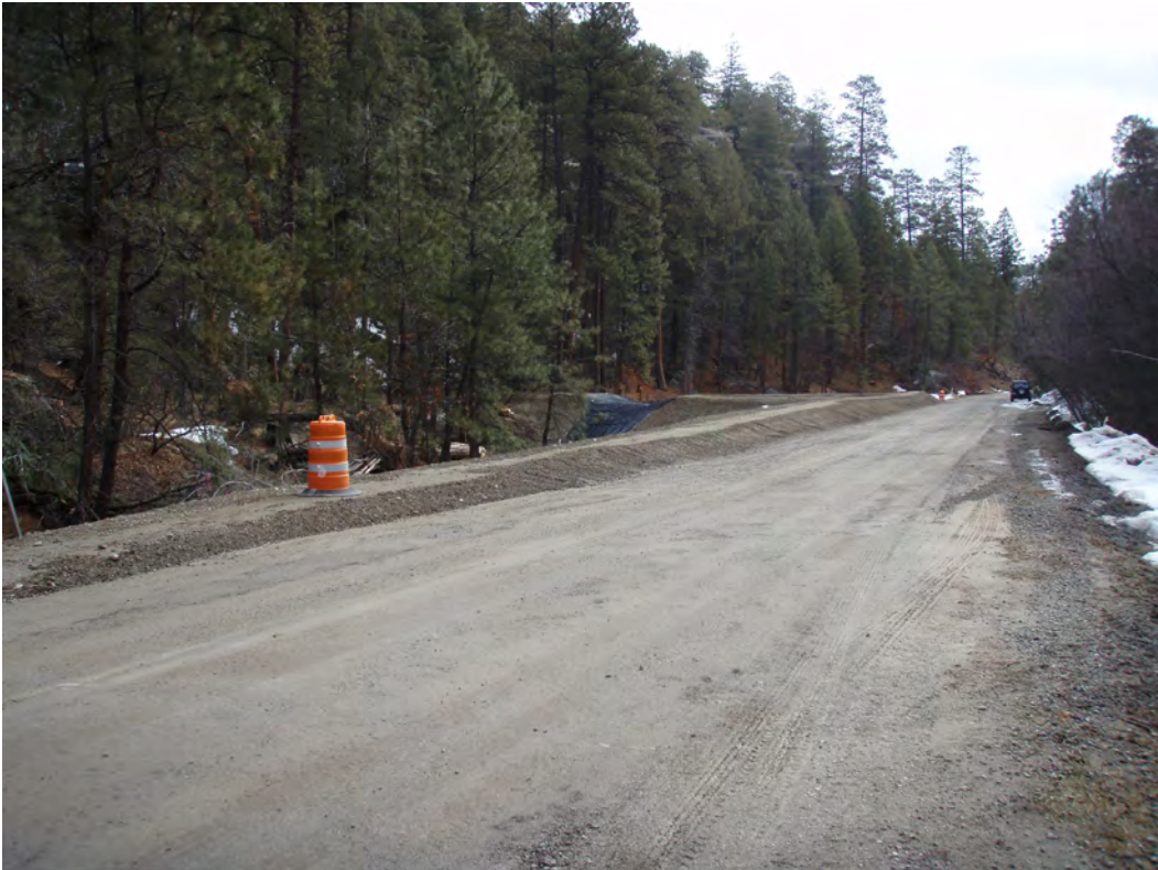
March 2010, looking downcanyon at retention pond berms
