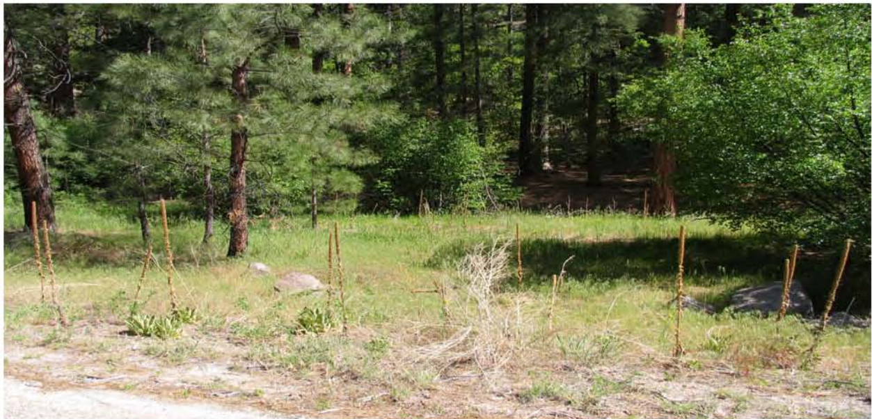
Sediment deposition area at base of drainage, looking north
