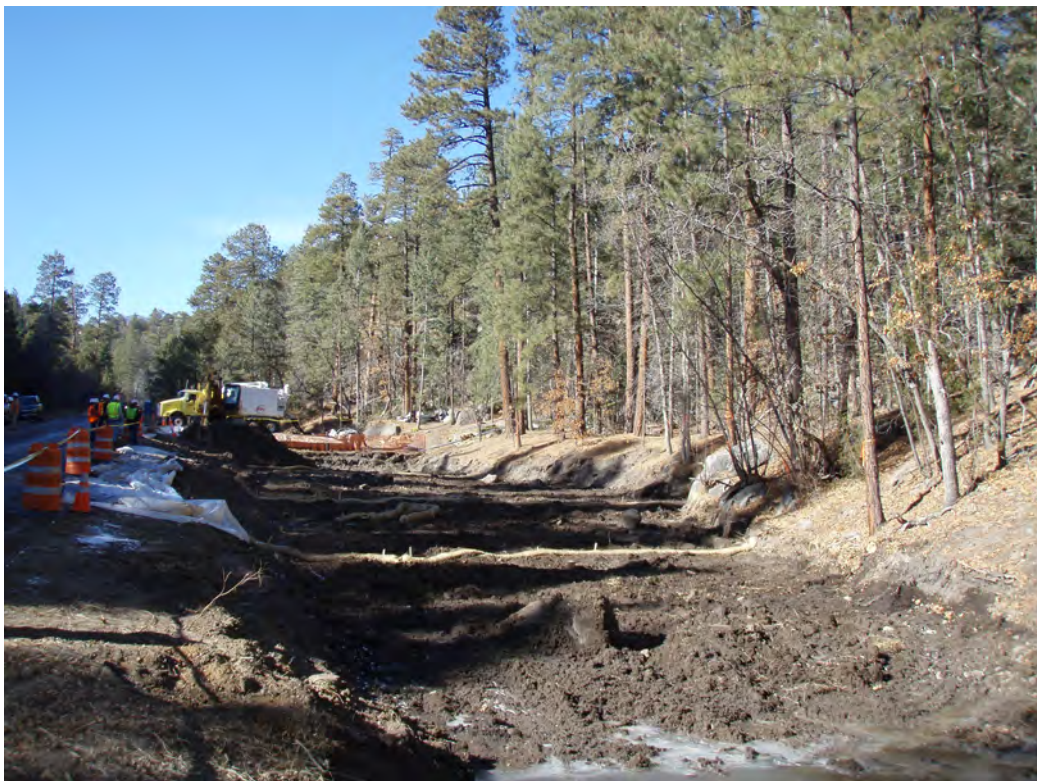
December 2009, looking upcanyon at excavation
