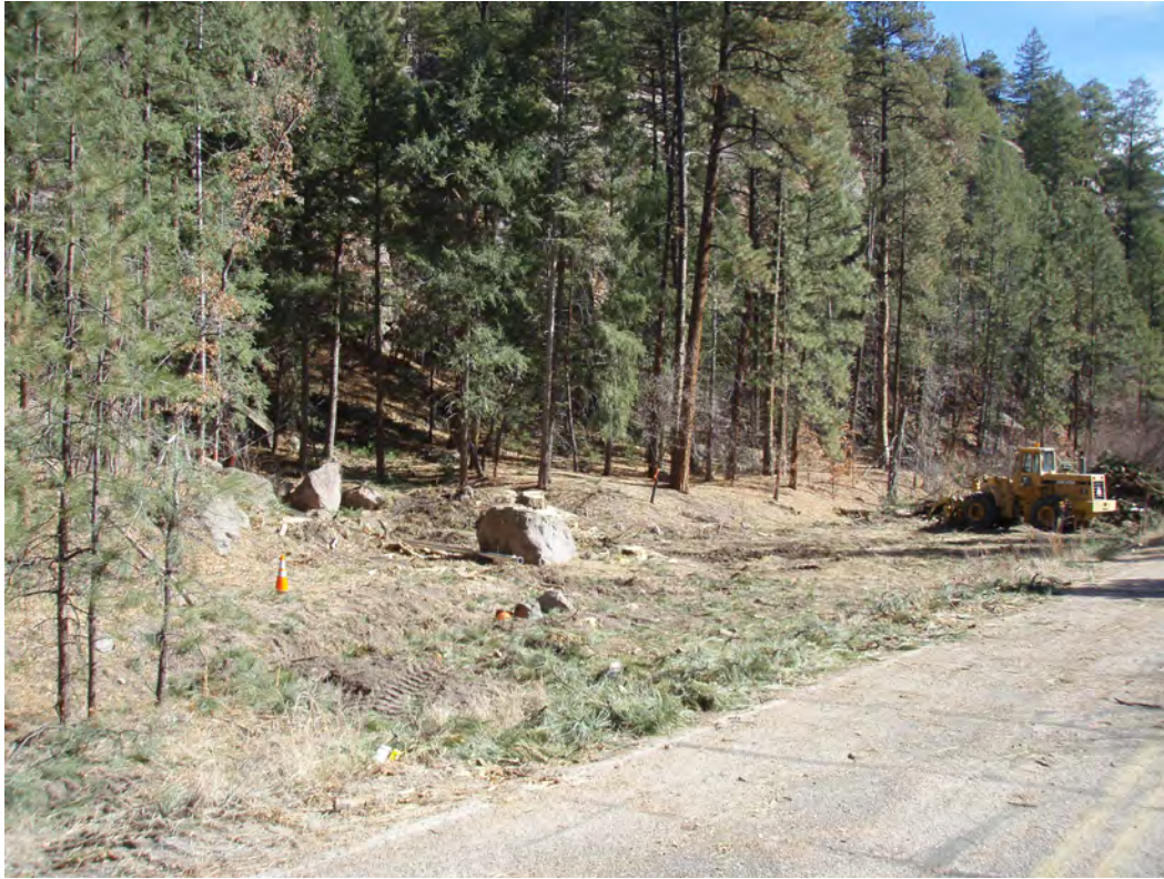
November 2009, looking downcanyon at brush/tree removal before pond construction
