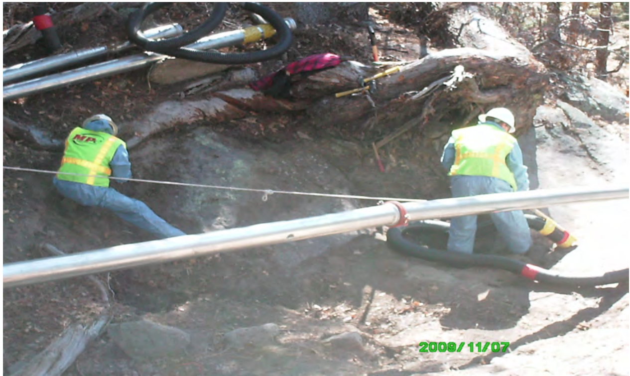
Crews vacuuming contaminated sediment from drainage
