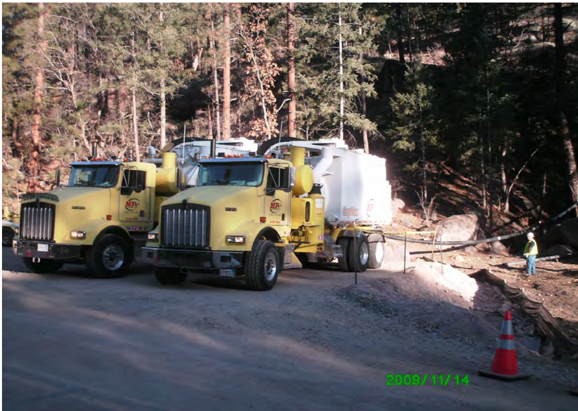
Vacuum truck staged in canyon bottom at base of drainage
