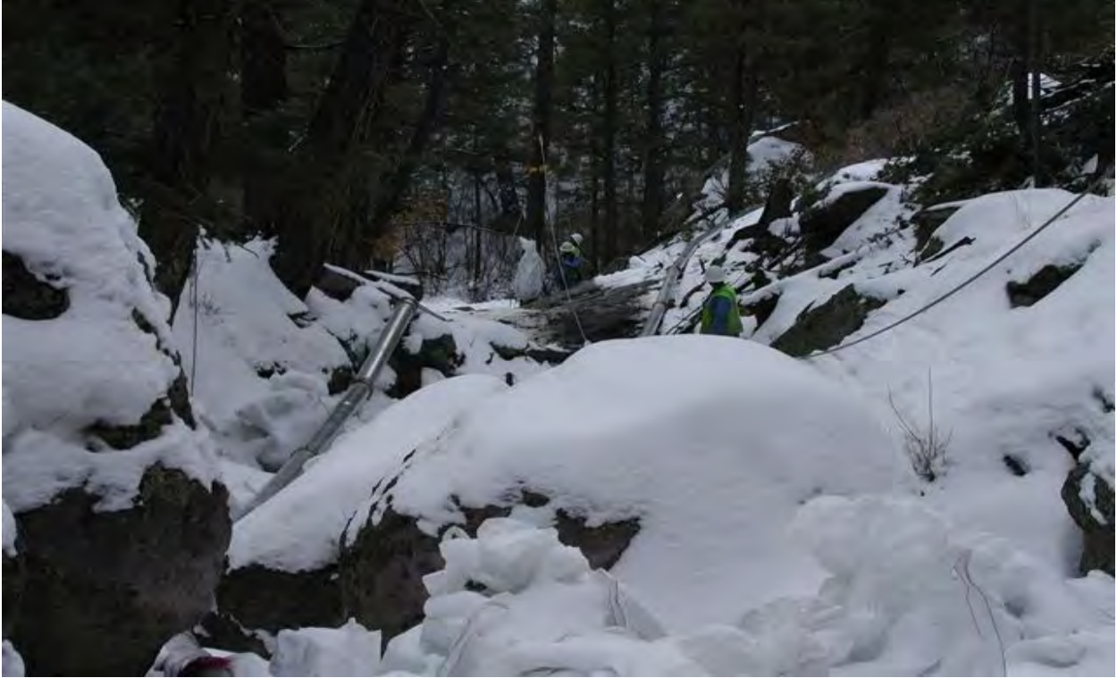
Crews setting up slip line within drainage following snow storm
