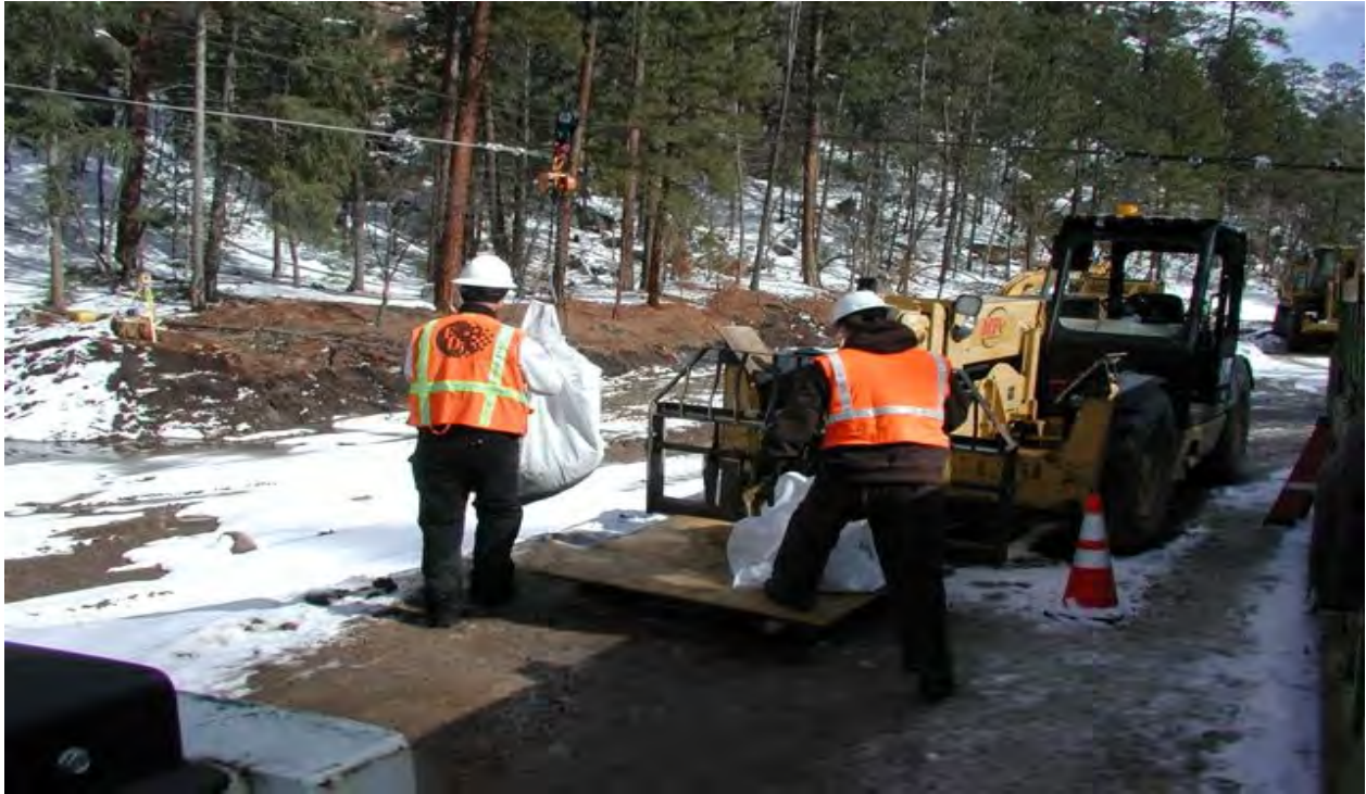
Bags of excavated rock off-loaded from slip line
