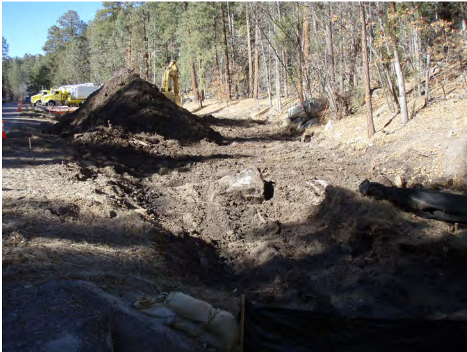
November 2009, looking upcanyon at excavation of soil in the deposition zone
