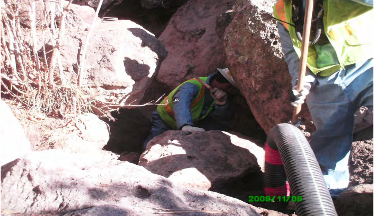
Crews vacuuming contaminated sediment between boulders in drainage
