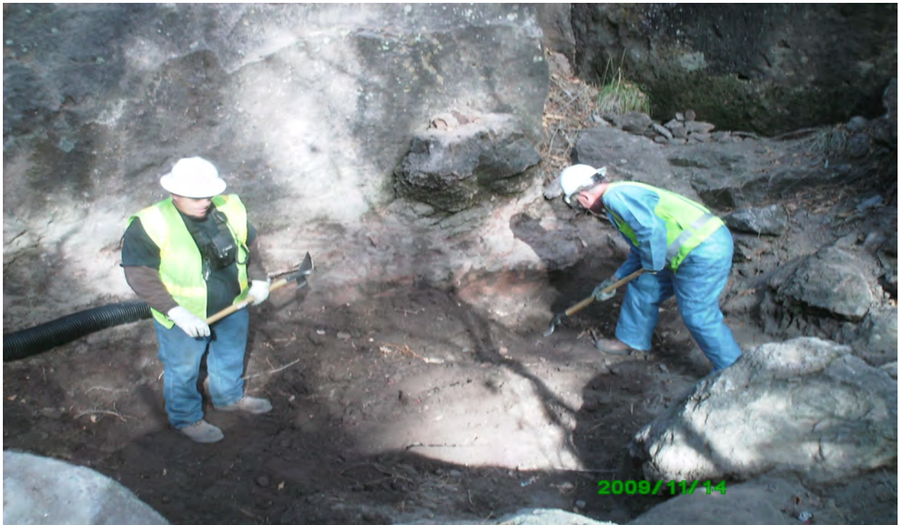
Crews vacuuming contaminated sediment from drainage
