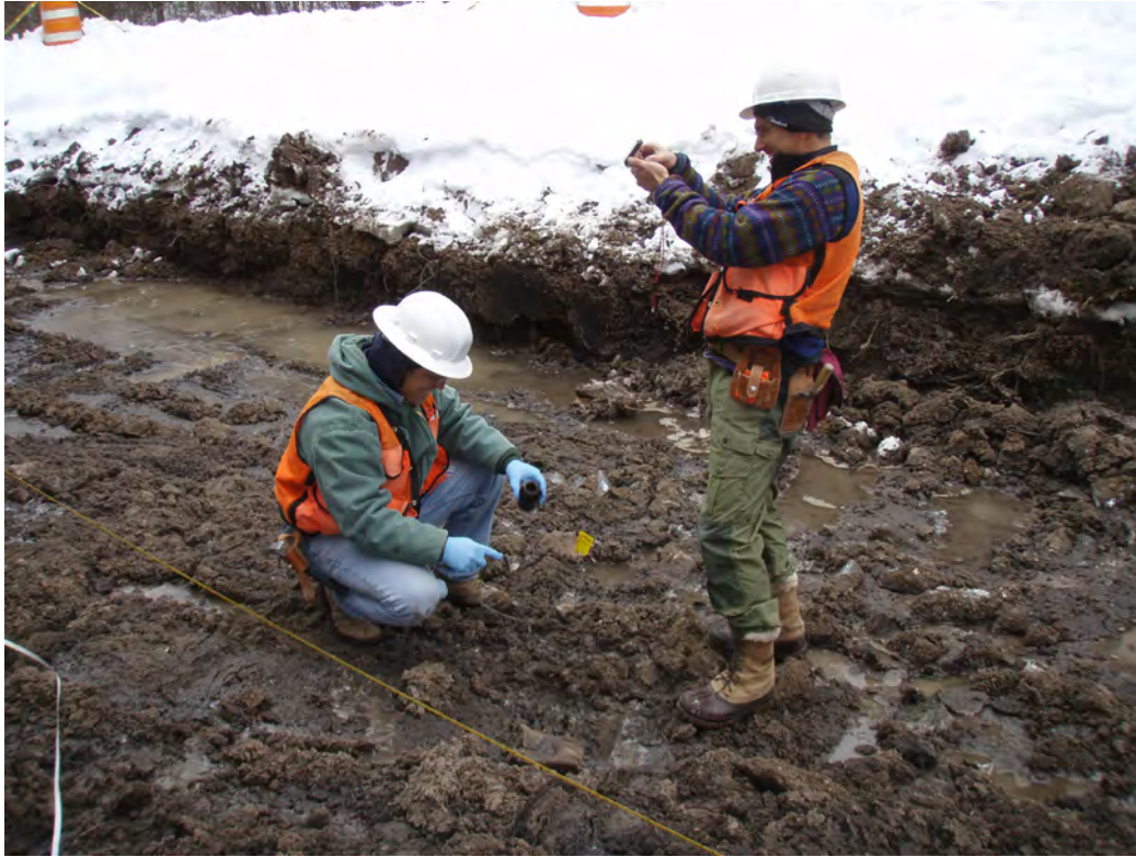
December 2009, collecting confirmation samples from excavation in winter conditions
