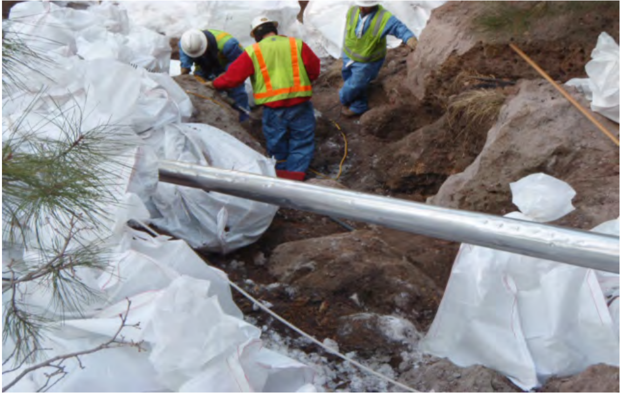
Rock removal and packaging activities within drainage
