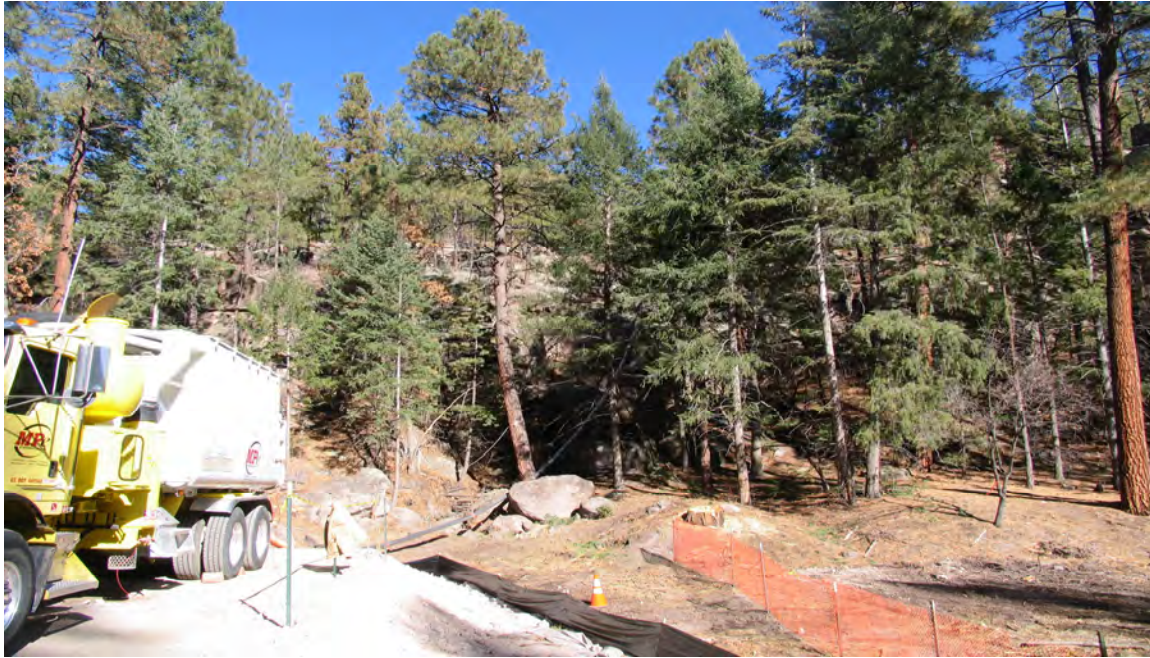
Vacuum truck staged in canyon bottom at base of drainage
