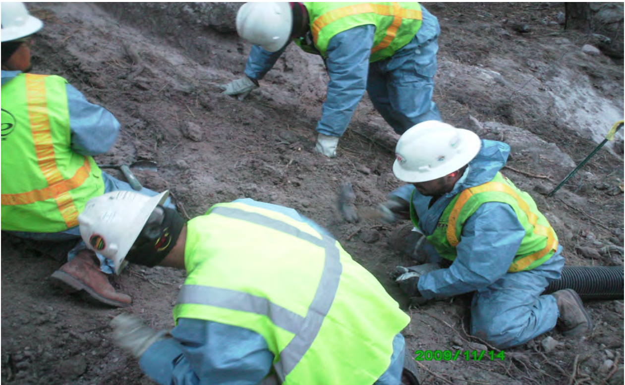
Crews vacuuming contaminated sediment from drainage
