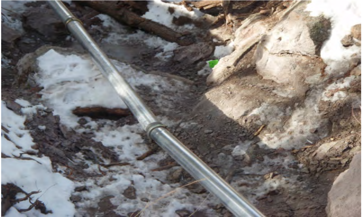
Confirmation sampling location and vacuum pipe within drainage
