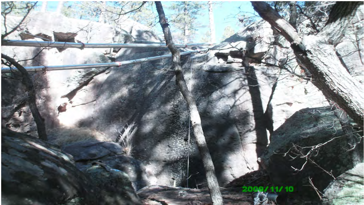
View of vacuum piping from bottom drainage
