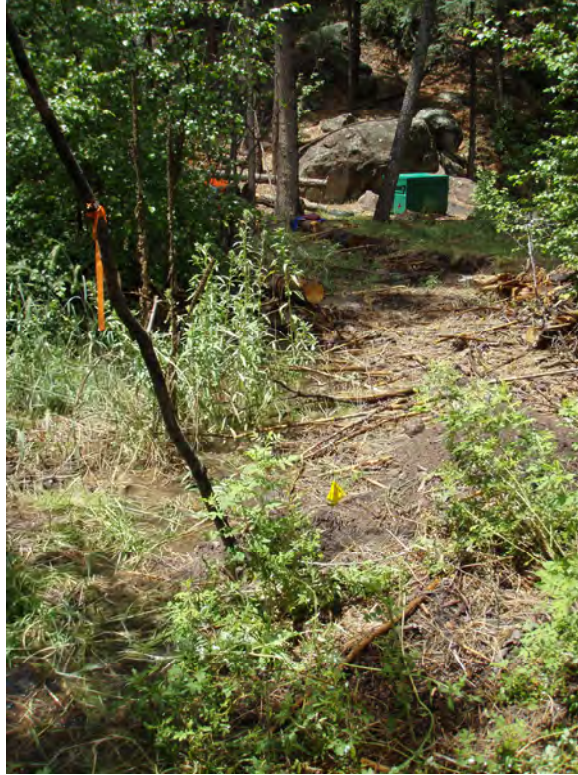
July 2009, Isco sampler in Geenlee box at west end of deposition zone. Note removal of woody debris to enhance infiltration in the deposition zone.
