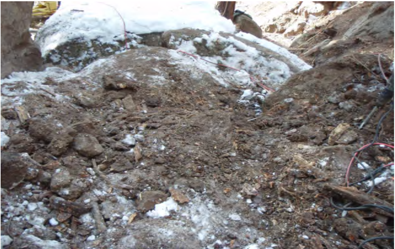
View of drainage during sediment and rock removal activities
