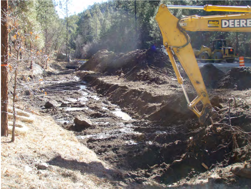
November 2009, looking downcanyon at excavation of soil in the deposition zone
