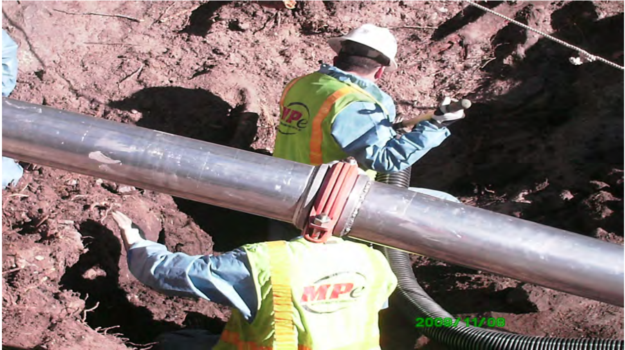
Crews vacuuming contaminated sediment from drainage
