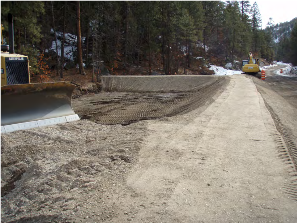
February 2010, looking downcanyon at lower retention pond berm construction
