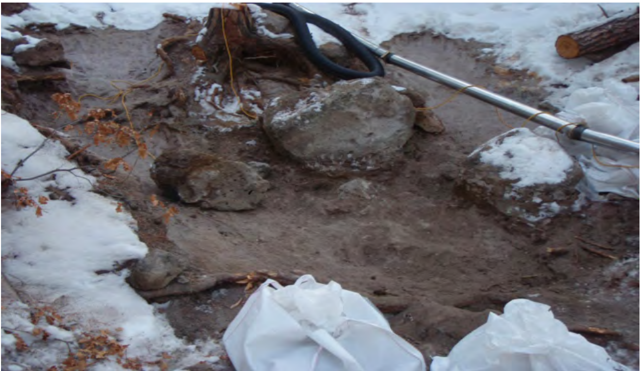
Bags of excavated rock and vacuum hose within drainage
