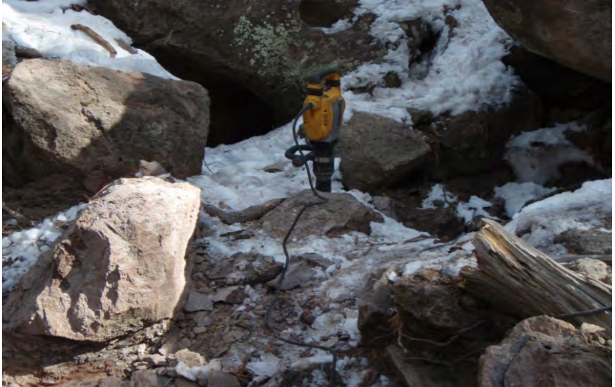
Jackhammer used to remove contaminated rock from drainage
