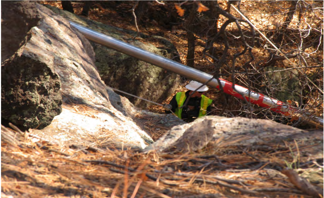
Vacuum operations within drainage
