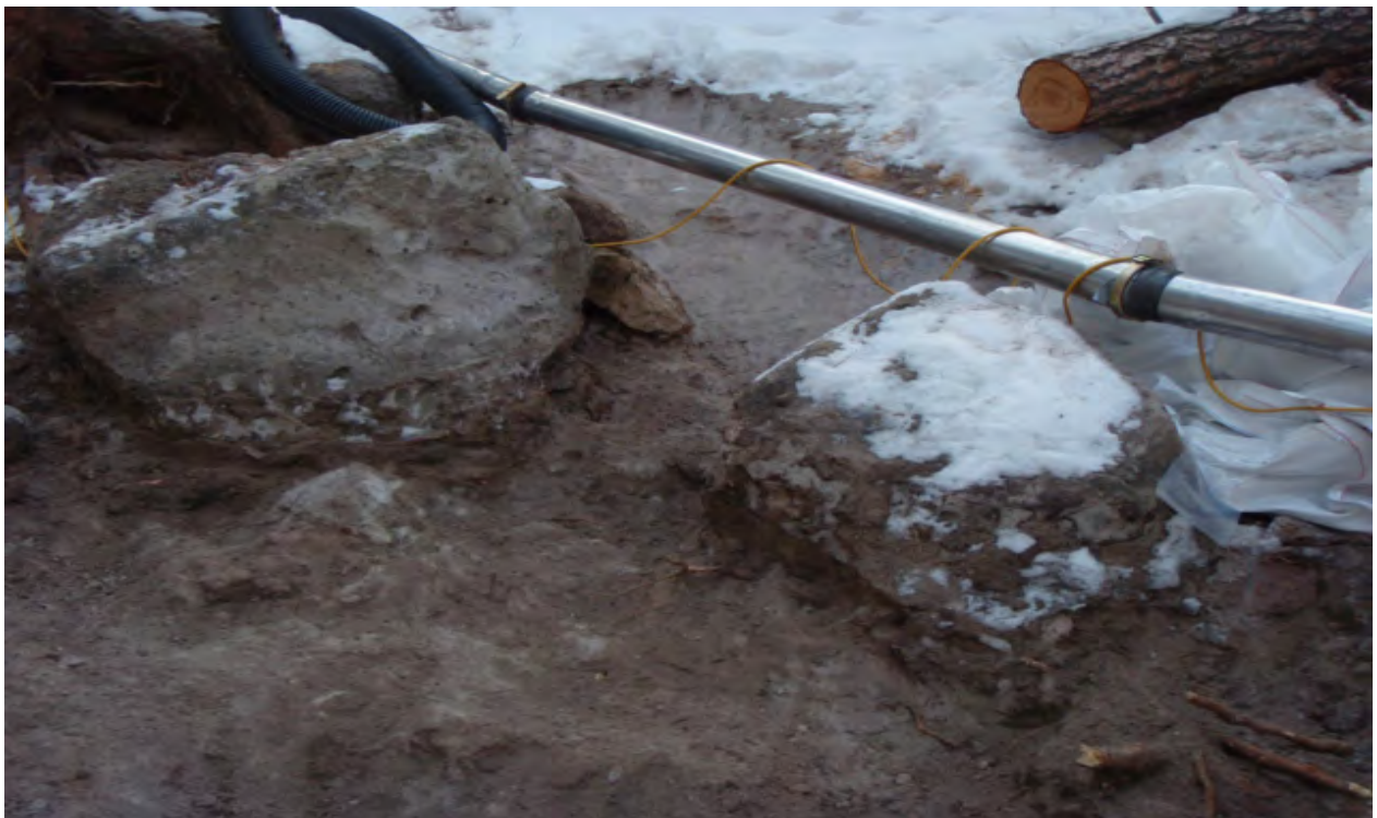
Section of drainage following sediment and rock removal
