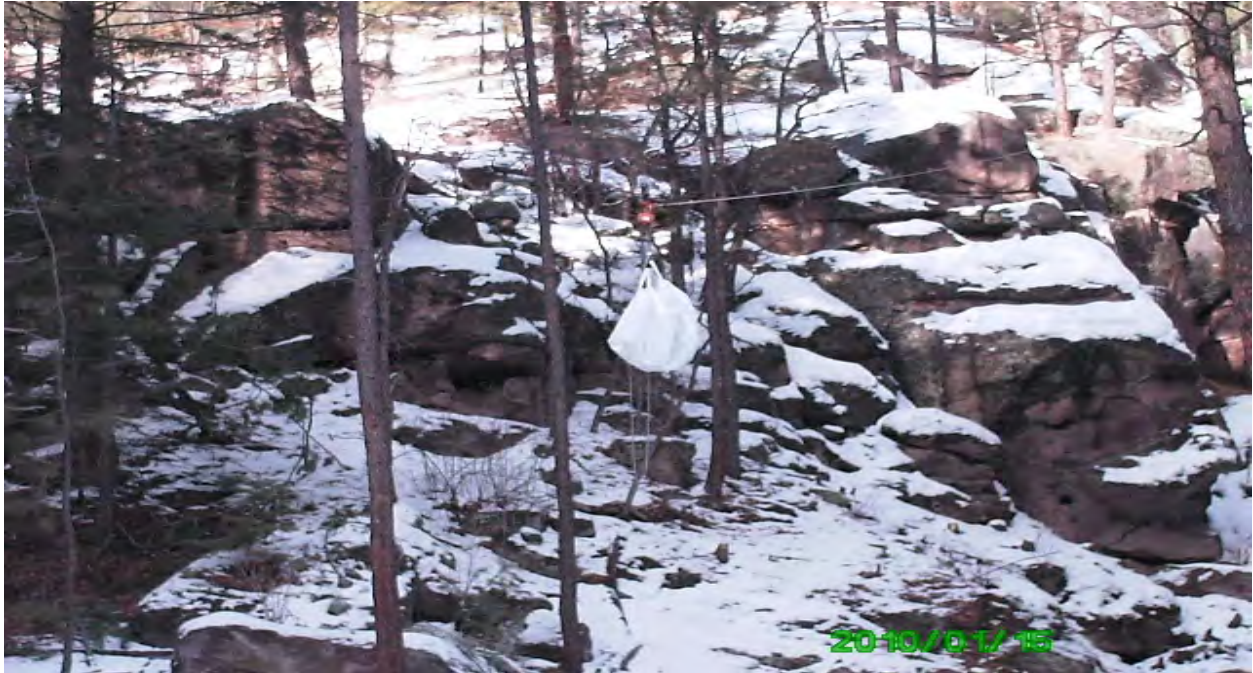
Bags of excavated rock transported on slip line
