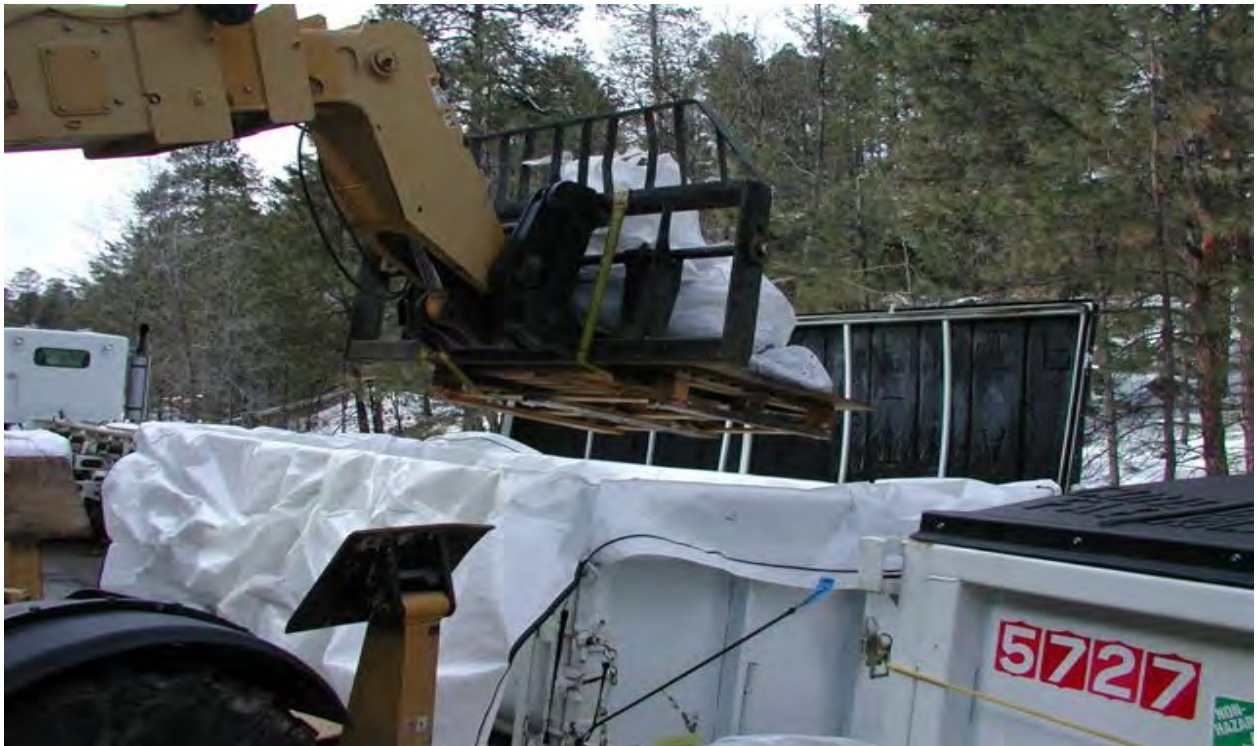
Bags of excavated rock placed into rolloff bin
