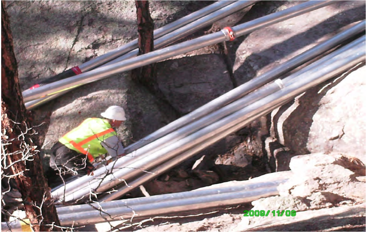
Crews setting up vacuum piping within drainage
