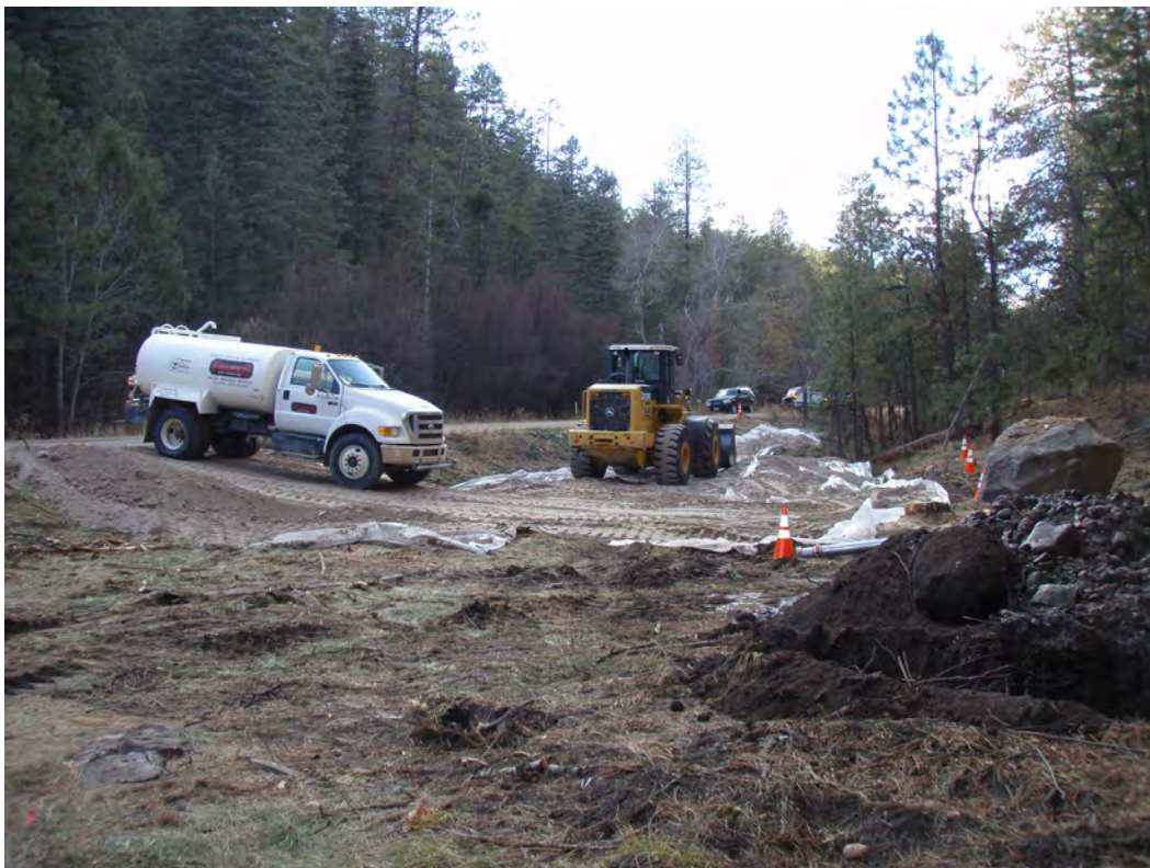
November 2009, initial pad construction for vacuum truck
