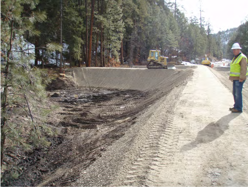
February 2010, looking downcanyon at upper retention pond berm construction
