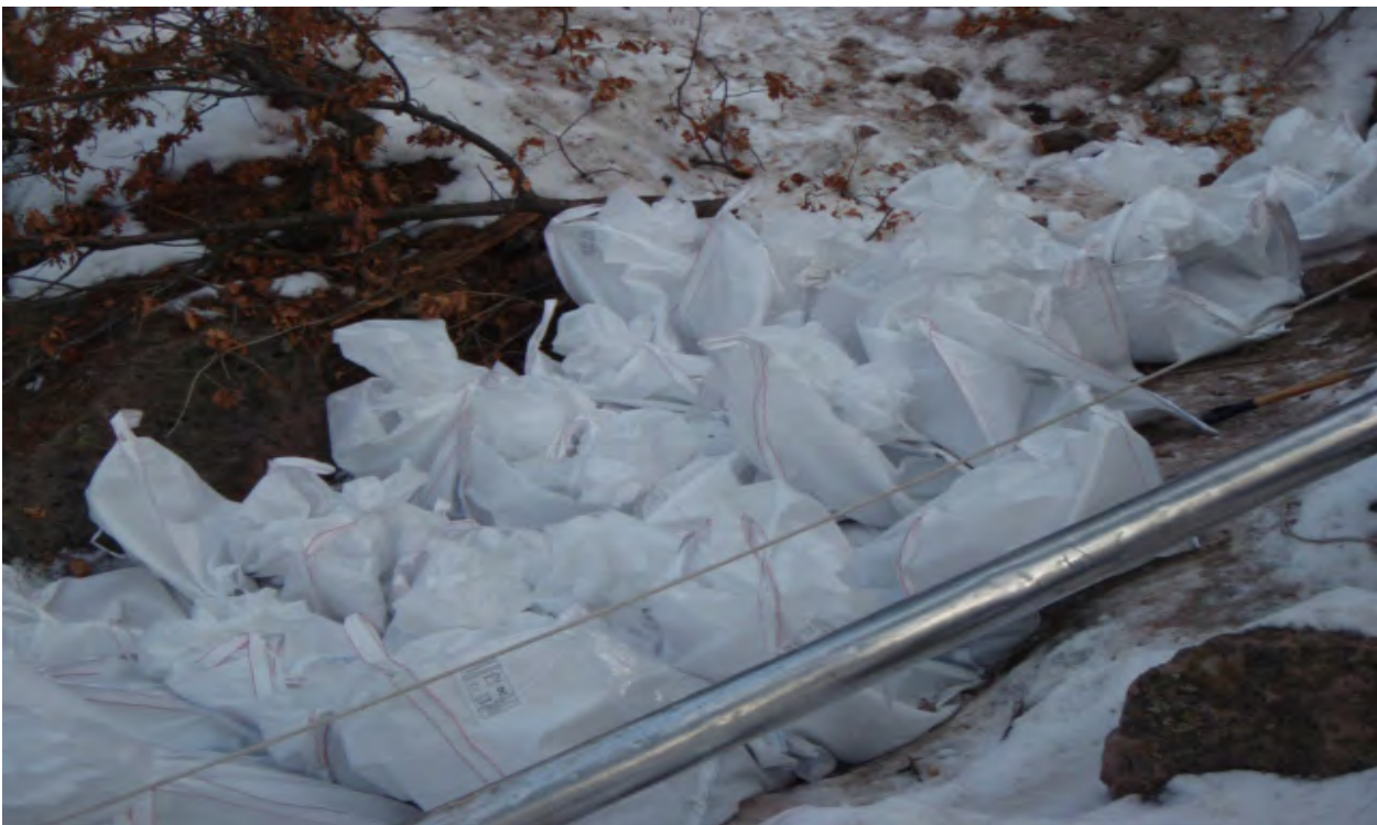
Bags of excavated rock staged with drainage next to vacuum pipe
