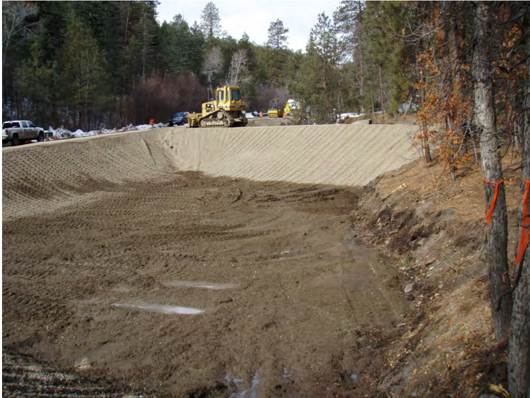
February 2010, looking upcanyon from lower berm to upper berm
