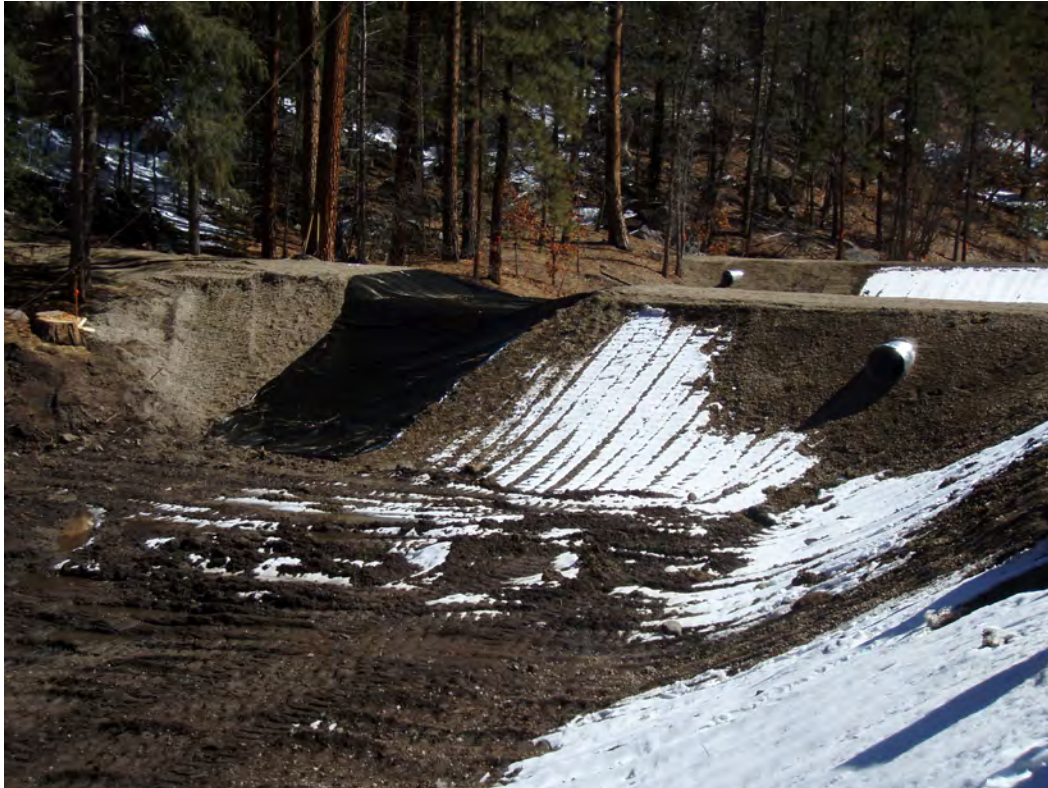
February 2010, looking downcanyon at upper retention pond spillway and overflow pipe
