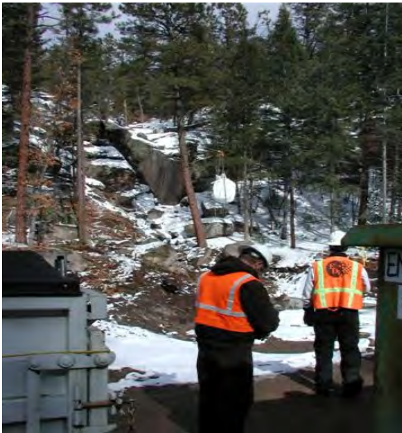
Bags of excavated rock coming down slip line to rolloff bins
