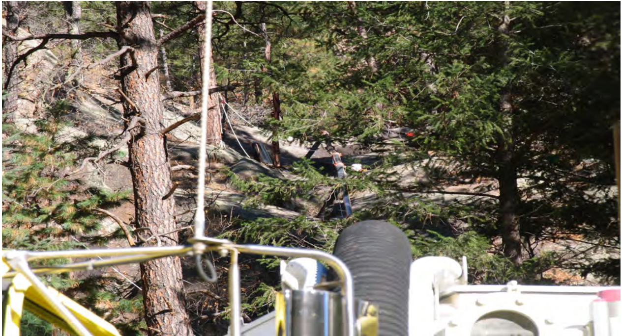
View from vacuum truck looking up to drainage from canyon bottom
