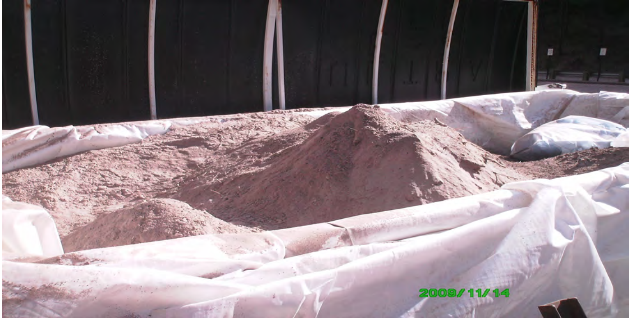
View of sediment vacuumed from drainage in rolloff bin
