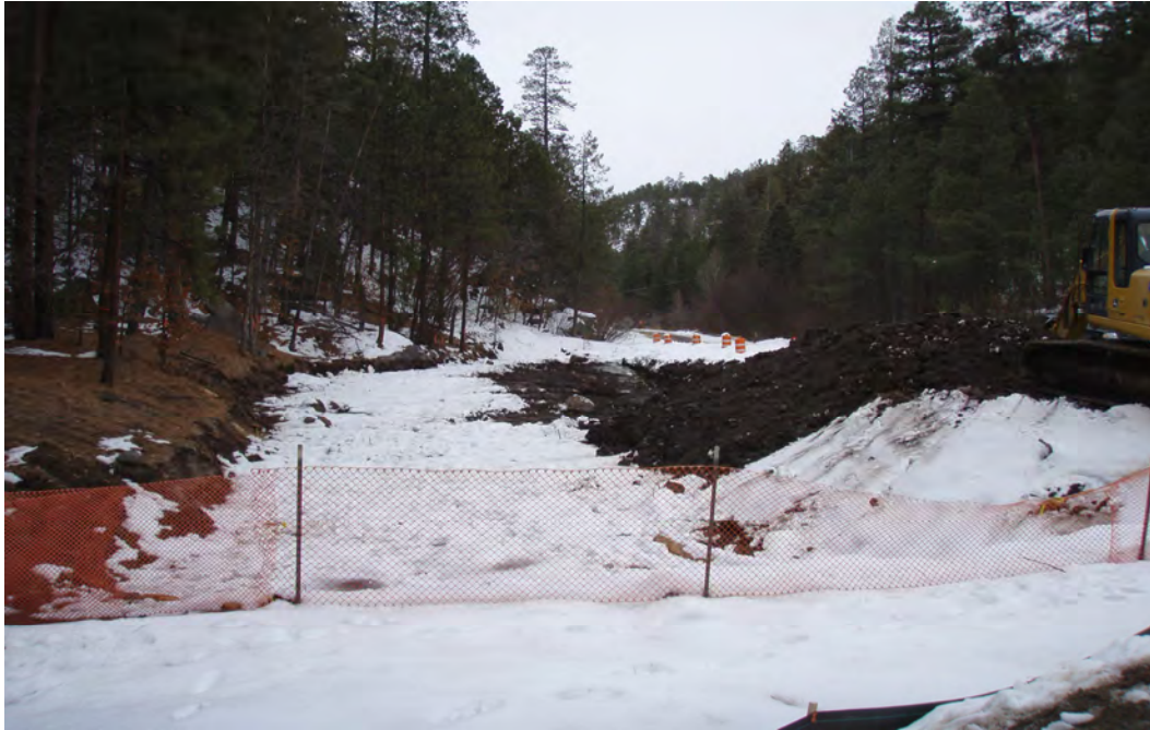
December 2009, view of excavated canyon floor drainage
