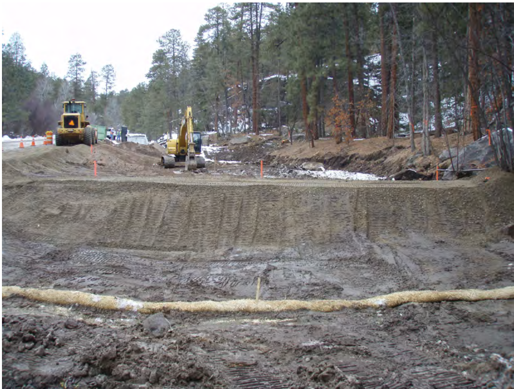
January 2010, temporary earthen berm built before construction of the retention pond berms
