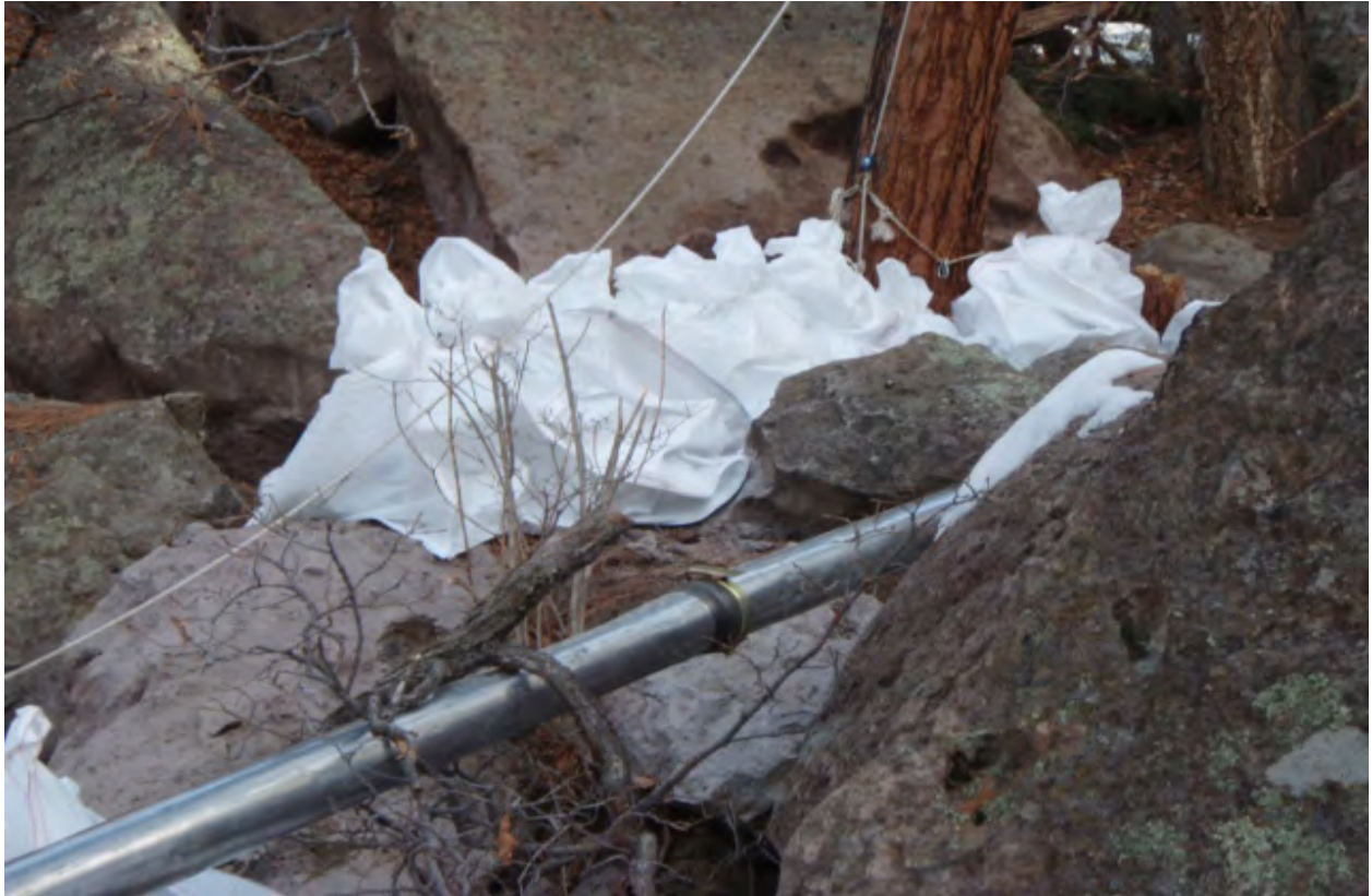
Bags of excavated rock staged along drainage adjacent to vacuum line
