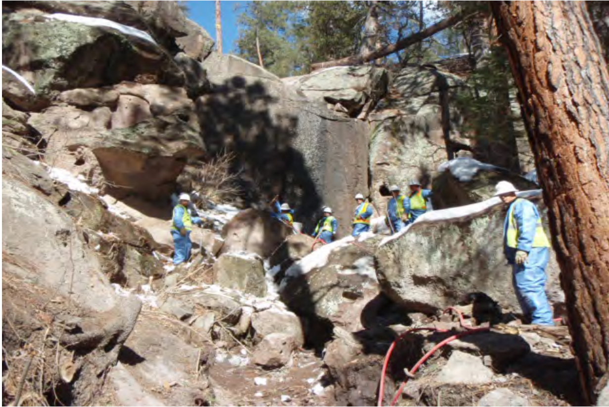
Crews removing contaminated rock from drainage using jack hammers
