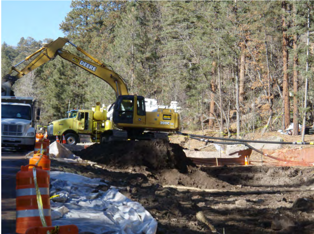
December 2009, excavation of soil into dump truck
