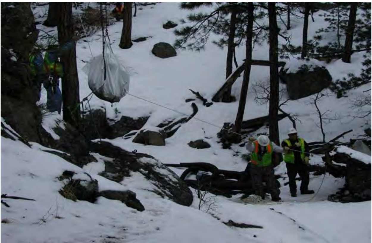
Bags of excavated rock coming down slip line in snowy conditions
