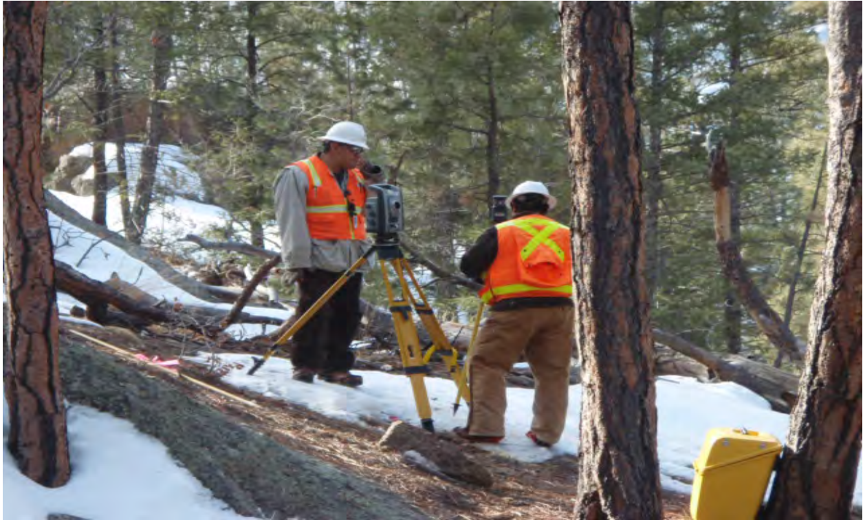
Surveying drainage and confirmation sampling locations
