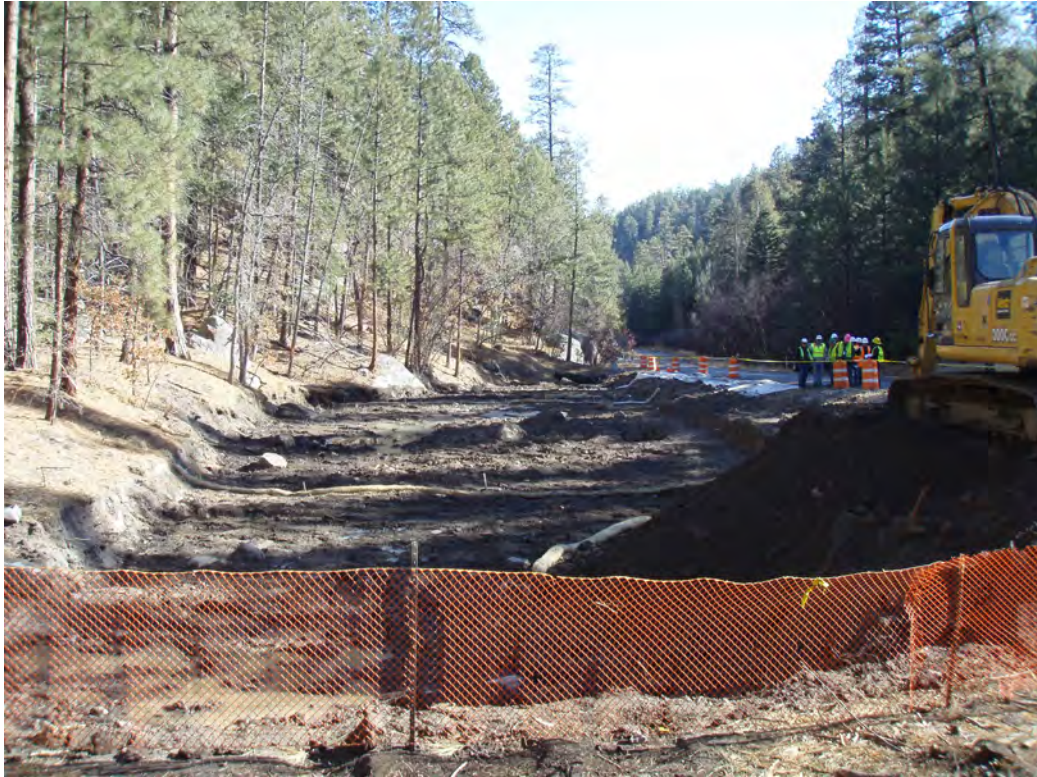
December 2009, looking downcanyon at excavation
