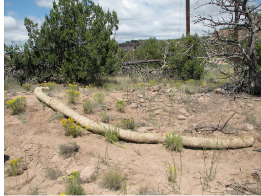
LA 21622 after wattle installation
