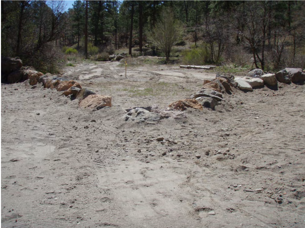
Figure 2 Pueblo Canyon cross vane 2 looking eastward (downcanyon). Note that the vertex is at the elevation of the stream bed, and the gaps in large rocks are filled.
