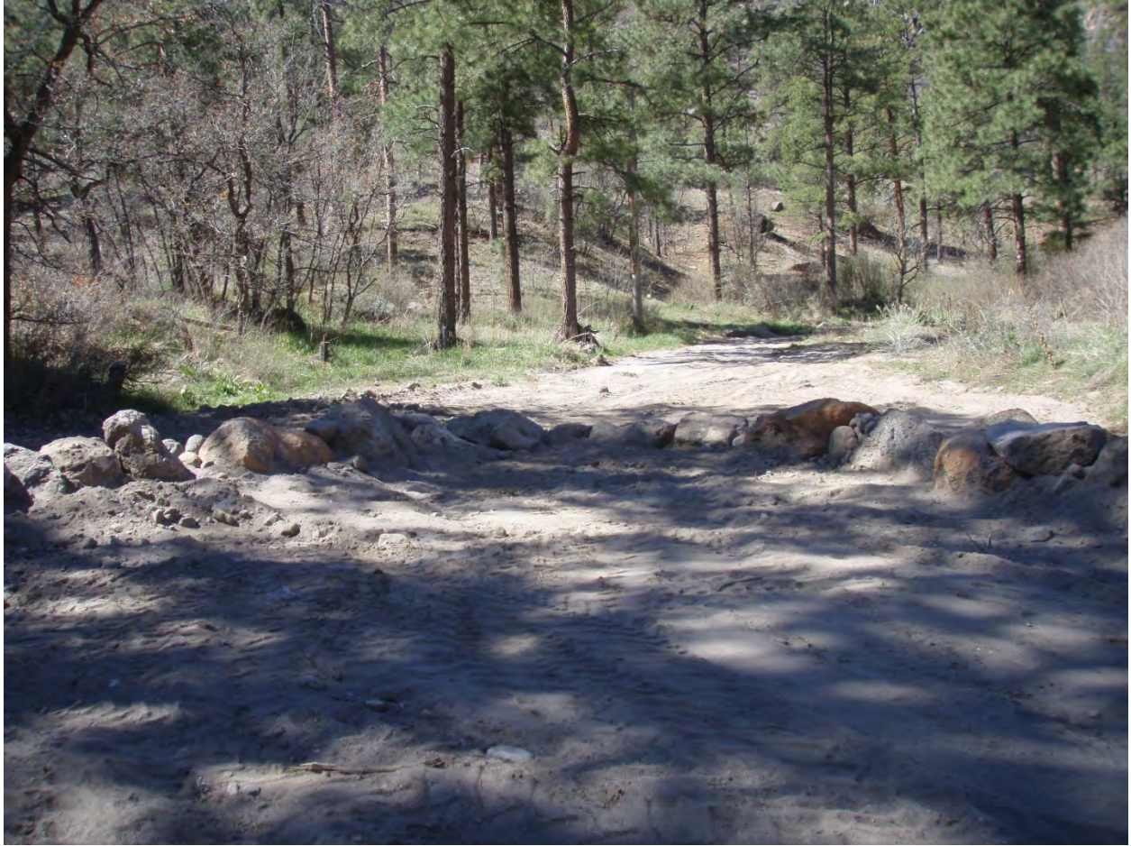
Figure 3 Pueblo Canyon cross vane 3 looking westward (upcanyon). Note that the vertex is at the elevation of the stream bed, and the gaps in the large rocks are filled.
