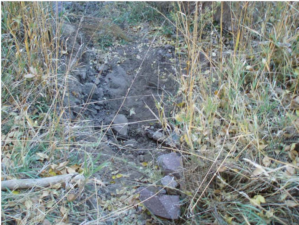
Figure 4.2-5 Before and after photographs of large asphalt boulder in the drainage removal
