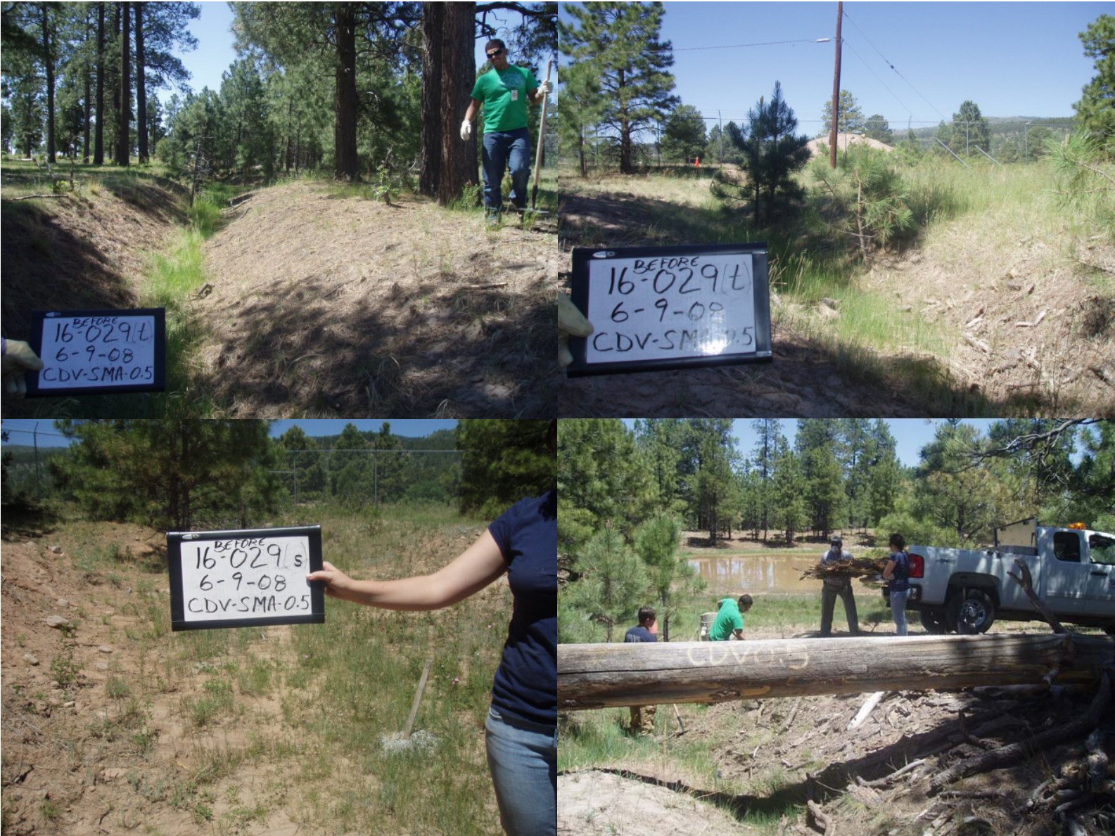
Figure 1 Drainages into the 90s Line Pond before best management practice (BMP) installation
