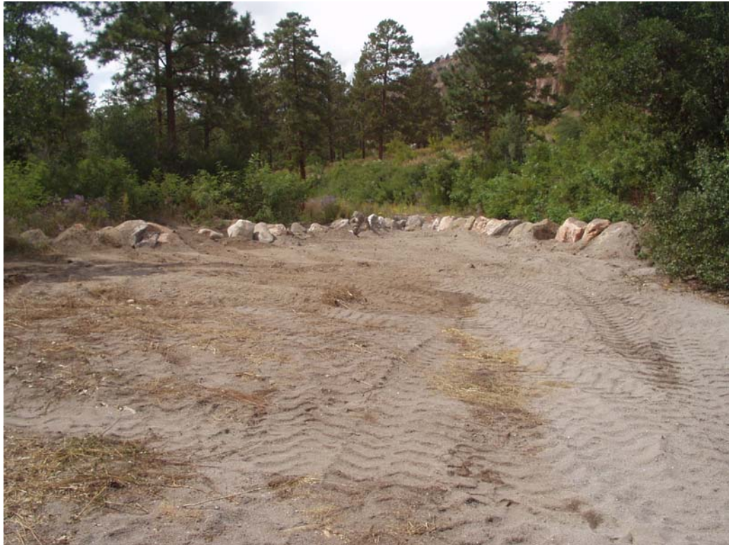
Figure 3b View looking upcanyon at the lower cross-vane structure
