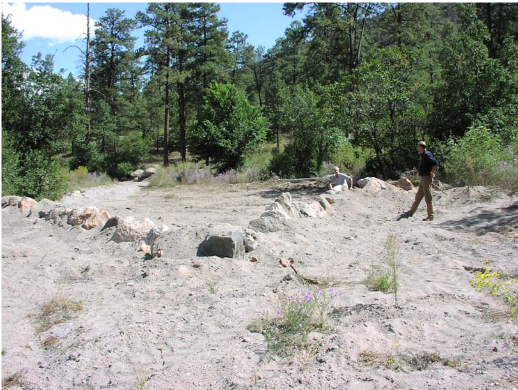
Figure 2b View looking downcanyon at the middle cross-vane structure
