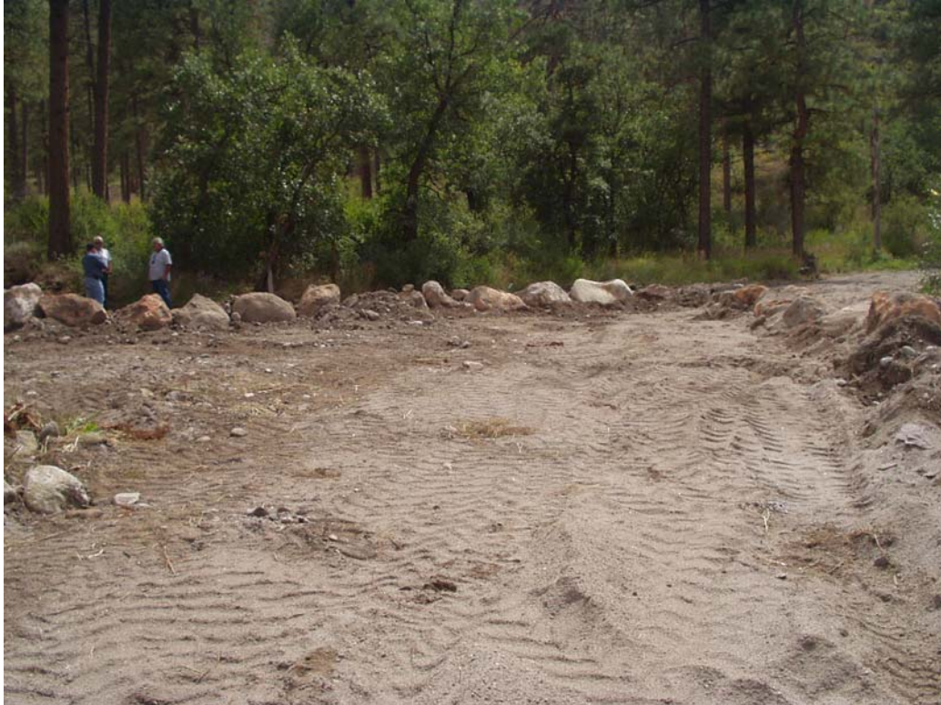
Figure 2a Upcanyon view of the middle cross-vane structure
