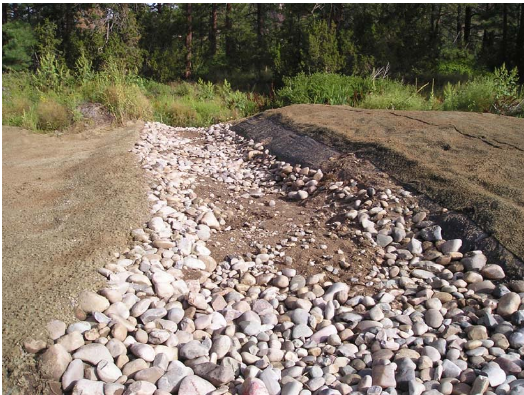
Figure 4 View looking upgradient along wing ditch after stabilization and hydromulching
