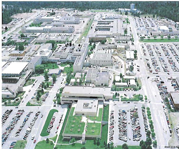
Figure 3. TA-3 in 1991; the CMR Building is located in the upper left
