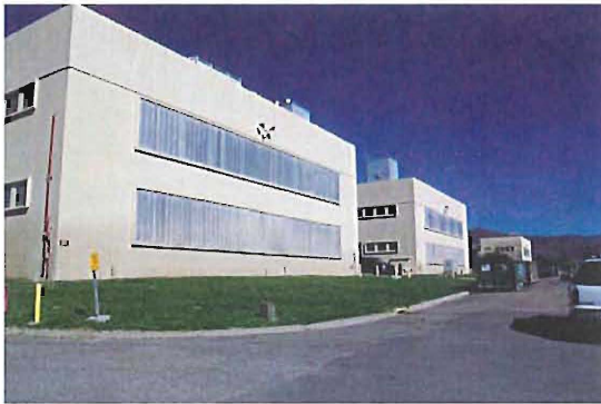
East side of Wings 7, 3, 2 (near to far) looking north (note: silver colored panels are blow-out panels)
