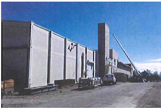
South side of Wings 9 (near with stack) and 7 (far) looking east
