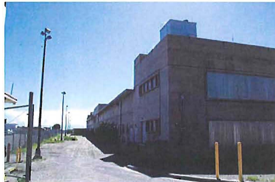
View of northwest corner looking along north wall to the east
