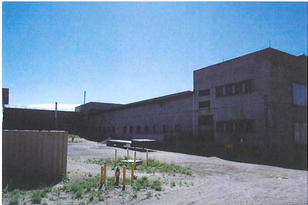
Area between Wing 1 and Wing 5 (right), facing southeast
