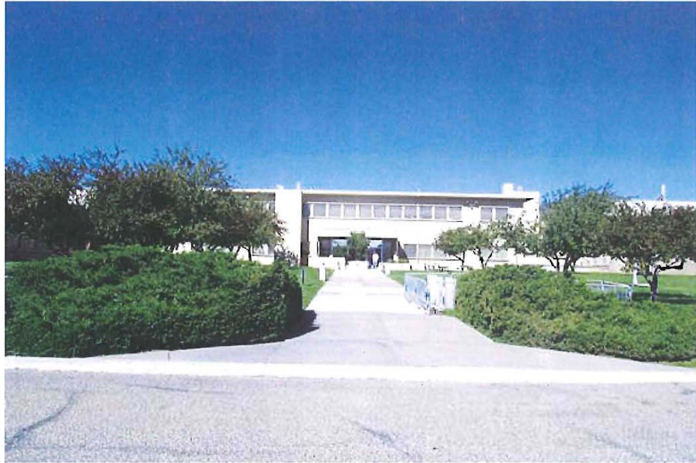
Administration Wing and main entrance, facing west
