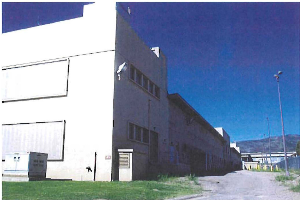
North side of Wings 2 and 4, facing west southwest
