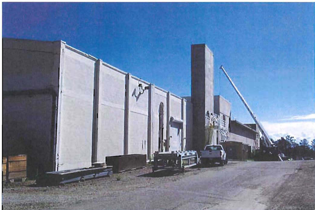
South side of Wings 9 and 7, facing east northeast
