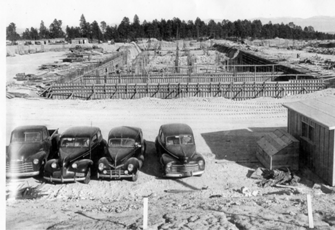
1949 CMR Construction Site
