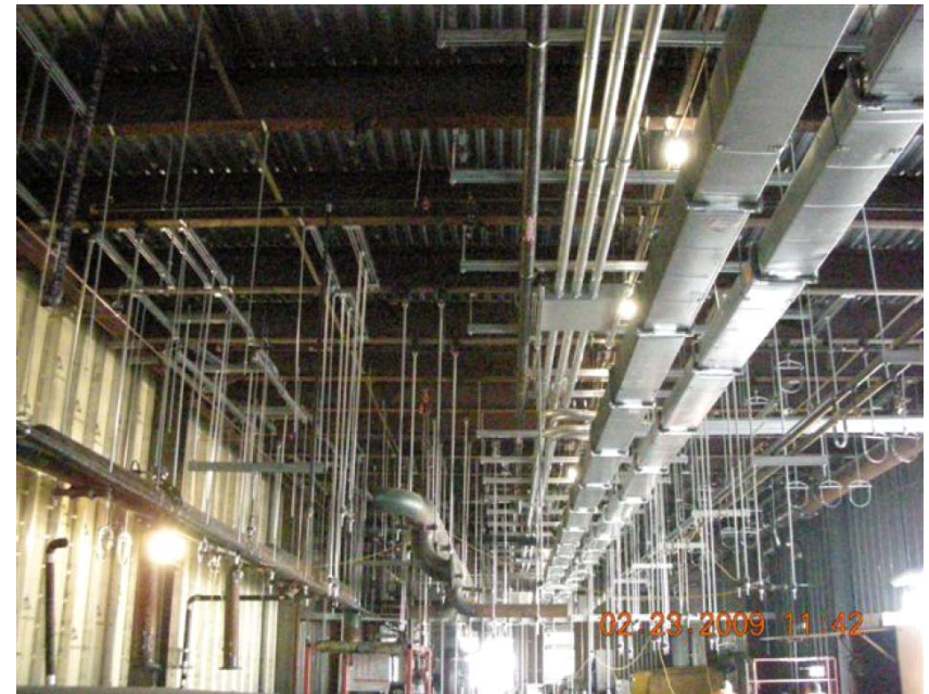
2 nd Floor Central Utility Building – Installation of Duct and Large Bore Pipe
