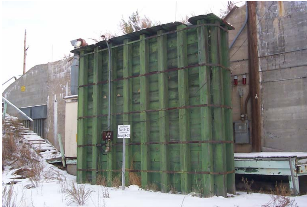
Figure 10. TA-8-3 (green barricade and stairs to be removed)
