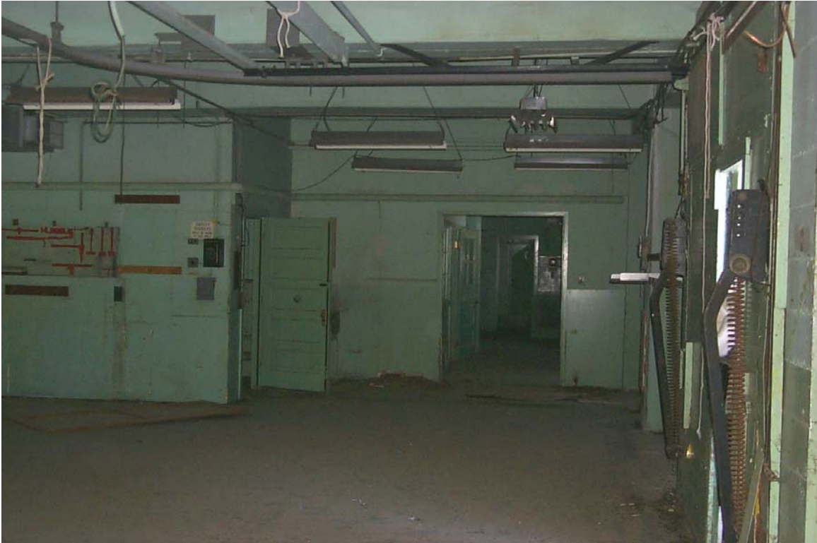
Figure 5a. Interior TA-8-1, current Room 5 looking west towards current Room 3
