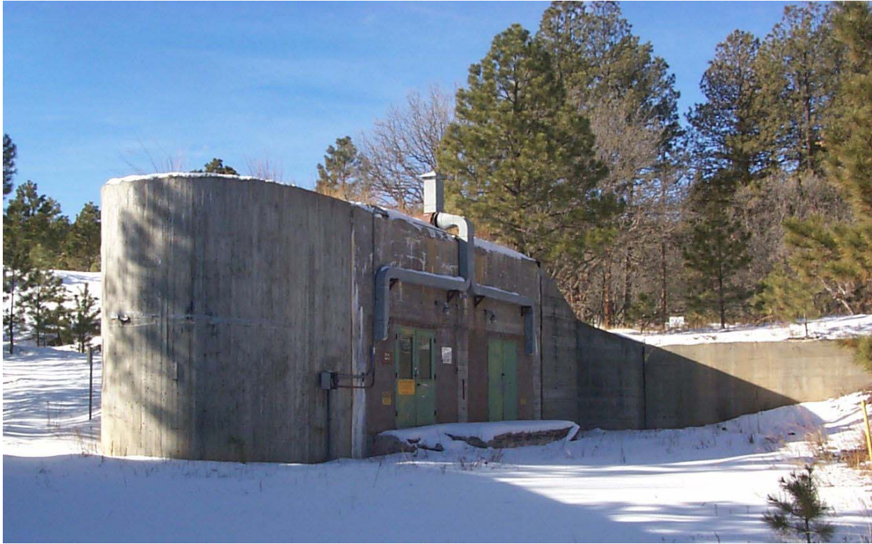
Figure 6b. Exterior TA-8-2
