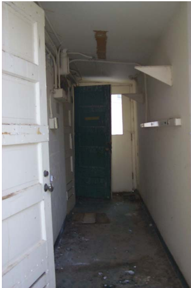
Figure 7a. Interior TA-8-3, enclosed dock
