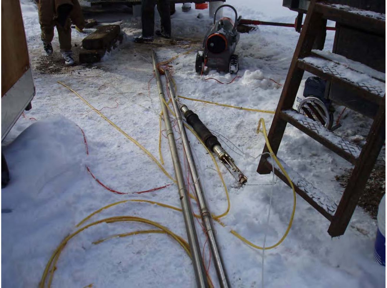
Figure 2.1-5 Extraction of Barcad sampling system components from R-33
