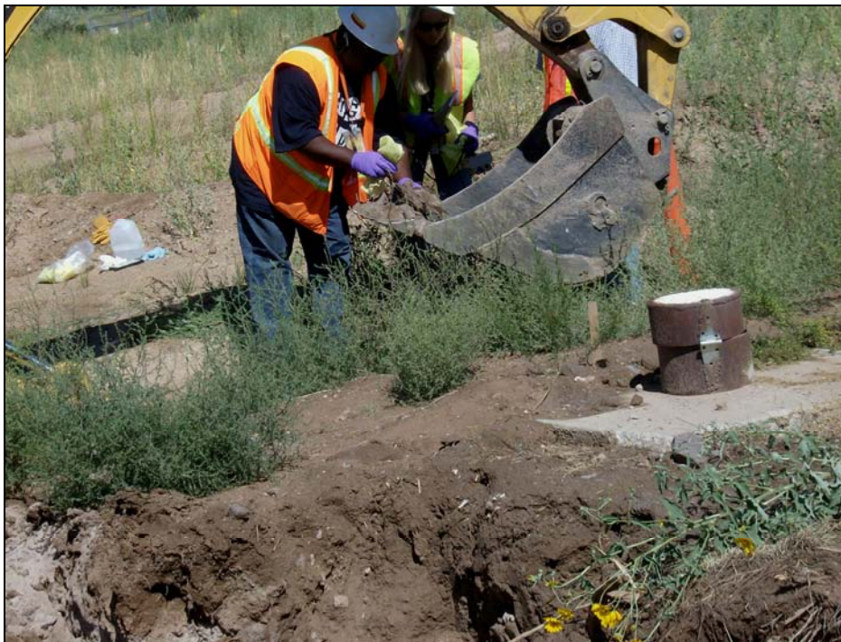
Photo 12 RCTs surveying soil in backhoe bucket during excavation, August–September 2007
