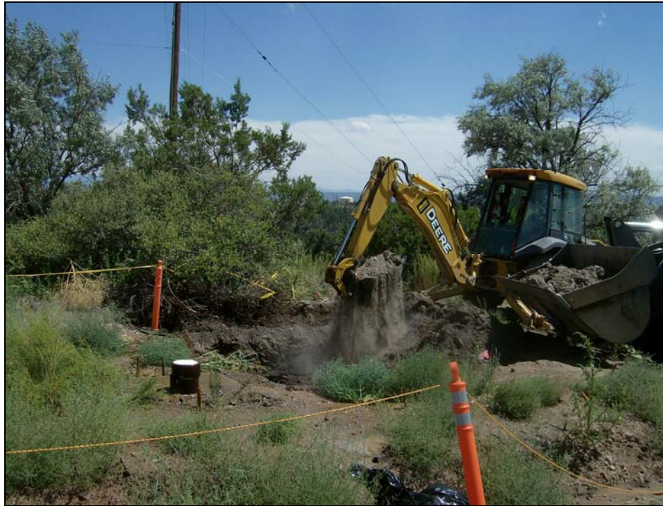
Photo 7 Excavation of elevated area of radioactivity, August-September 2007
