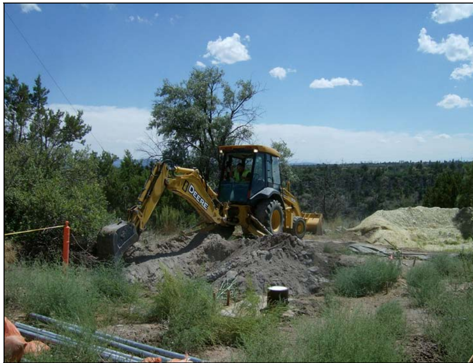
Photo 6 Excavation of area of elevated radioactivity, August–September 2007
