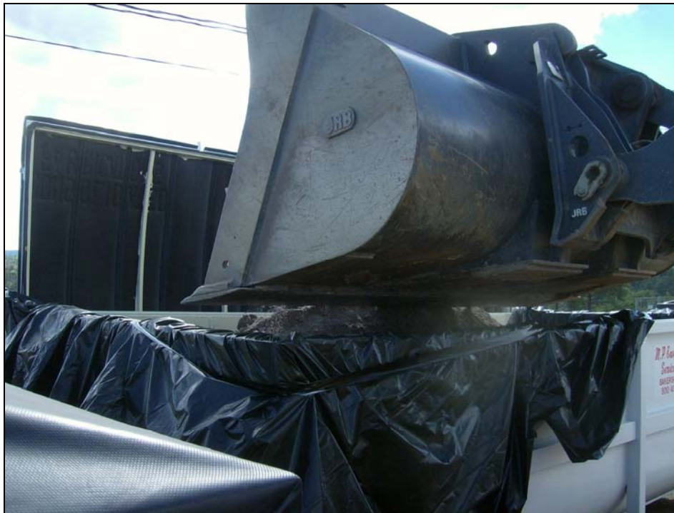
Photo 10 Front-end loader delivering removed soil to rolloff bins, August–September 2007
