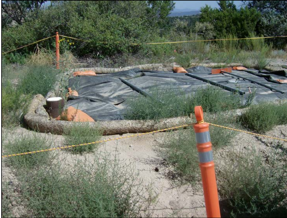
Photo 1 Area of elevated radioactivity before excavation, May 2007 (view to the east)
