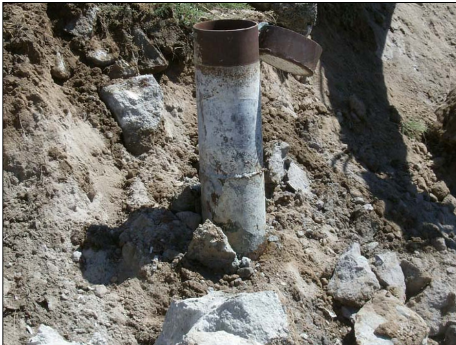
Photo 14 Exposed borehole 21-02523 in center of excavation area
