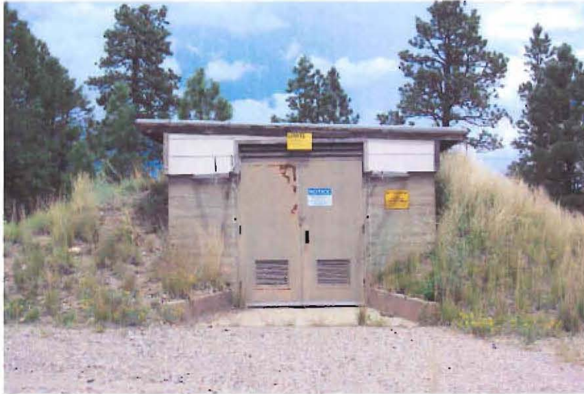
Figure 6. Typical TA-28 magazine building
