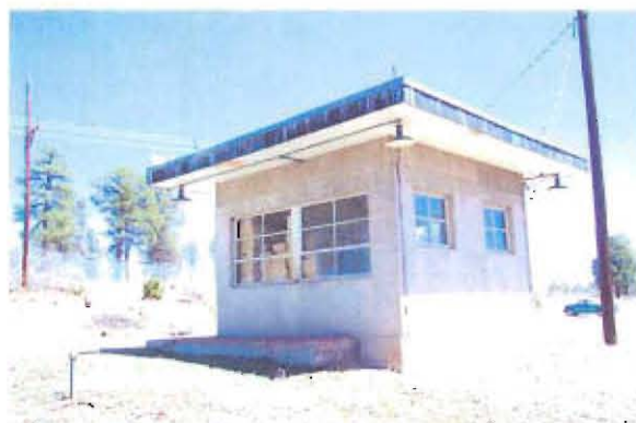
Oblique view of west and south sides
