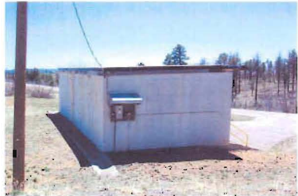
Oblique view of west and north sides
