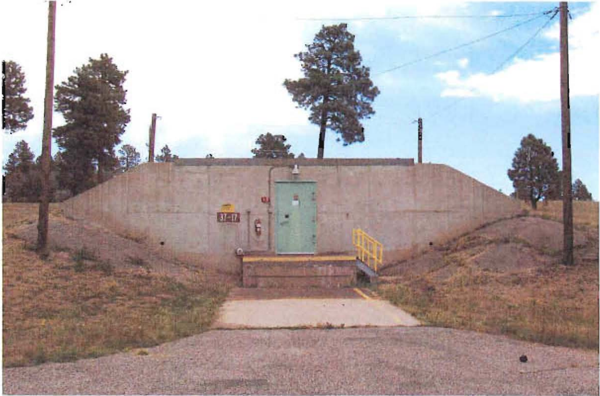
TA-37-17 Southwest Elevation
