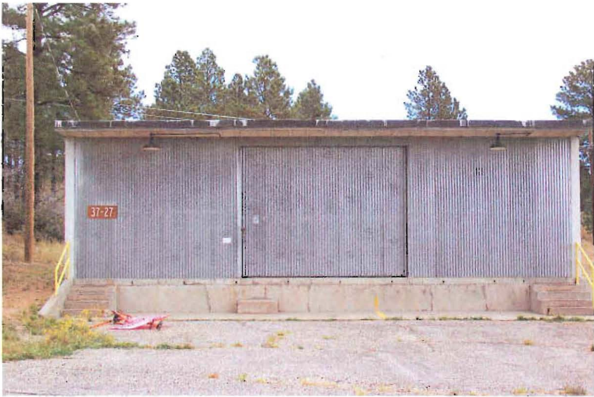
TA-37-27 Southwest Elevation
