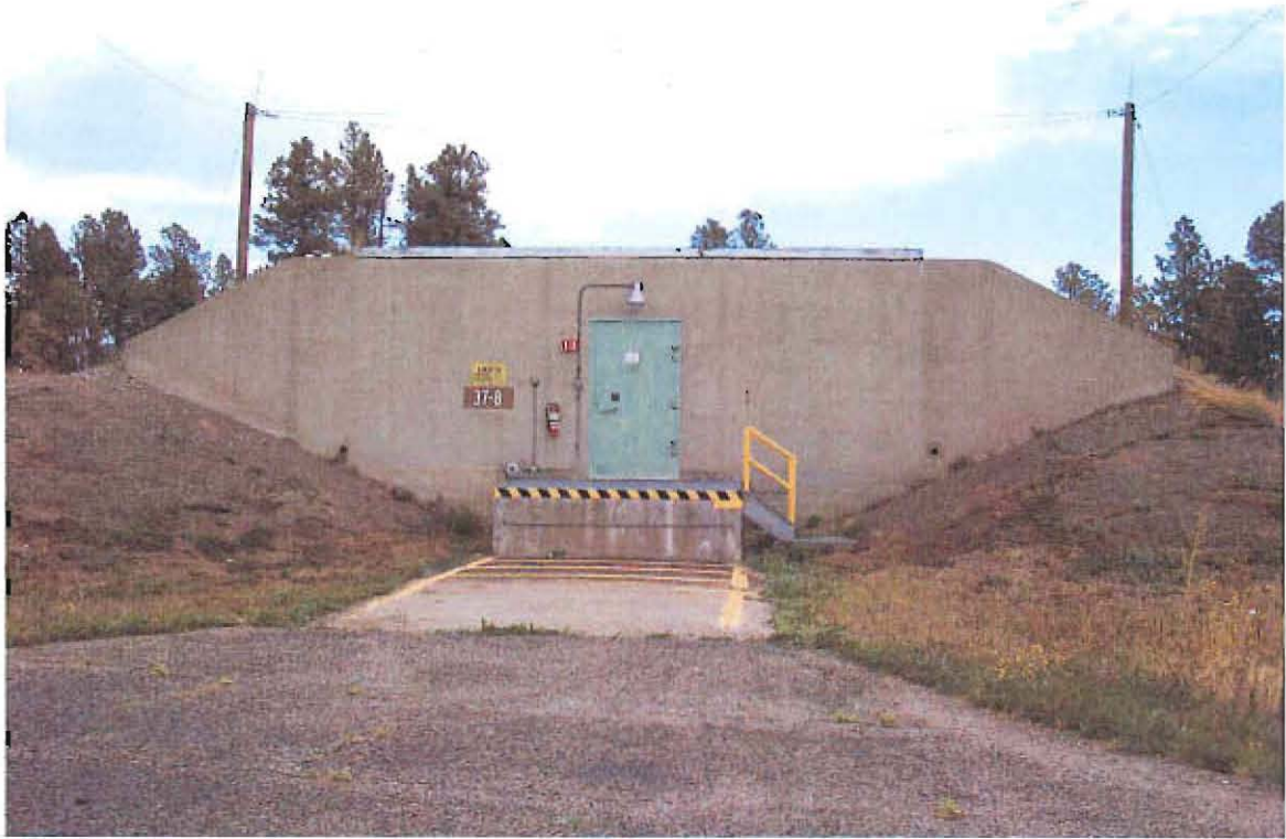
TA-37-8 South Southwest Elevation
