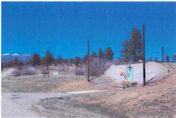
View to west with TA-37-17 in foreground and TA-37-27 in background
