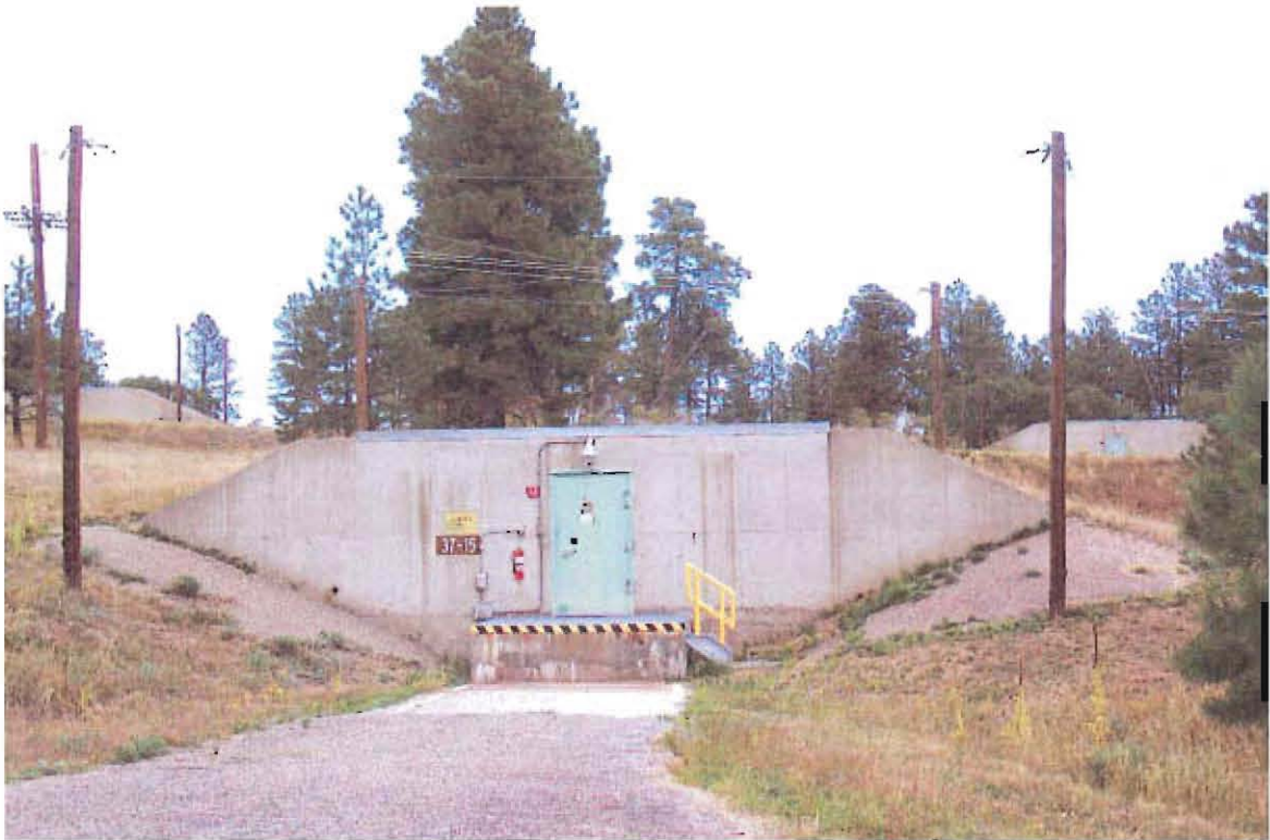
TA-37-15 Southwest Elevation
