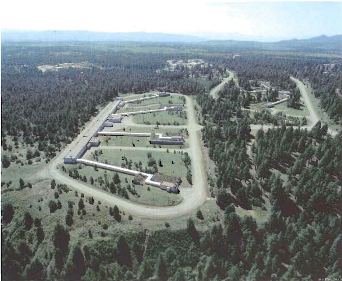
Figure 4. S-Site (TA-16), aerial view of high explosives processing “lines,” 1991
