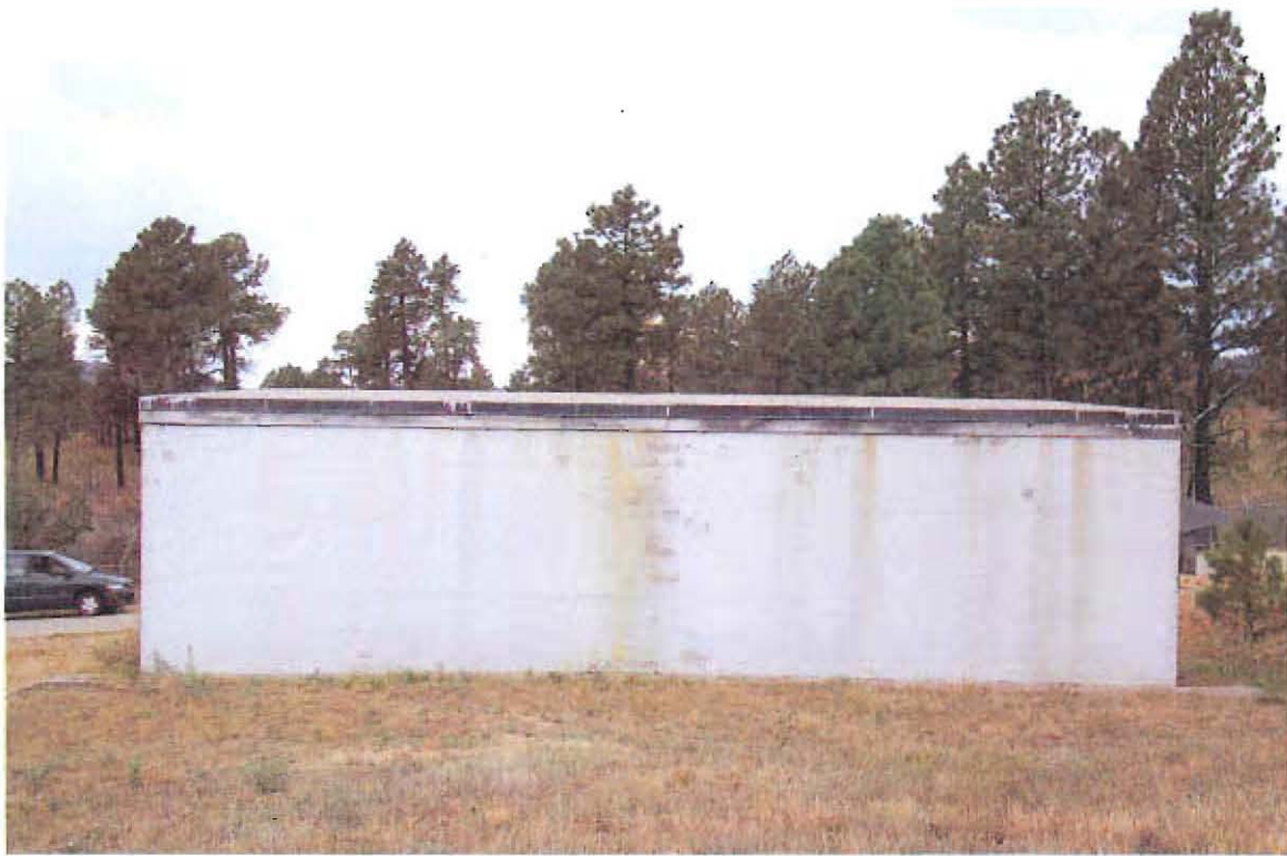
TA-37-27 Northeast Elevation
