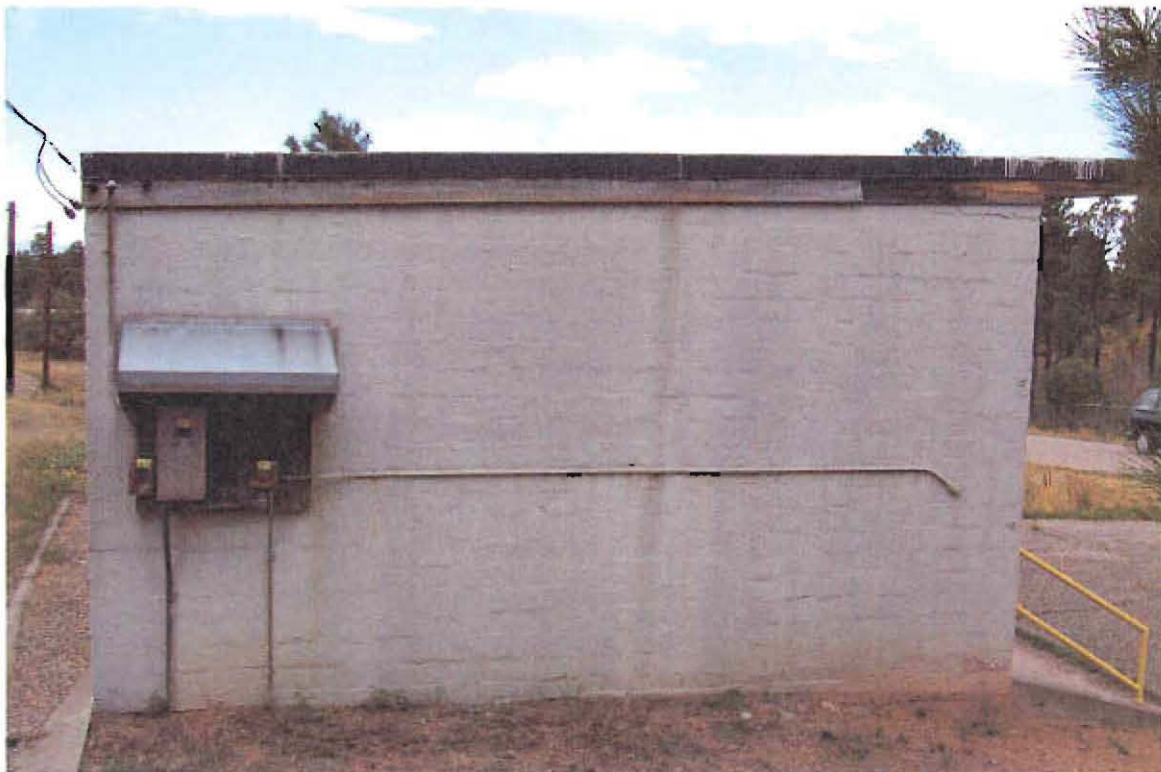
TA-37-27 Northwest Elevation
