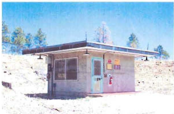
Oblique view of west and south sides
