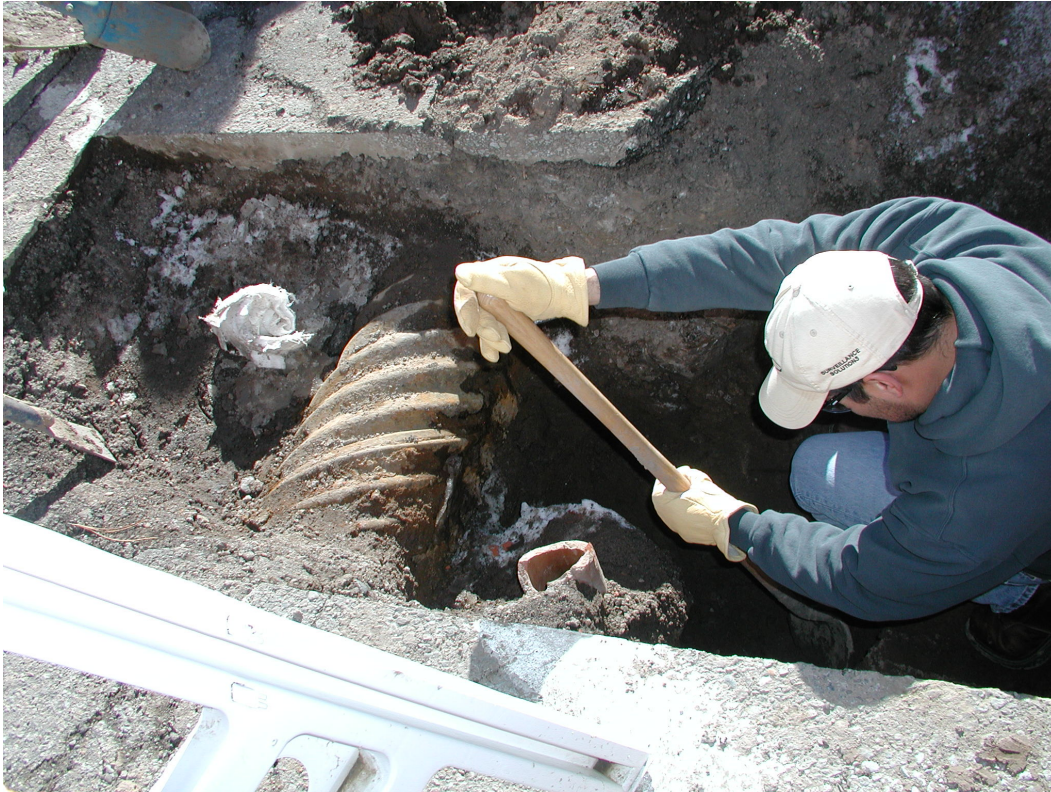
Figure B-18 Locating the roof drain at the third elbow
