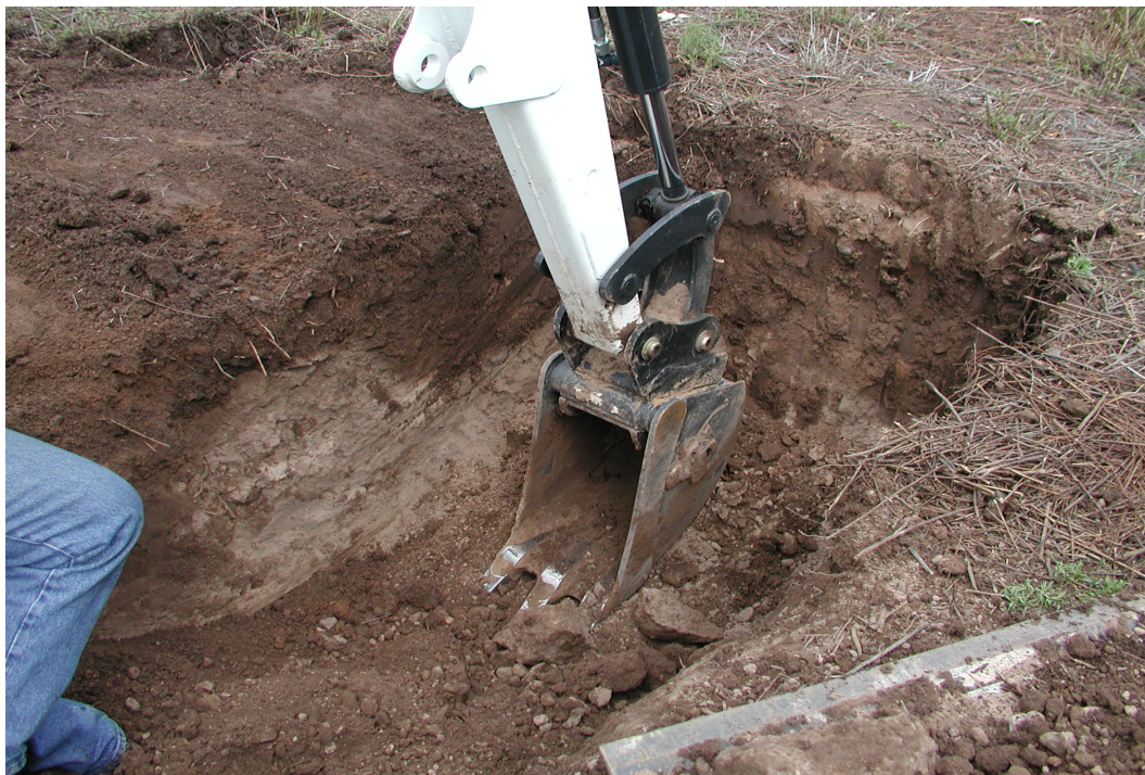
Figure B-2 Excavation activities at AOC 16-024(v)
