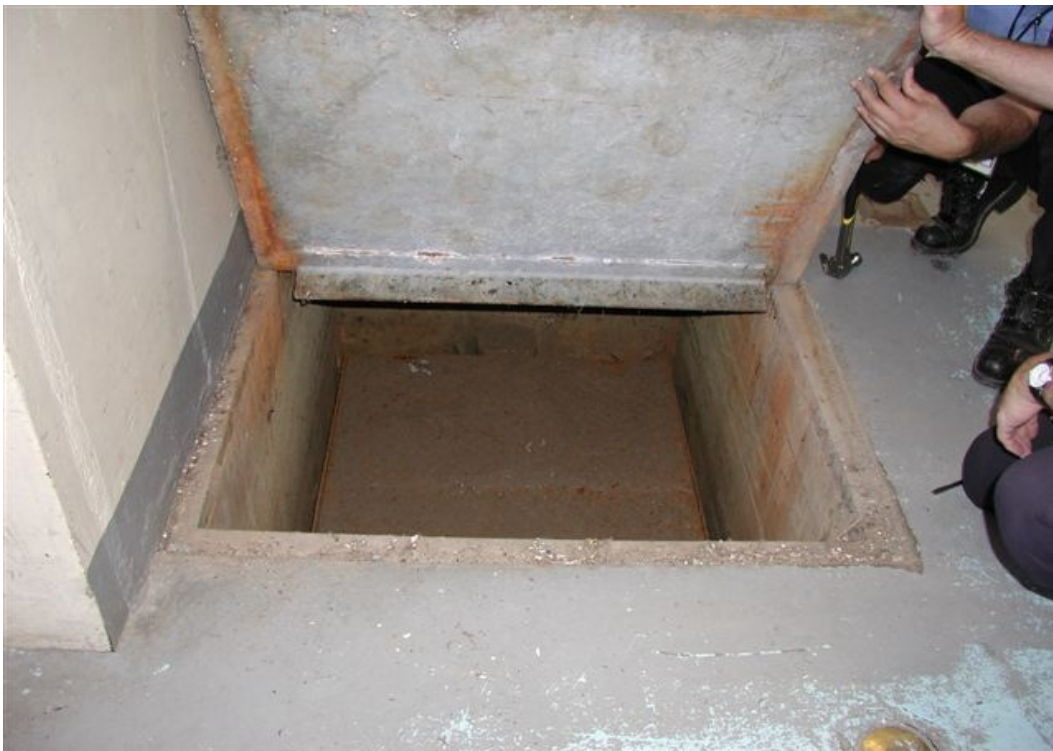
Figure B-6 The oil/water separator's interior shows little use.
