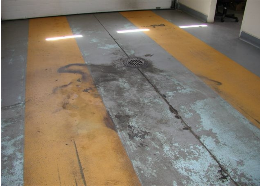
Figure B-5 Floor drain inside Fire Station #5
