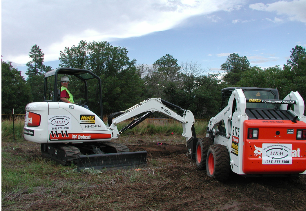
Figure B-1 Excavation activities at AOC 16-024(v)
