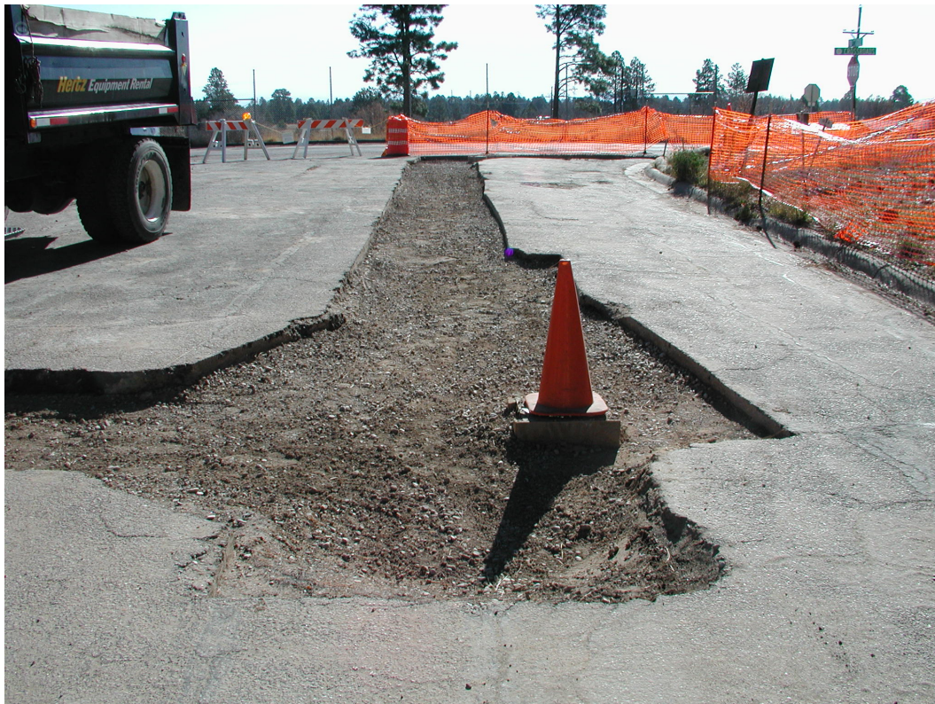
Figure B-20 The backfilled trench
