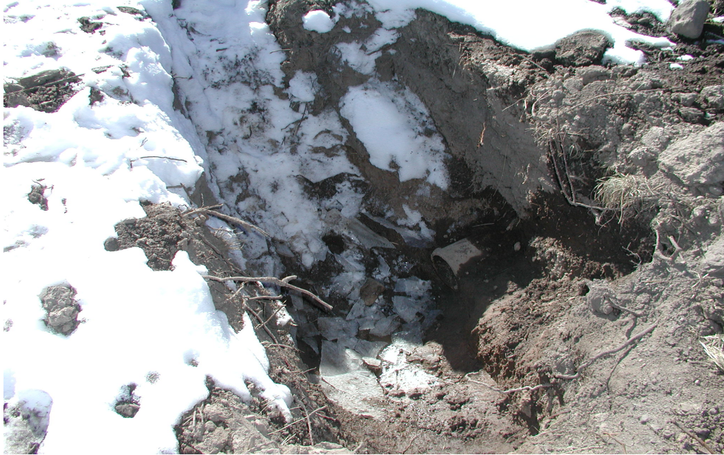
Figure B-19 Roof drain discharge location
