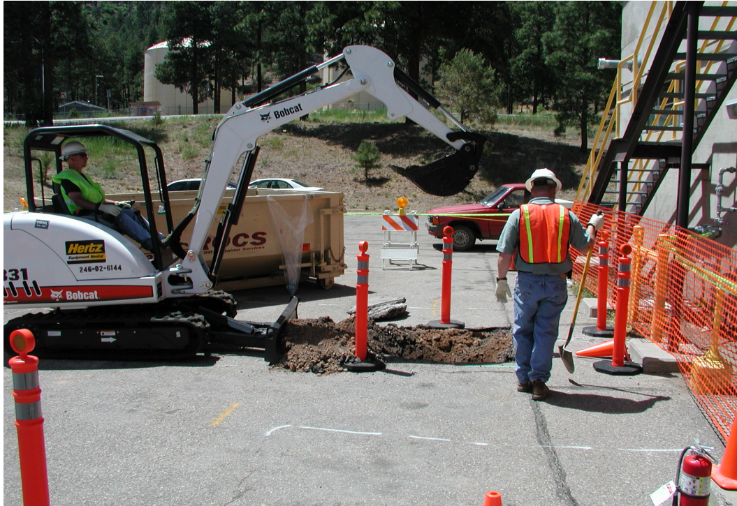
Figure B-7 Excavation activities at SWMU 16-026(r)
