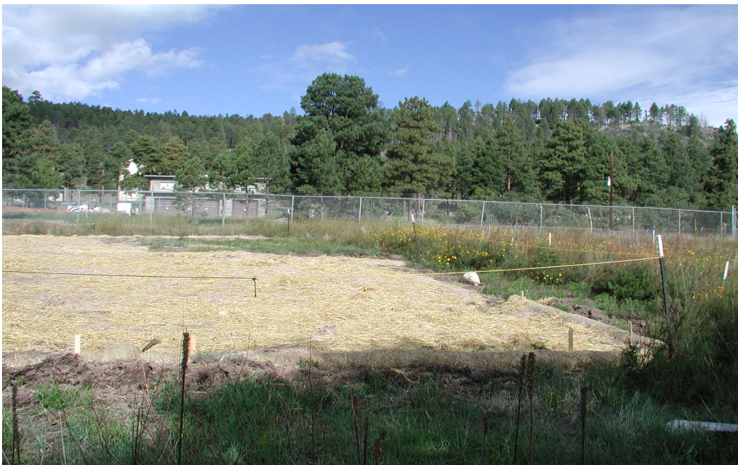
Figure B-4 AOC 16-024(v) reseeded and mulched
