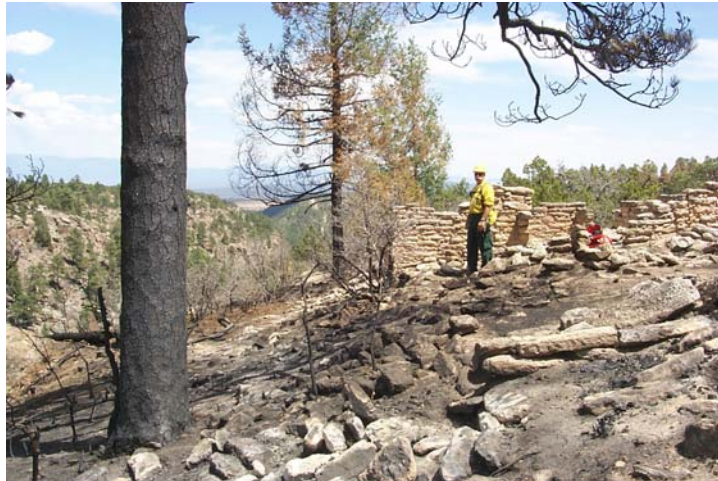
Figure 21. Site before Cerro Grande fire rehabilitation.
