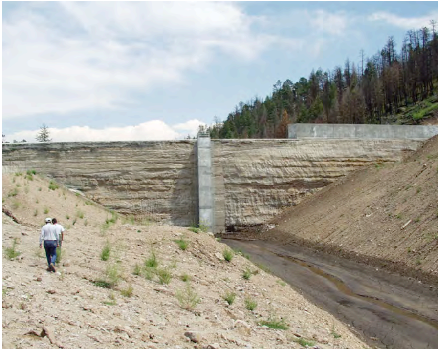
Figure 6-9. Flood retention structure, looking east.
