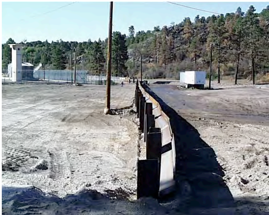
Figure 6-10. Steel diversion wall under construction.
