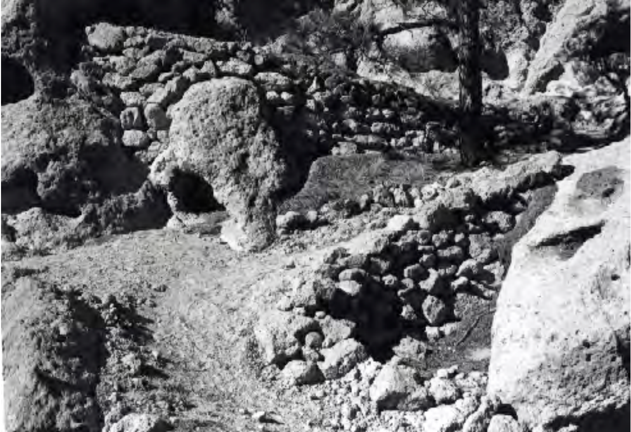
Ranch School students incorporated features of the terrain into their embankment work along the Camp Hamilton Trail.
