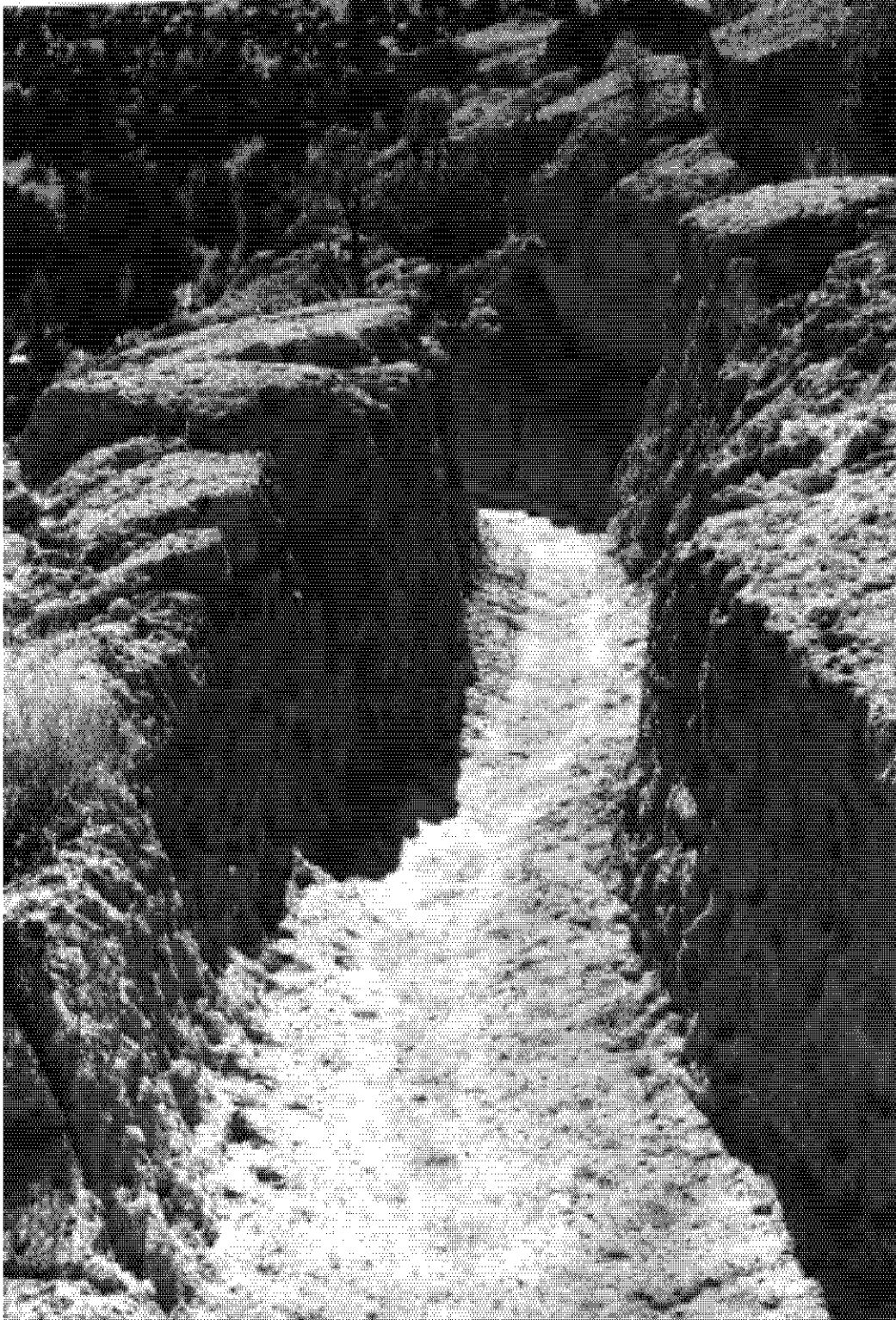
Ranch School students constructed this passage through solid rock on the Camp Hamilton Trail to accommodate horses. Note the uniform pick marks on the sides of the trench. The trench is over six feet deep.
