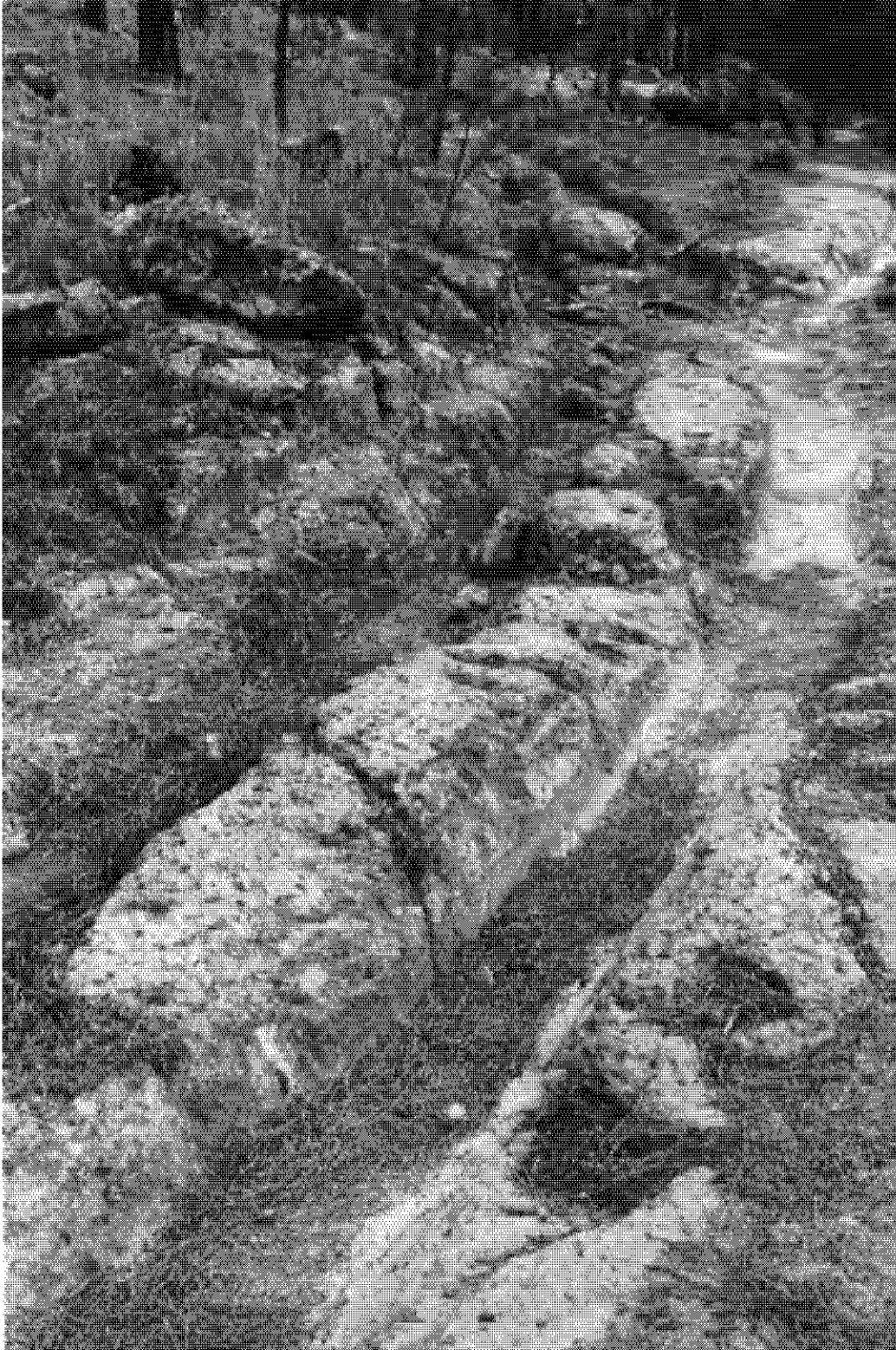
Characteristic step feature to the left of the ruts shows pick marks cut in the bedrock above, creating a low wall. The step is at the level of the original roadbed. This is the Grant Road leading from the head of Bayo Canyon to Guaje Pines Cemetery in Rendija Canyon.
