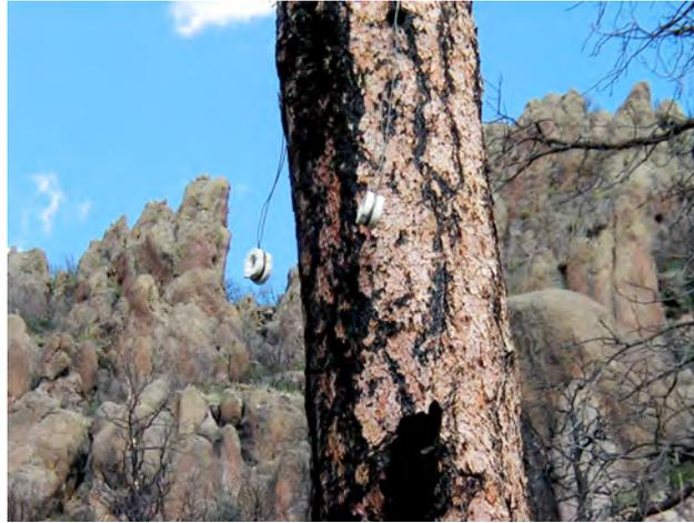
**Fig. 5-12. Thomas Flat-sided Oval. Two oval split knobs hang from a large decapitated ponderosa in Cabra Canyon, between the Pajarito Trail and Guaje Mountain. This insulator type was the most common type found on the corridor of the old Pajarito Line. (GPS waypoint PT3)**
