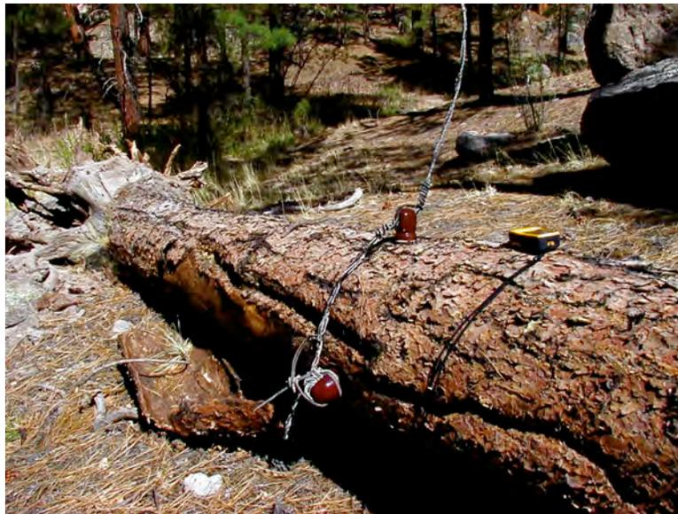
**Fig. 5-30. Two Post-style Insulators in Hidden Canyon.** These two brown post-style insulators are not forestry split knobs but are a single piece that was designed to screw directly into posts. The wire found on this segment of line is an insulated type of wire. (GPS waypoint H5)
