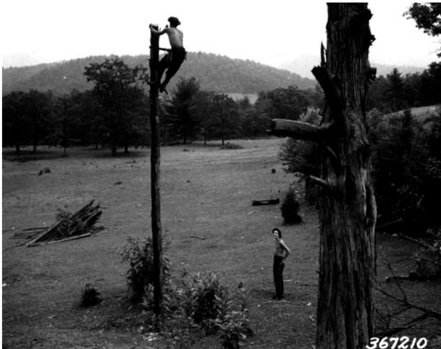
**Fig. 3-11. Pole Climbing Practice, 1938. Two CCC boys take turns practicing with climbing spurs used when hanging telephone line. (Photo: U.S. Forest Service)**
