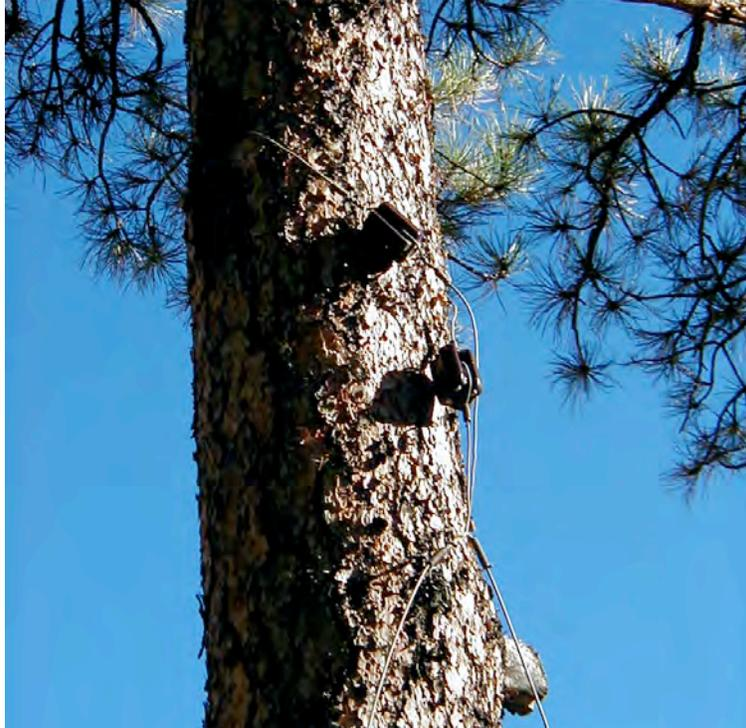
**Fig. 5-26. Double Strain Insulators.** This medium-sized ponderosa with two strain insulators is located near the bottom of Pueblo Canyon. The line jumped to the south rim of Pueblo Canyon where there was a second tree with a strain insulator to help support the line under stress. (GPS waypoint PC12)
