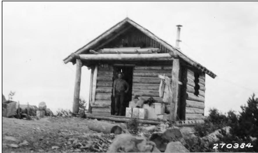
**Fig. 2-8. Saint Peter's Dome Cabin, 1932. The lookout cabin that was built soon after the peak of the Dome was blasted off in 1930. This was probably one of the last of the log cabin lookouts built. (Photo: U.S. Forest Service)**
