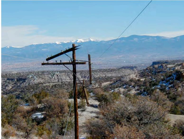
**Fig. 5-42. Broken Arms of the Mountain States. It once carried twelve wires on two cross arms to bring phone and telegraph service to Los Alamos.**
