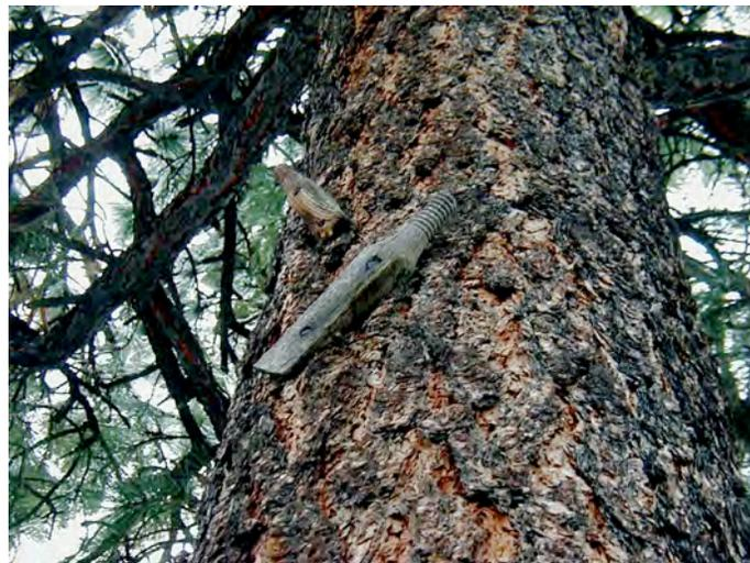
**Fig. 5-18. Double Brackets West of Ashley Pond.** Two wood brackets are nailed to the north side of a ponderosa in a parking lot west of Ashley Pond and north of Trinity Drive. This tie tree carried two east-west lines. (GPS waypoint BR1)
