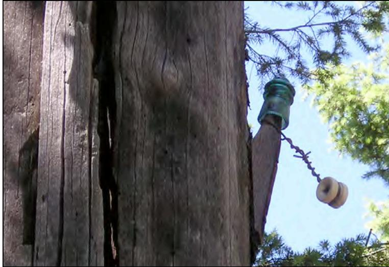
**Fig. 4-7. Hemingray with RT&SCO. This appears to be a transition between the Hemingray No. 9 and the small round split knob found on the spur line to Cerro Pelado Lookout—a line originally constructed in 1914. (GPS waypoint AP6)**
