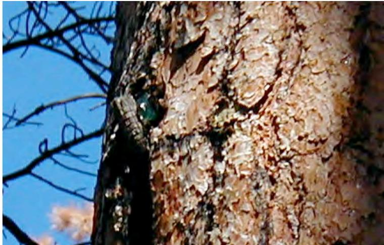
**Fig. 5-3. Bracket in Bark. The oldest insulators were sometimes completely enveloped by the bark of the tree. Just the threaded tip of the foot-long wood bracket and a piece of blue glass are all that's visible on a ponderosa in Rendija Canyon. (GPS waypoint R15)**
