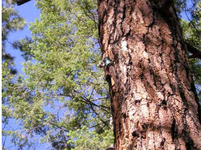
**Fig. 5-5. Hemingray and RT&SCO. Along the early branch line to Cerro Pelado the only insulator types found were the Hemingray and the early RT&SCO, a split knob. This particular alignment was abandoned by the early 1920s when the telephone line corridor was moved approximately three miles to the east. (GPS waypoint AP12)**
