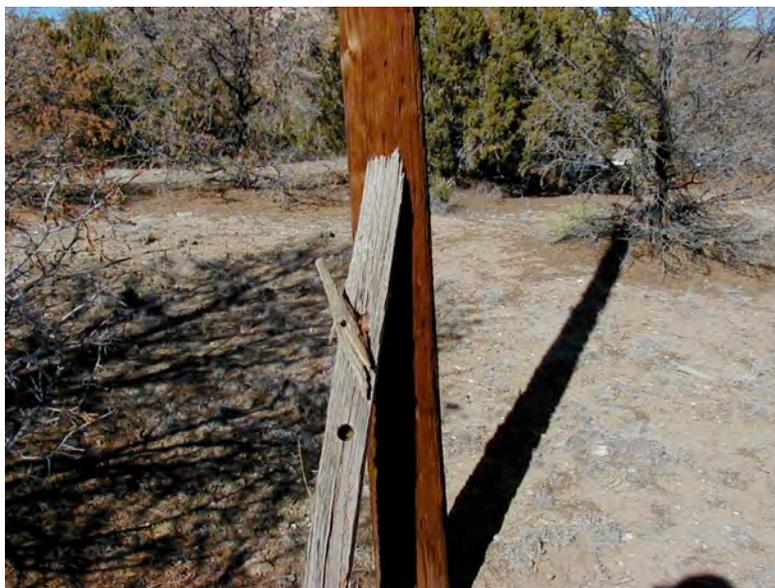
**Fig. 5-43. Two Generations of Telephone Poles. This desiccated cross arm and bracket leaning up against a creosoted pole suggests that an earlier line may have preceded the current standing poles. This earlier line may have been the original one built by the men from San Ildefonso and Santa Clara Pueblos. This pole is located in a north branch of Los Alamos Canyon.**
