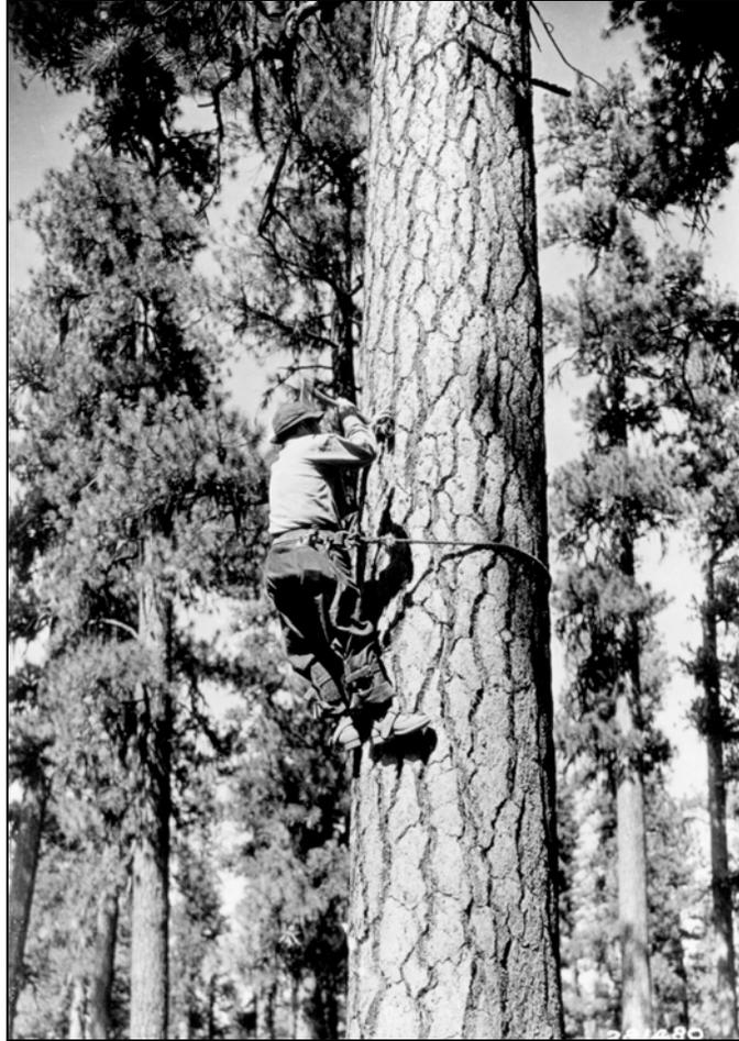
**Fig. 1-3. Hanging the Telephone Line, 1933. Men used climbing spurs to attach telephone insulators twenty feet up in tall, straight ponderosas. (Photo: Forest History Society at Duke University)**
