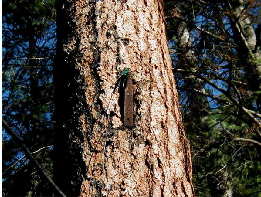
**Fig. 5-20. Wood Bracket on Reservoir Trail.** A large ponderosa on the edge of an old trail to Los Alamos reservoir has a single wood bracket on its south side. Telephone wire and a piece of blue glass are still caught between the bracket and tree. (GPS waypoint RR6).
