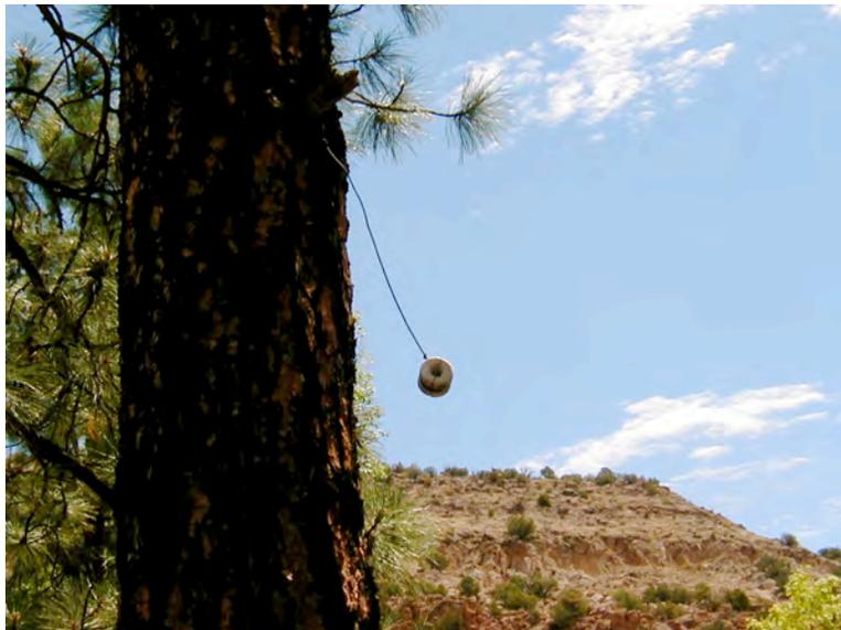
**Fig. 4-5. Split Forestry Knob. Porcelain insulator hangs at end of wire in Frijoles Canyon near Headquarters. The telephone wire would have passed through the center hole of the insulator. (GPS waypoint HQ4)**
