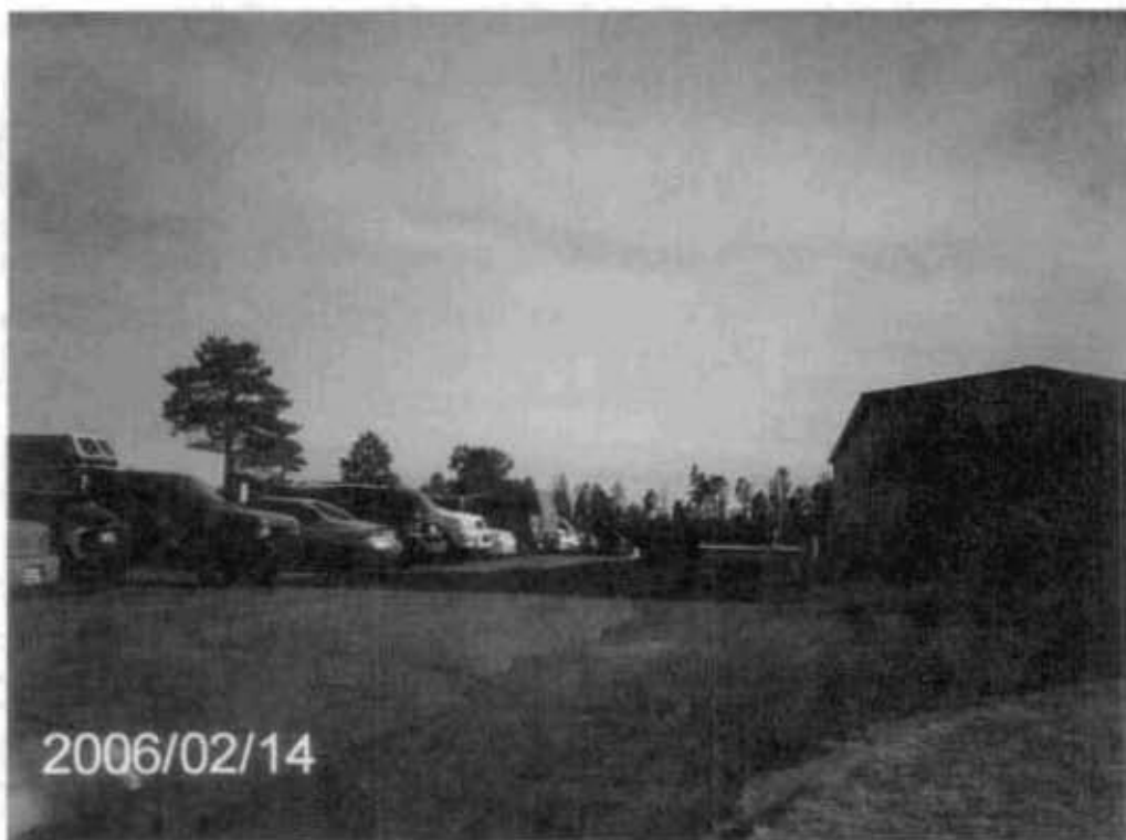
a) Looking south, line 170 runs beneath parking between LAMC (building on left) and HRL (building on right)
