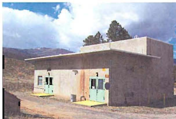
Photo 1d. View of south and east sides of TA-9-43
