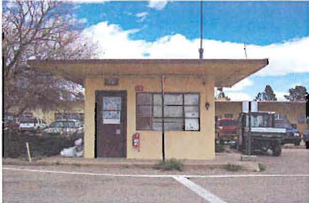
Photo 4a. View of south side of TA-15-46
