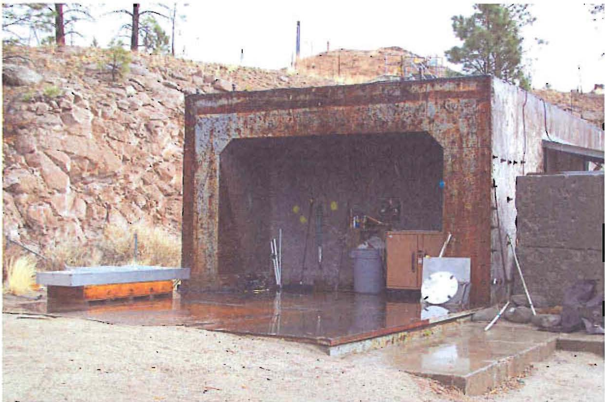
TA-40-4, southwest side
