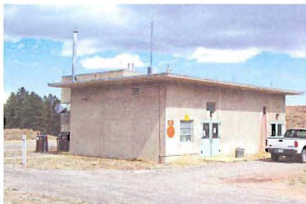
Photo 2. View of west and south sides of TA-9-34
