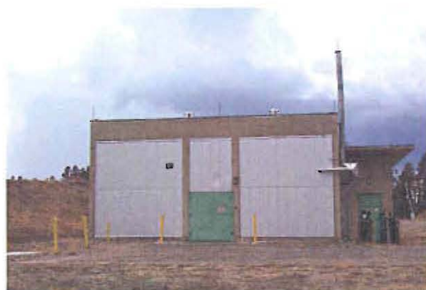
Photo 3. View of north side of TA-9-34
