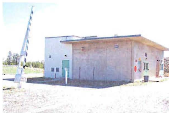
Photo 1b. Oblique view of west and south sides of TA-9-35. (Note addition at northwest corner.)
