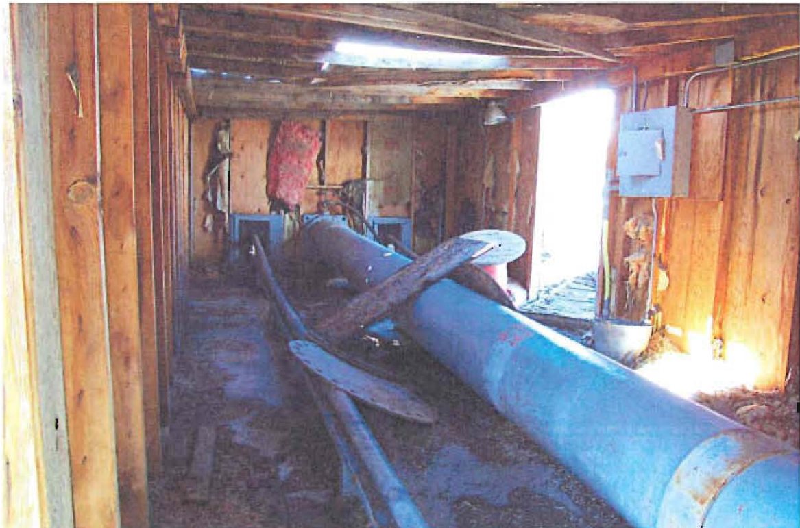
TA-49-121, Hydraulic Ram Enclosure, direction northwest (2005)
