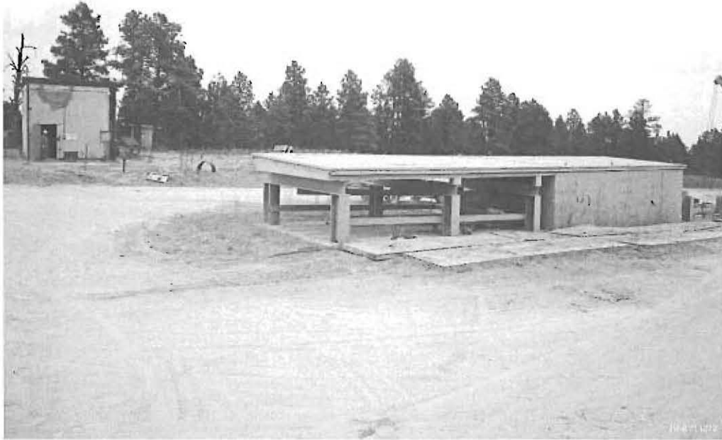
TA-49-121, west and south sides, TA-49-23 in left background (1971)
