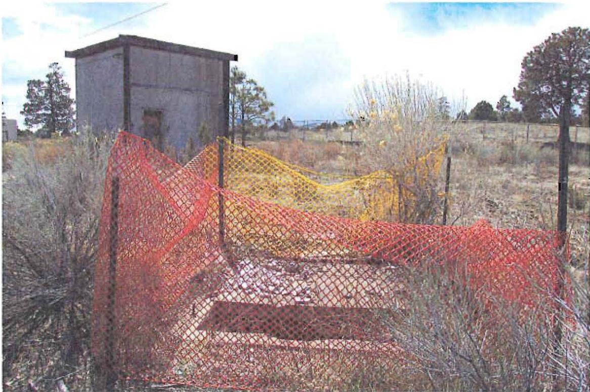
TA-49-21, Latrine remains. TA-49-23, in the background, direction southwest (2005)
