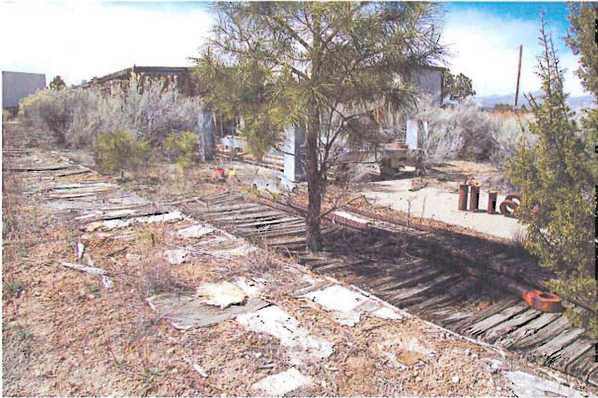
TA-49-121, pallets located south of building, direction northwest (2005)
