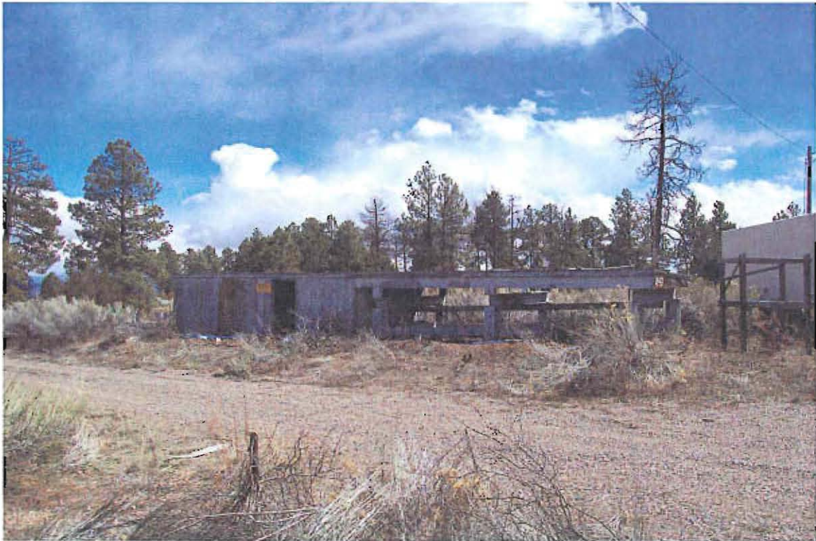
TA-49-121, Cable Test Facility, with Hydraulic Ram Enclosure, north side (2005)
