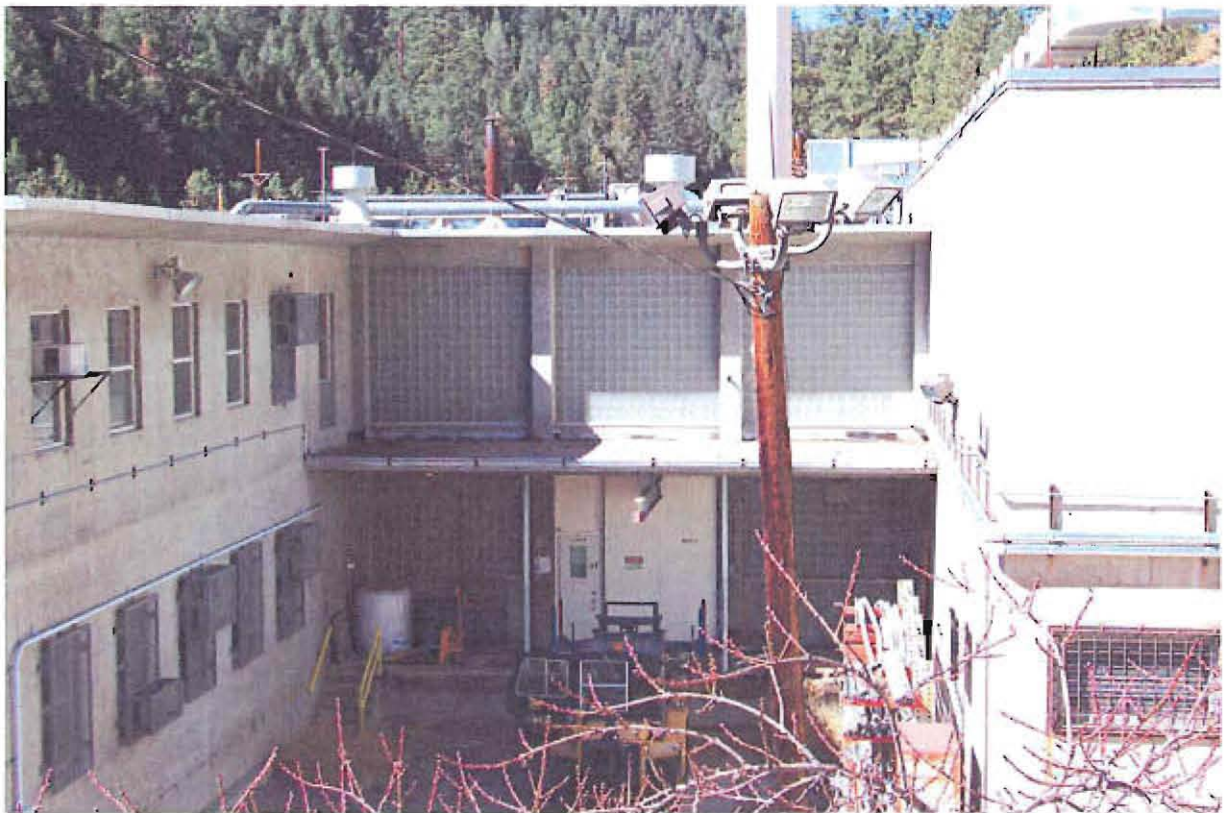
TA-41-4 Laboratory and Office Building, East Elevation
