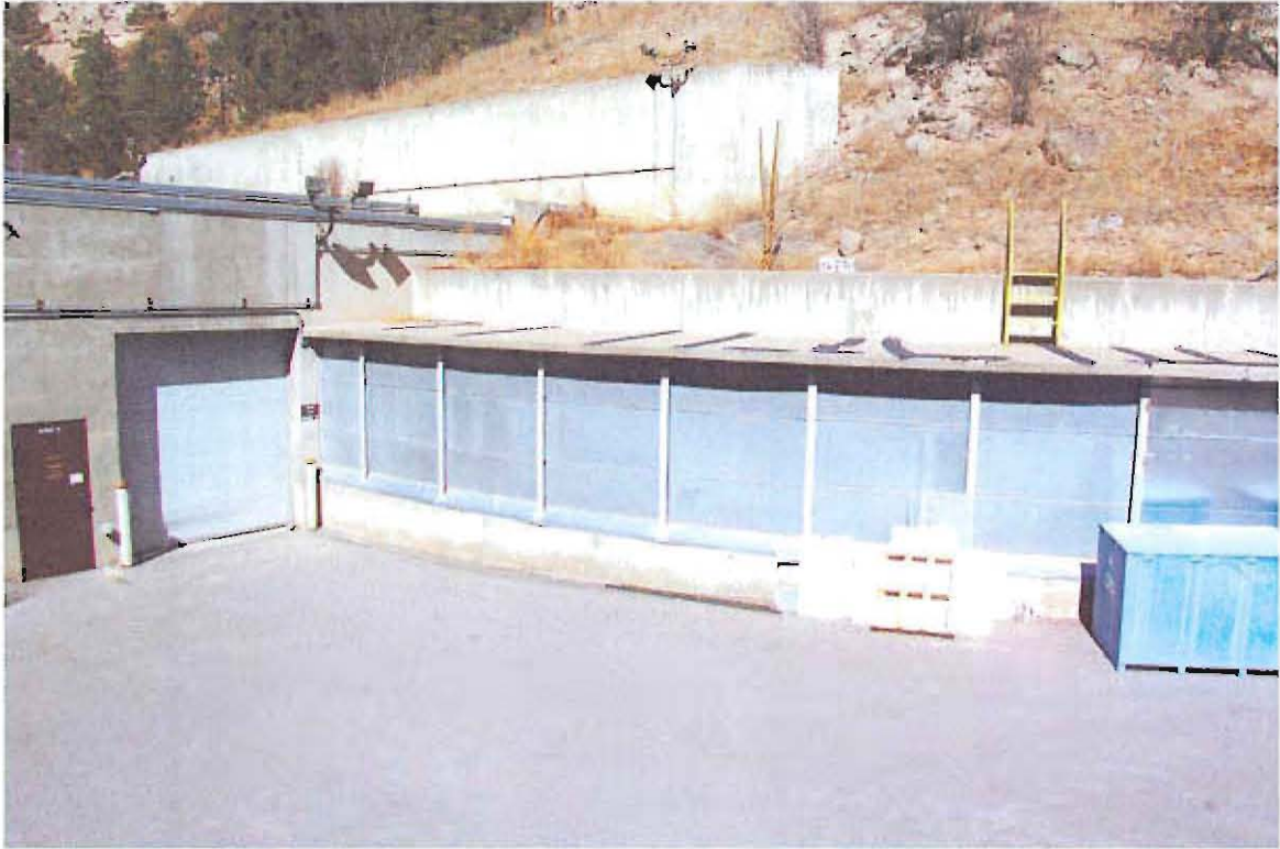
TA-41-6 Passageway, Connecting Building TA-41-4 (on left) to Building TA-41-1, South Elevation
