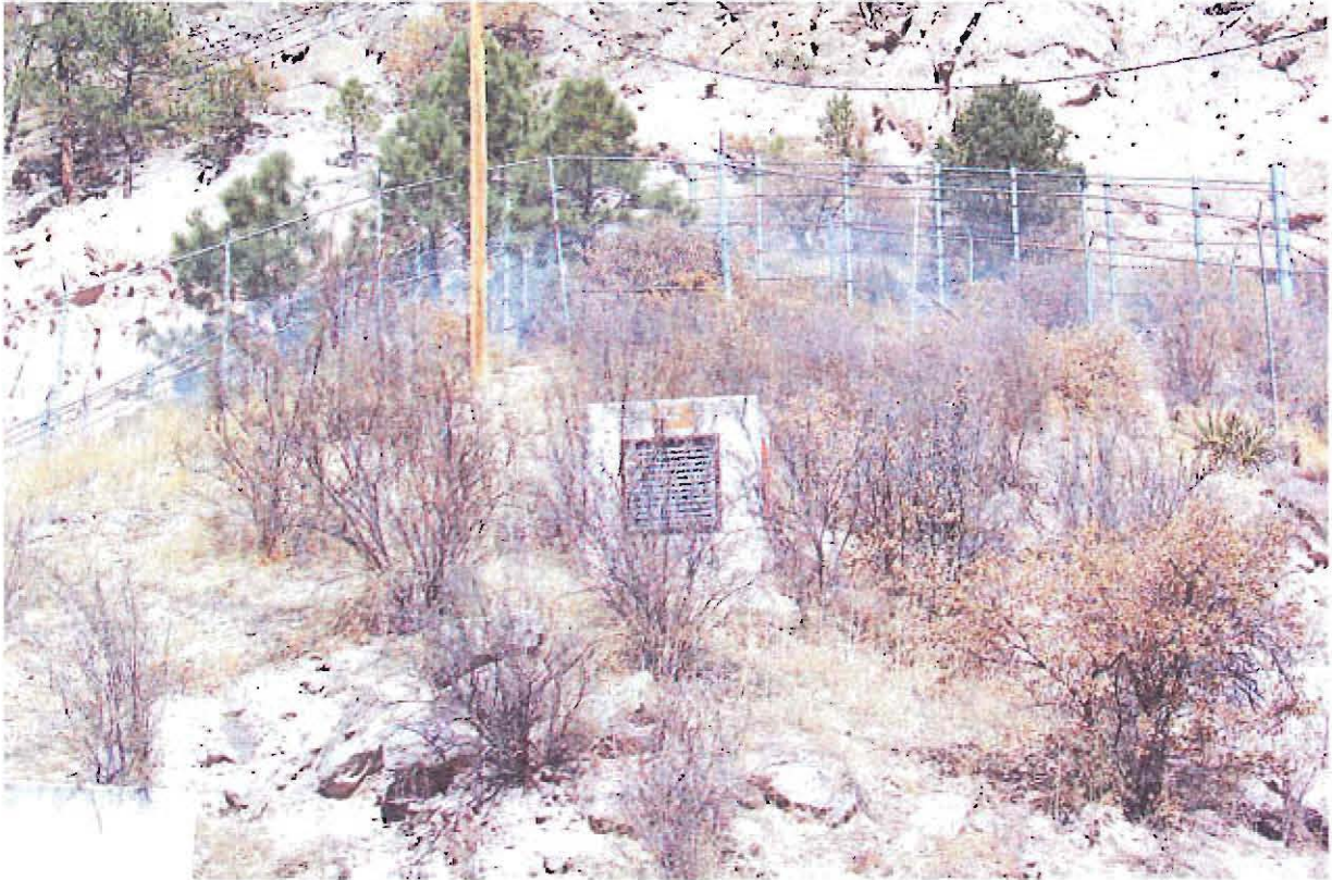
TA-41-3 Blower House Air Intake, South Elevation
