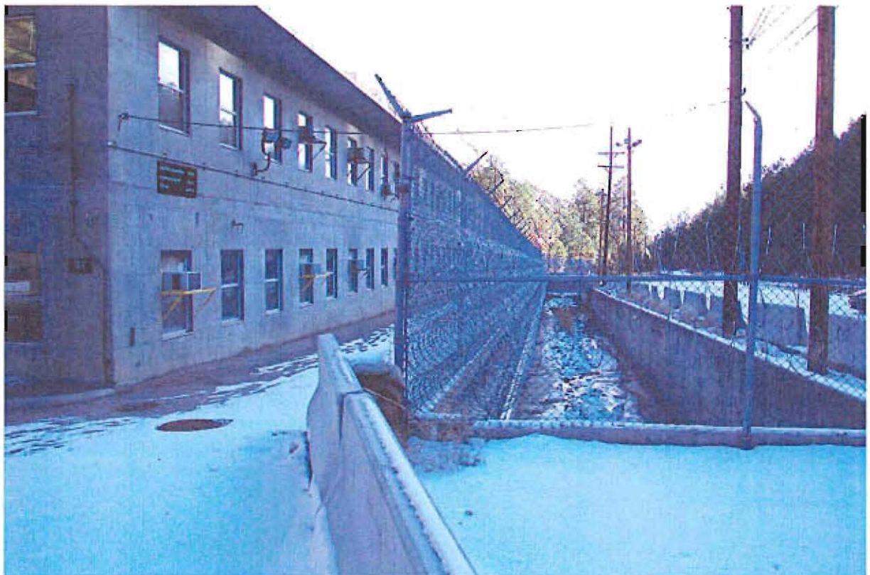
TA-41-4 Laboratory and Office Building, South Elevation
