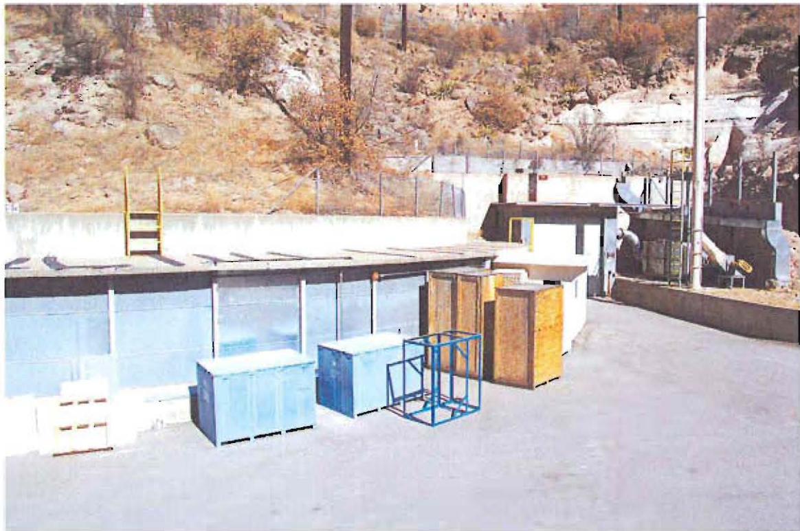
TA-41-6 Passageway, Connecting Building TA-41-1 (on right) to building TA-41-4, South Elevation
